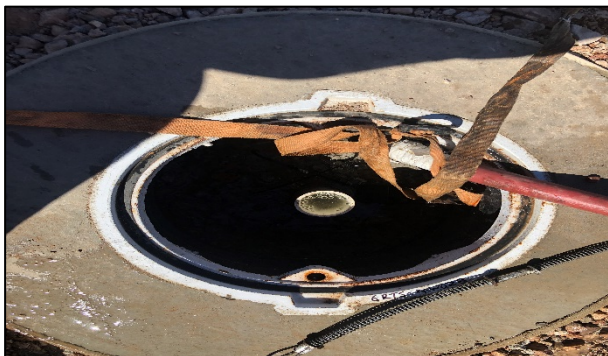
7. September 19, 2018 Post Injection and Demobilization Site Conditions
