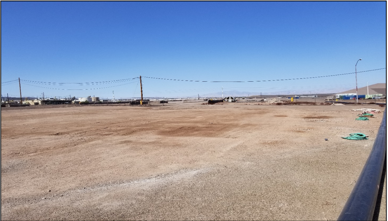
Facing West: Former UFIW-05, UFIW-06, UFIW-07 and UFIW-08 locations after well abandonment.
