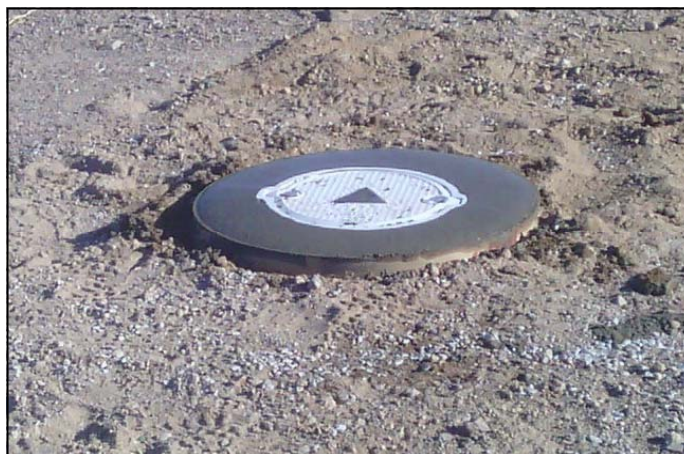
Typical Monitoring Well Surface Completion
