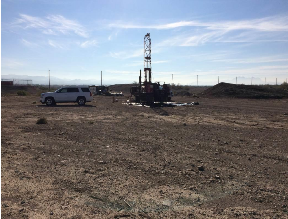
Photo 3. Borehole BH-L09-1, View looking southeast.
