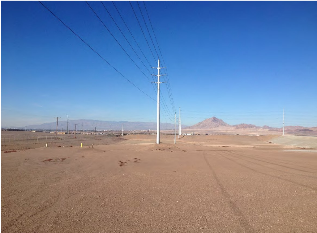
Photo 11: ECA D1 facing Northwest
