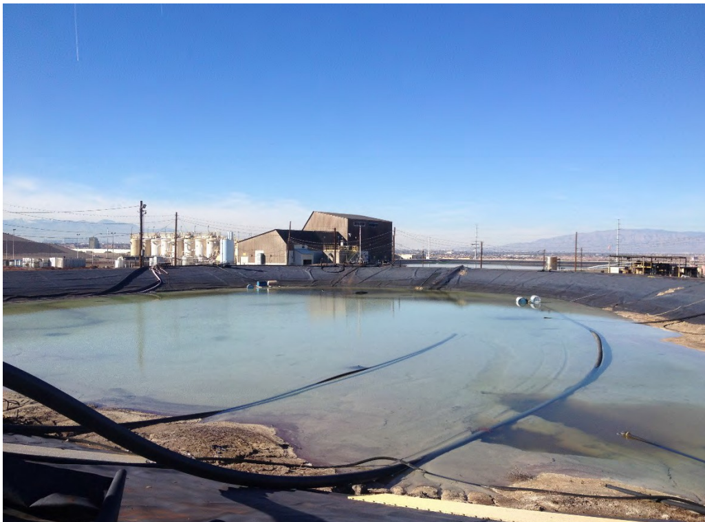
Photo 10: ECA D8 facing Northwest
