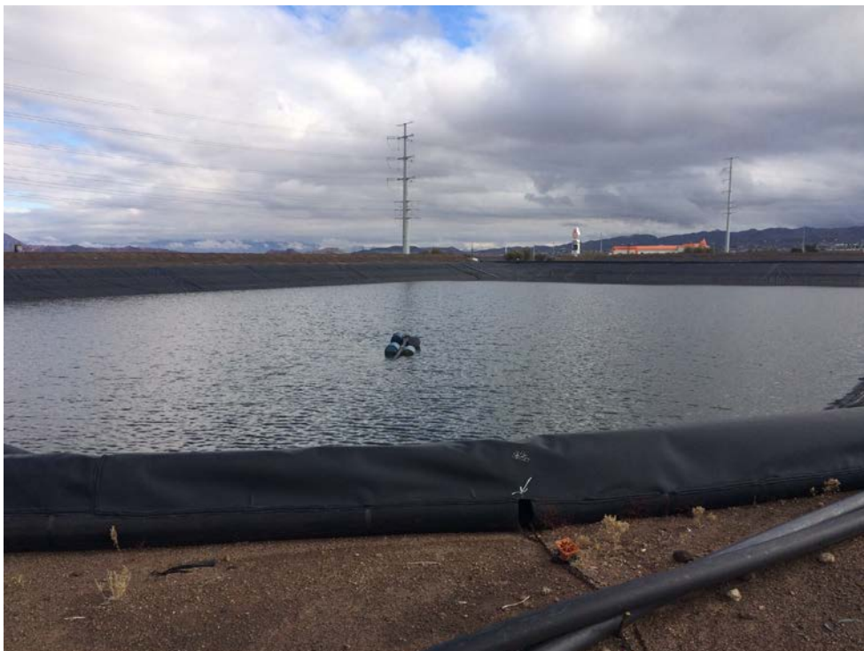
Photo 10: WC-East Pond Facing East
