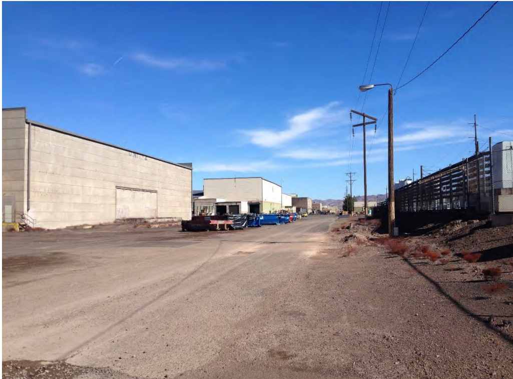
Photo 1: Excavation Control Area (ECA) from Unit 1 in Zone B facing Northeast
