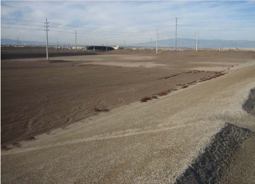
Photo 1: Former Impoundment Soil Removal Area Directly West of GW-11
