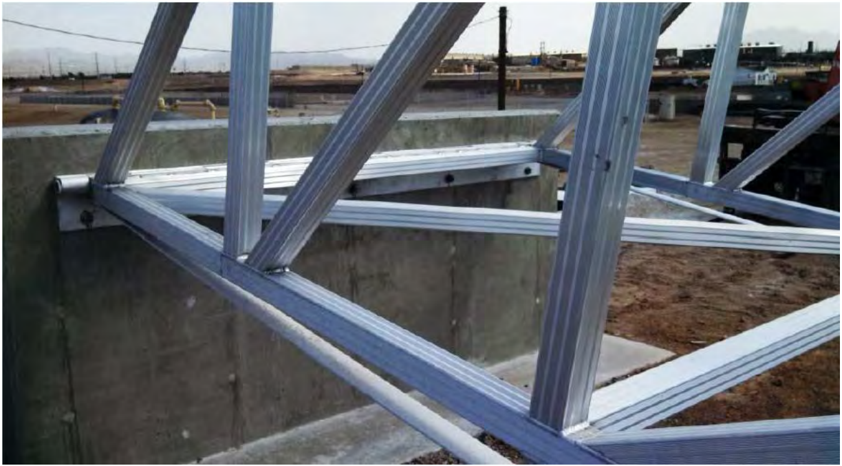
Photo 5: Facing southeast. View of the completed bridge footing structure.
