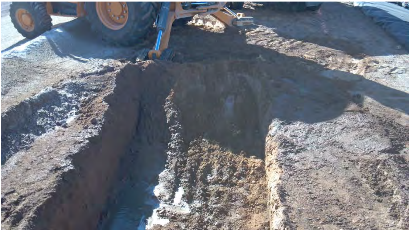
Photo 4: Facing south. View of the excavation in progress.
