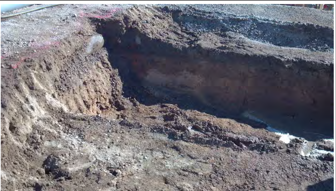
Photo 3: Facing northeast. View of the excavation in progress.
