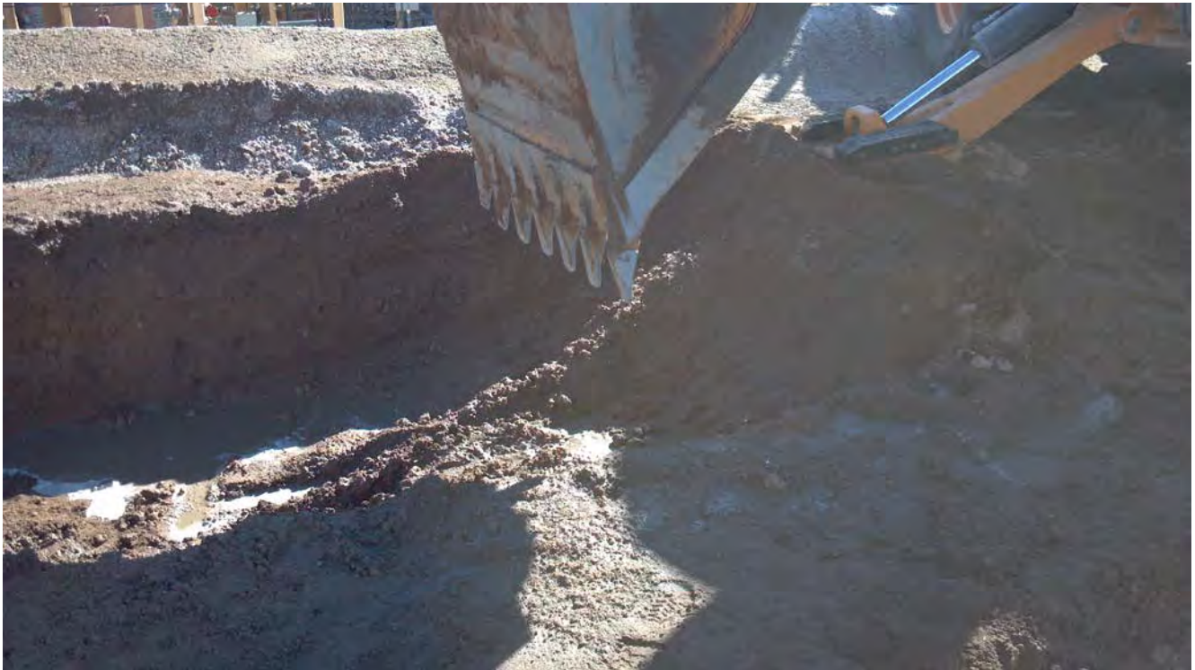
Photo 2: Facing east. View of the excavation in progress.
