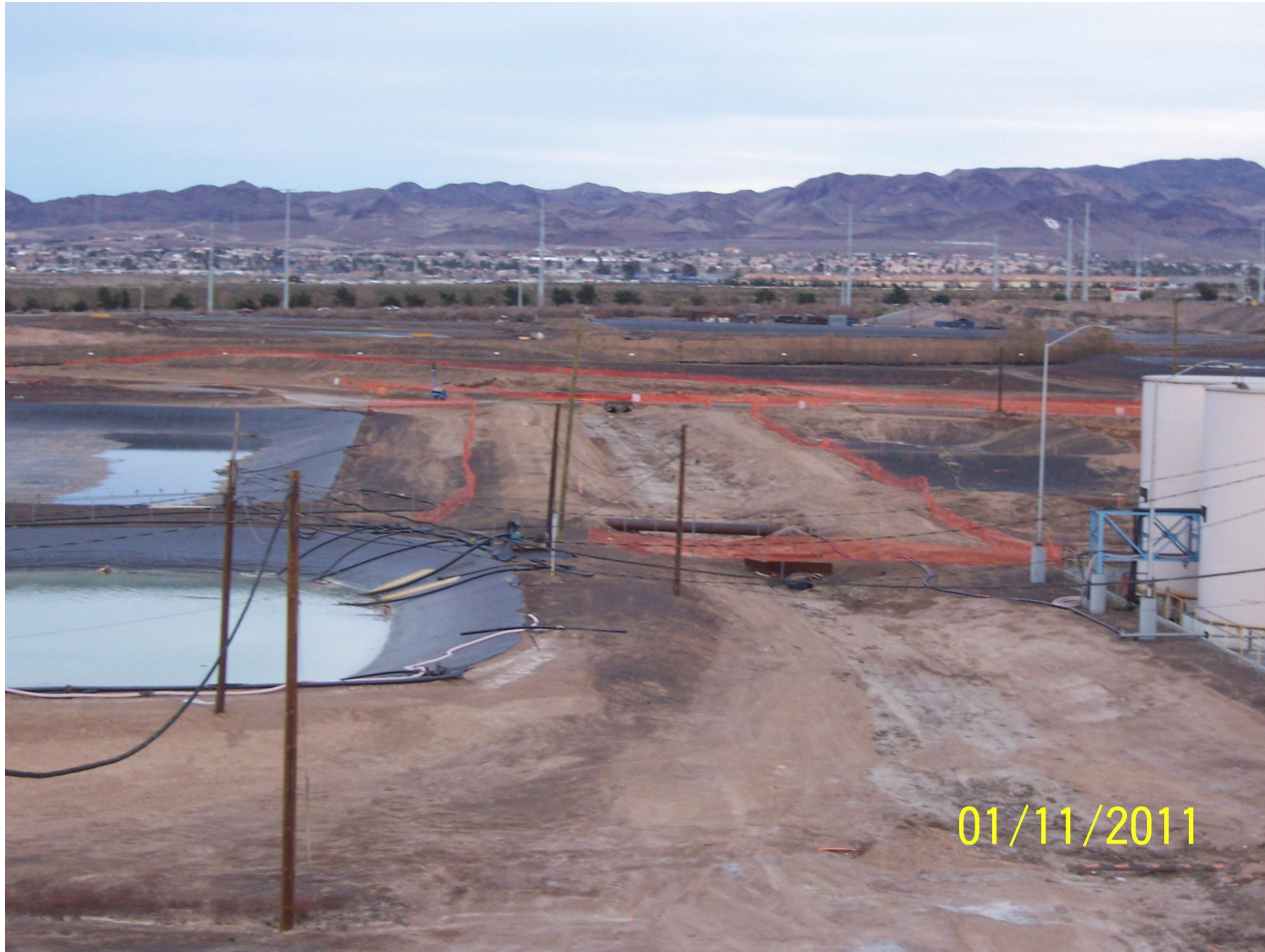
RZ-E-8B, 9, 10, 11, 12 Before Polygon Excavation with Orange Fence
