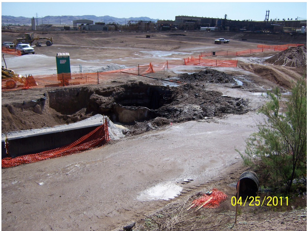
RZ-E-14A Polygon Excavation with Orange Fence
