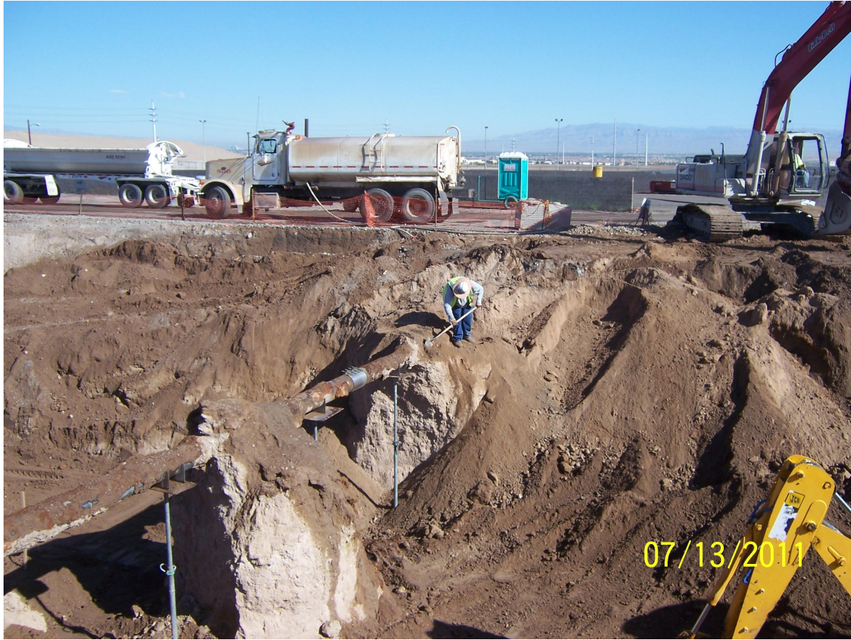
RZ-E-4 Polygon Excavation Around Waterline
