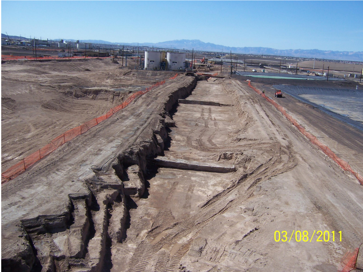
RZ-E-12 to 8B ACM Excavation with Orange Fence
