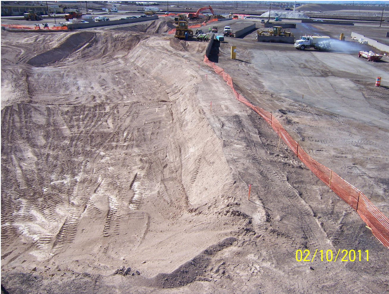
RZ-E- 6 & 4 Polygon Excavation The Line between RZ-C & RZ-E was Carefully Cut
