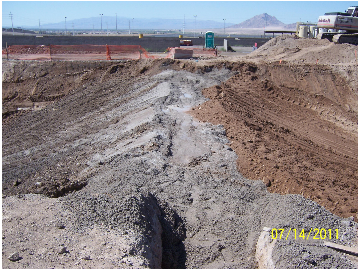
RZ-E-4 Polygon Excavation Around Waterline as Backfill is Placed
