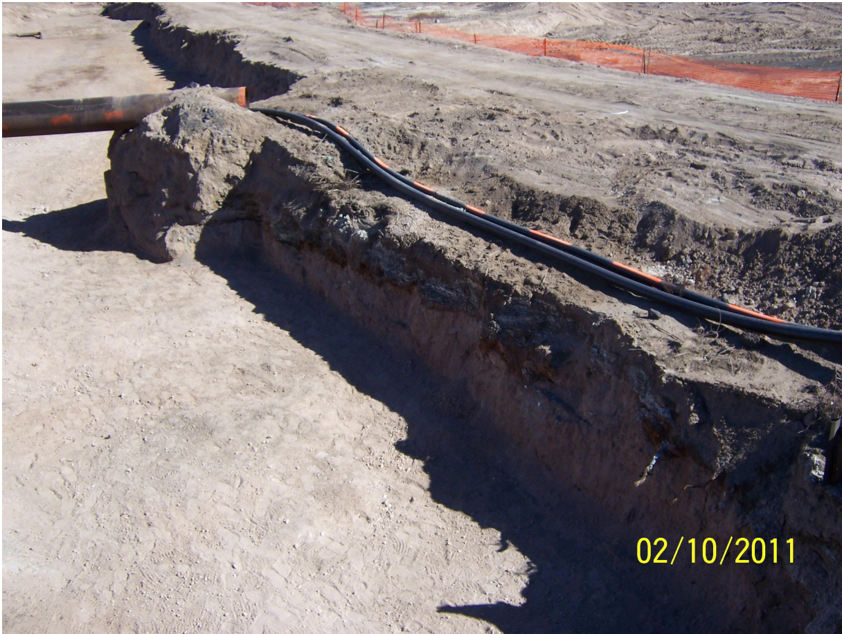
RZ-E-8B ACM Excavation with Orange Fence with additional Visually Impacted Soil
