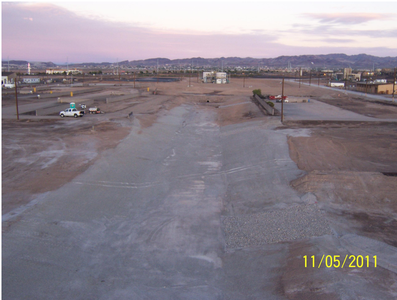
RZ-E-2, 3, 3A, 4 Polygon Backfill and Finish Grading with Erosion Control Down Drains
