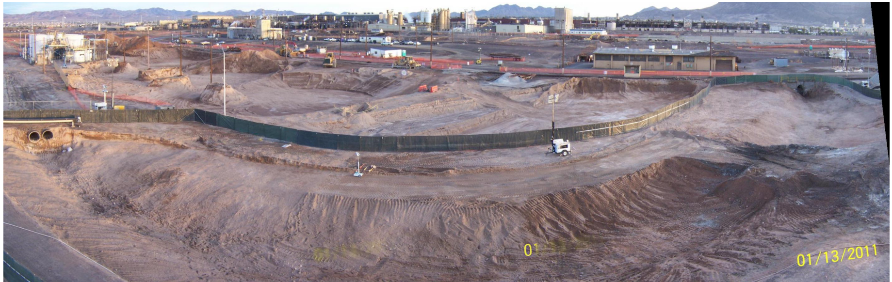
RZ-E- 4 to 8 ACM Excavation with Orange Fence
