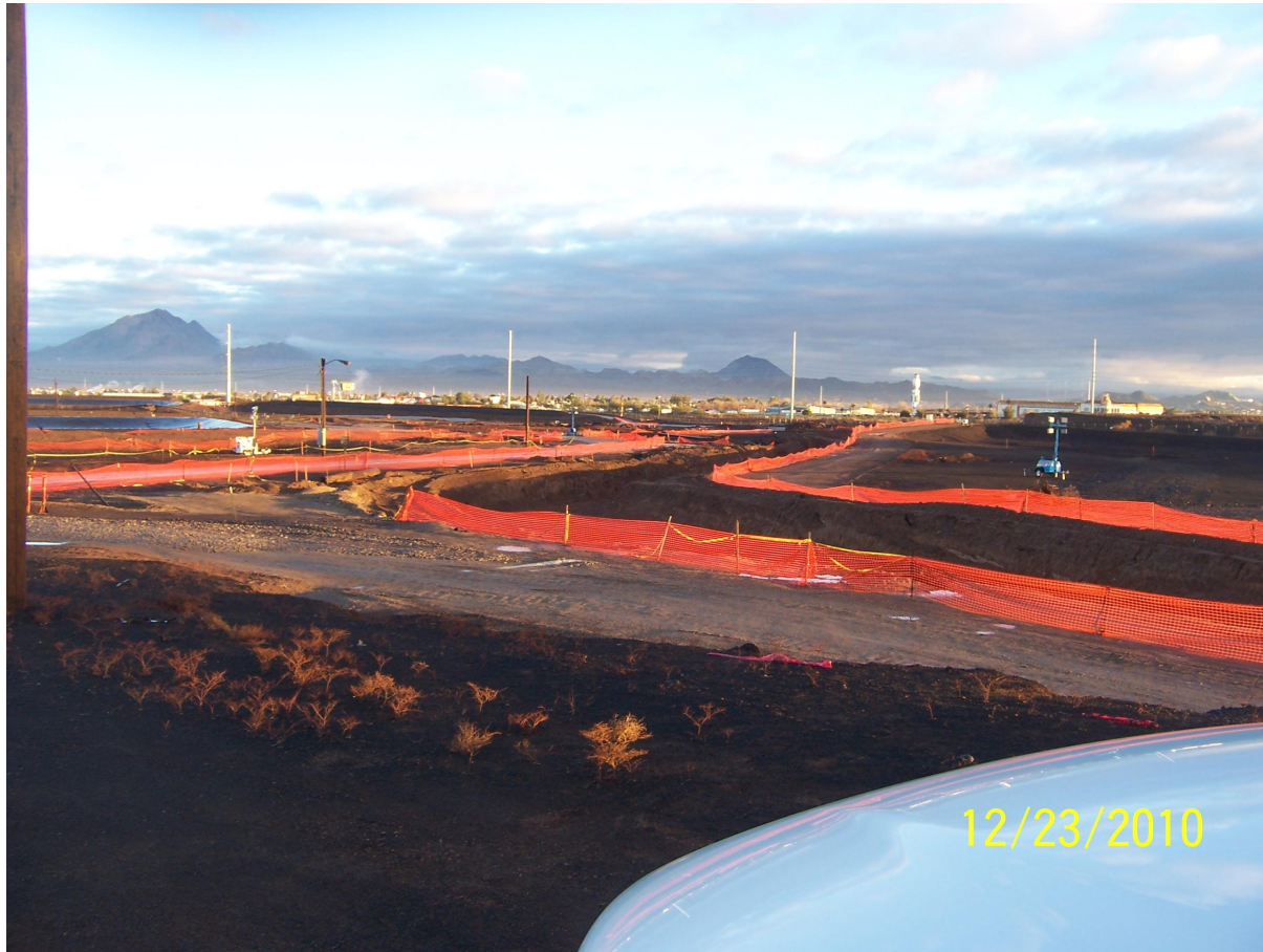
RZ-E-14, 14A, 14B Polygon Excavation with Orange Fence
