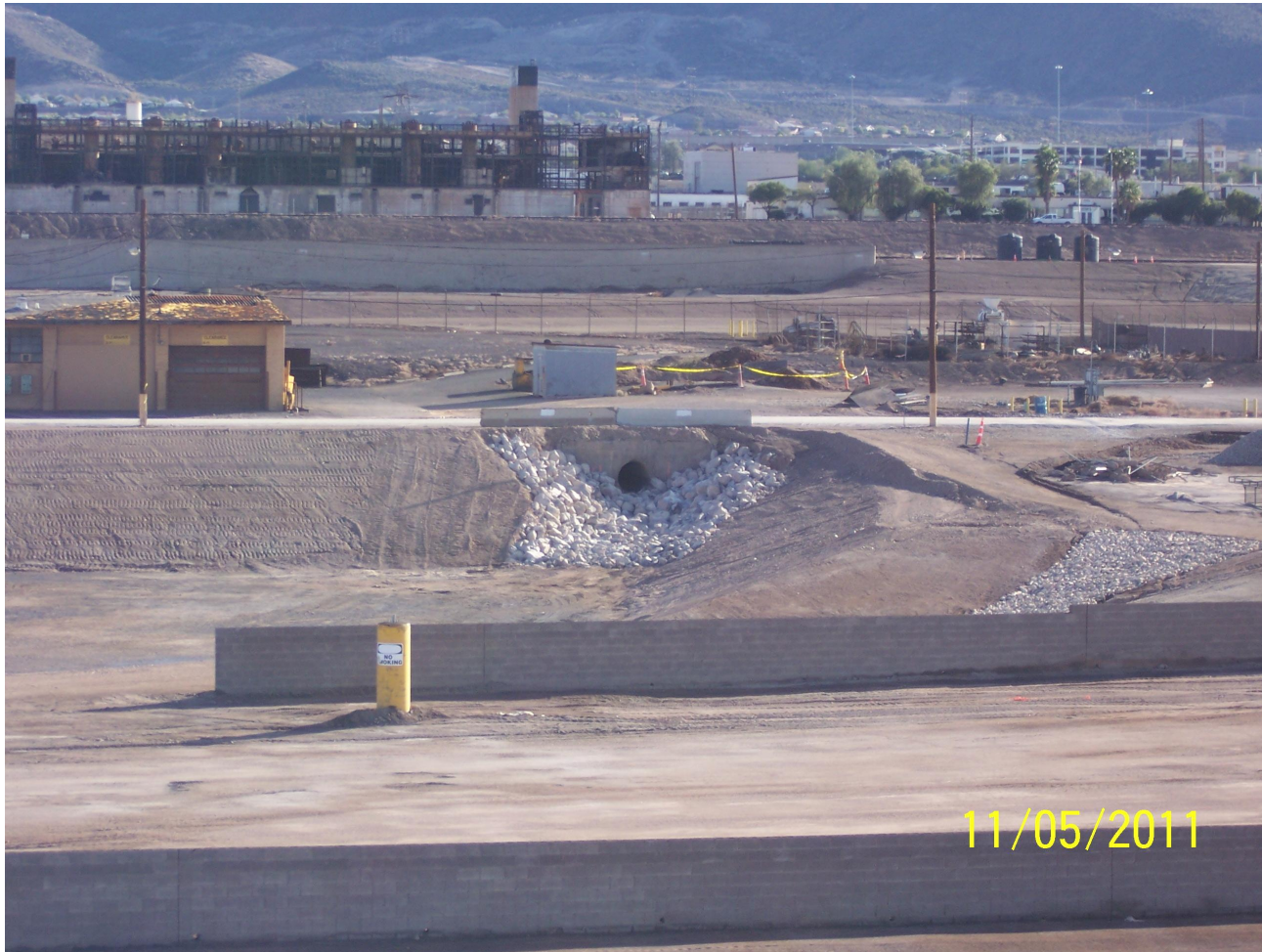
North RZ-C- Central Basin Area Storm Water 60" Plant Drain Pipe with Rip Rap
