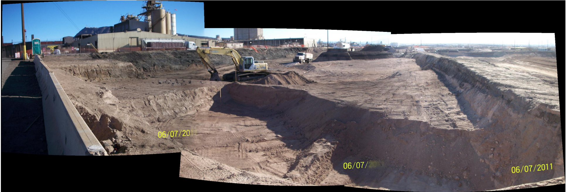
South RZ-C- 23 & 27 Polygon Excavation
