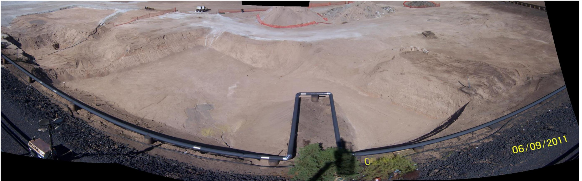
South RZ-C- 44 Polygon Excavation
