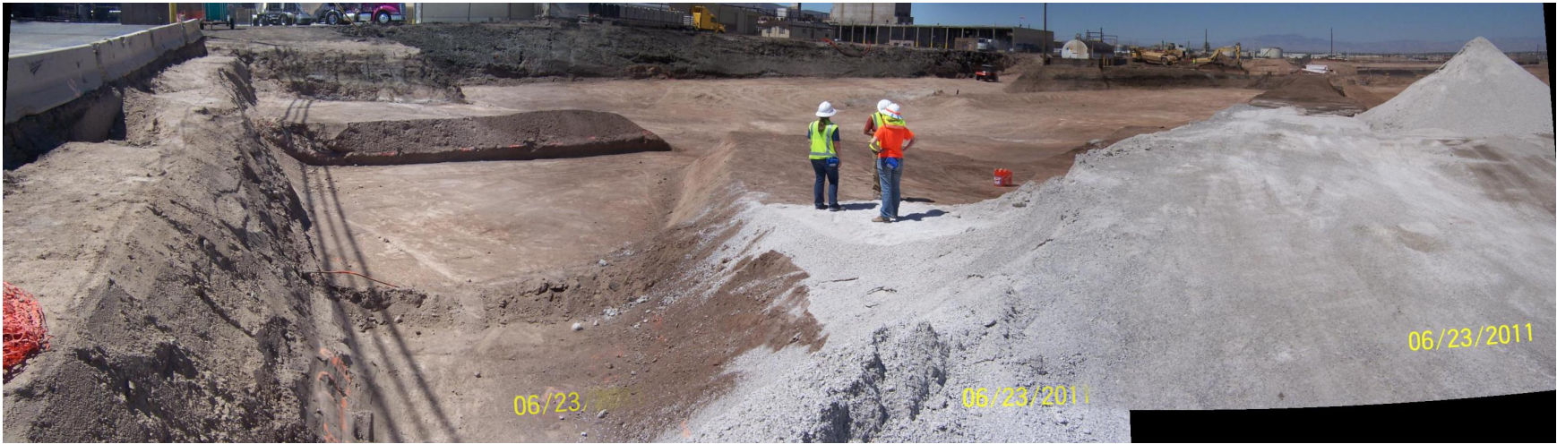
South RZ-C- 27 Polygon Excavation
