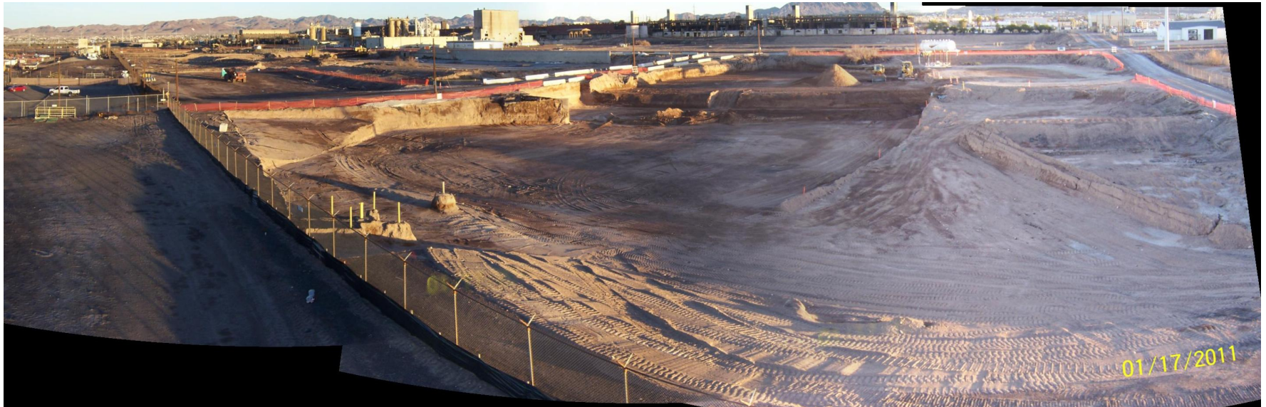
South RZ-C-1 through 4 Polygon Excavation
