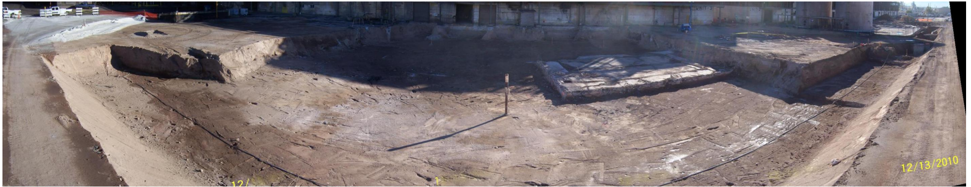
North Side of Unit Buildings 3 Finished Polygon Excavation
