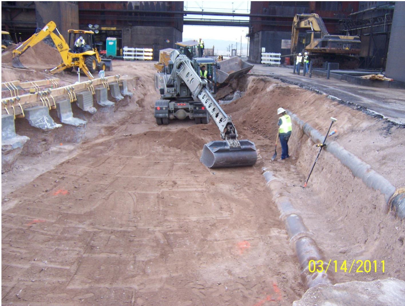
RZ-B-19,20,21 Polygon Excavation Finish Grading around Utilities
