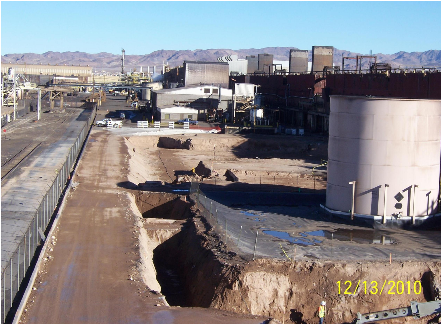
North Side of Unit Buildings 2 & 3 Polygon Excavation
