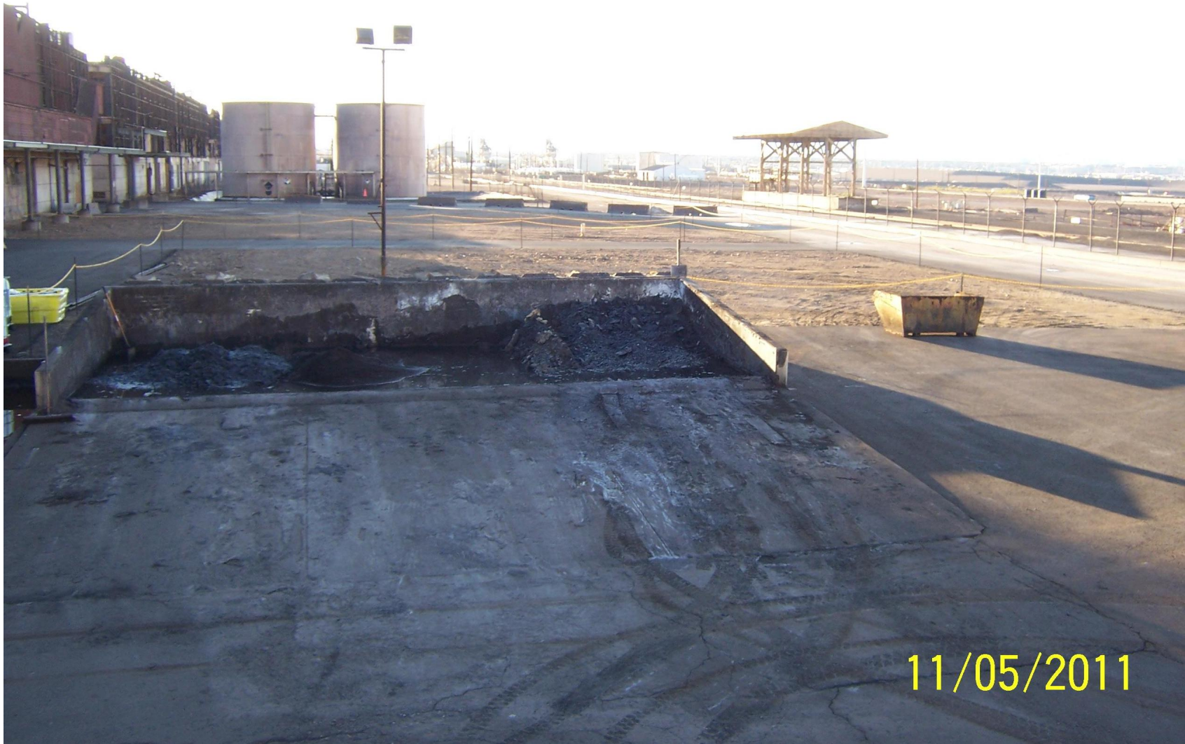
North Side of Unit Buildings 3 Finished Polygon Backfill
