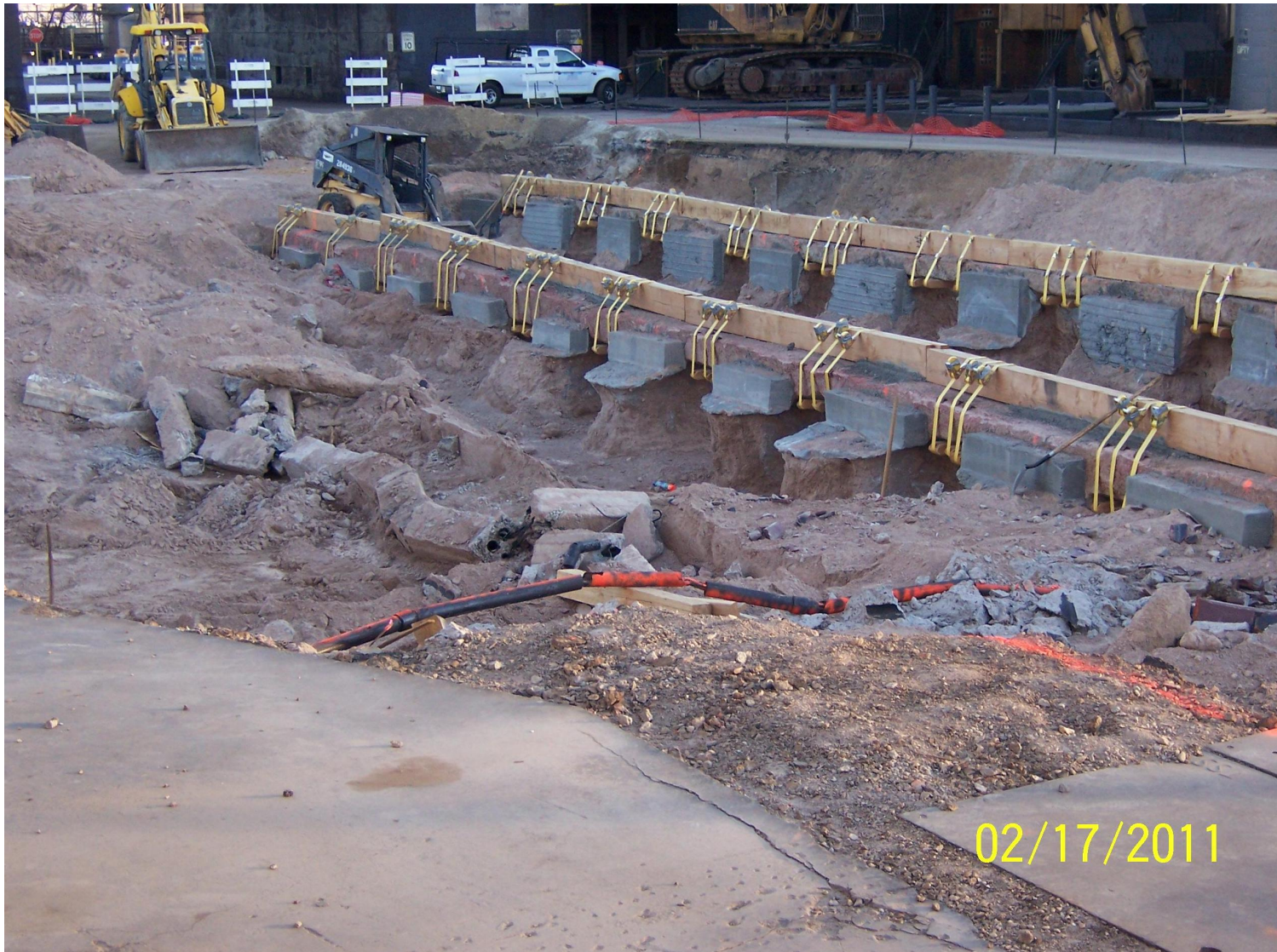
RZ-B-19,20,21 Polygon Excavation with Utility Underpinning
