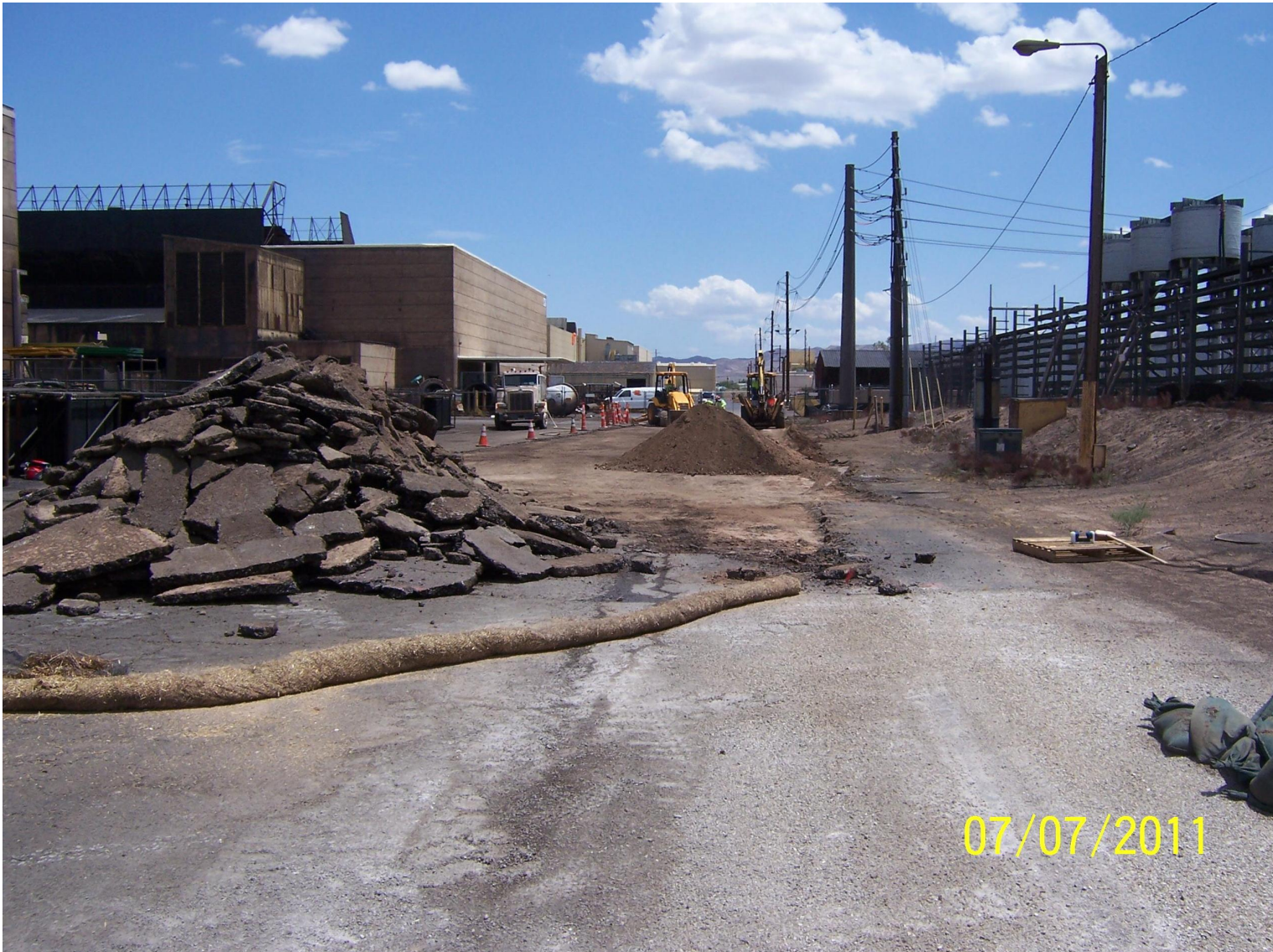
RZ-B-23A During Polygon Excavation
