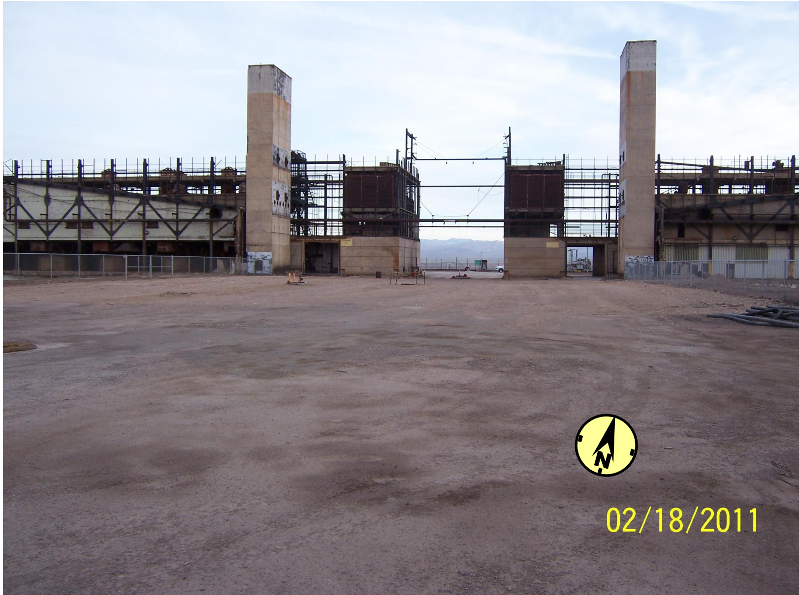
South Side of Unit Building #1 & 2 Finished Polygon Excavation, No Backfill
