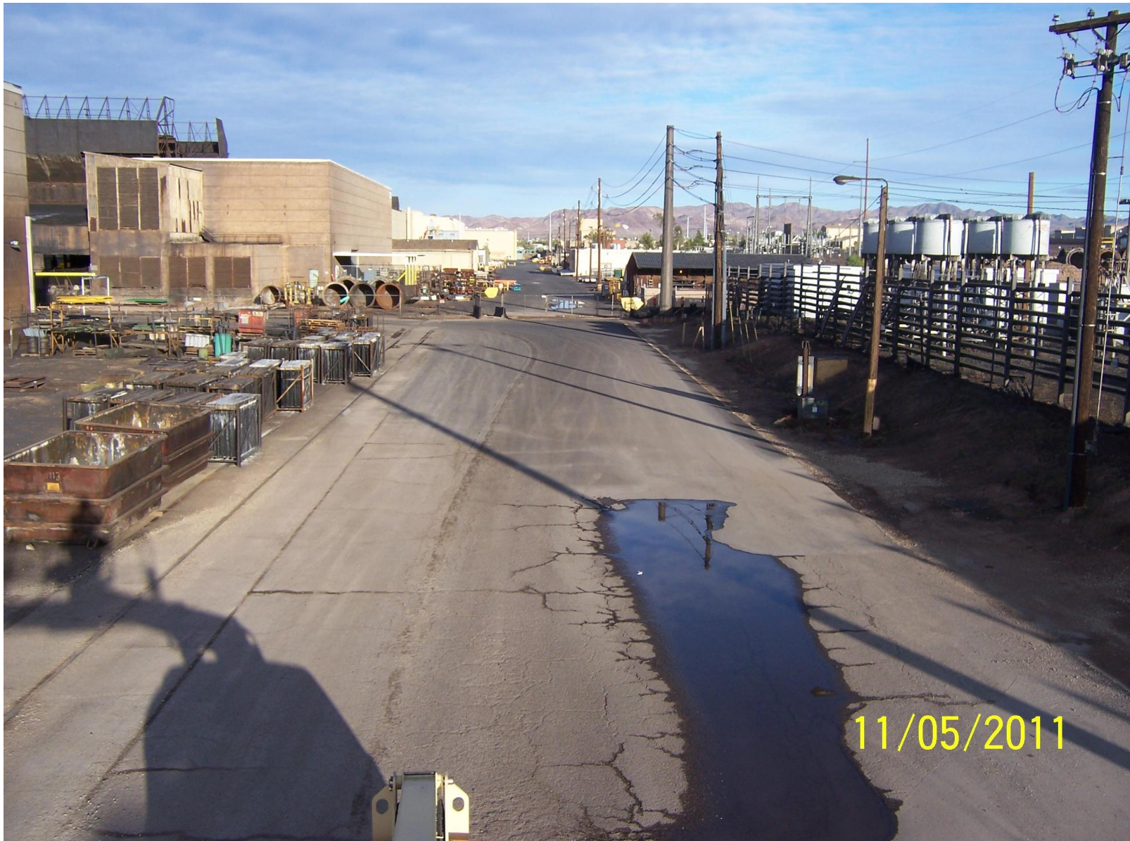
RZ-B-23A Area Backfilled with Chat and Paved with Asphalt
