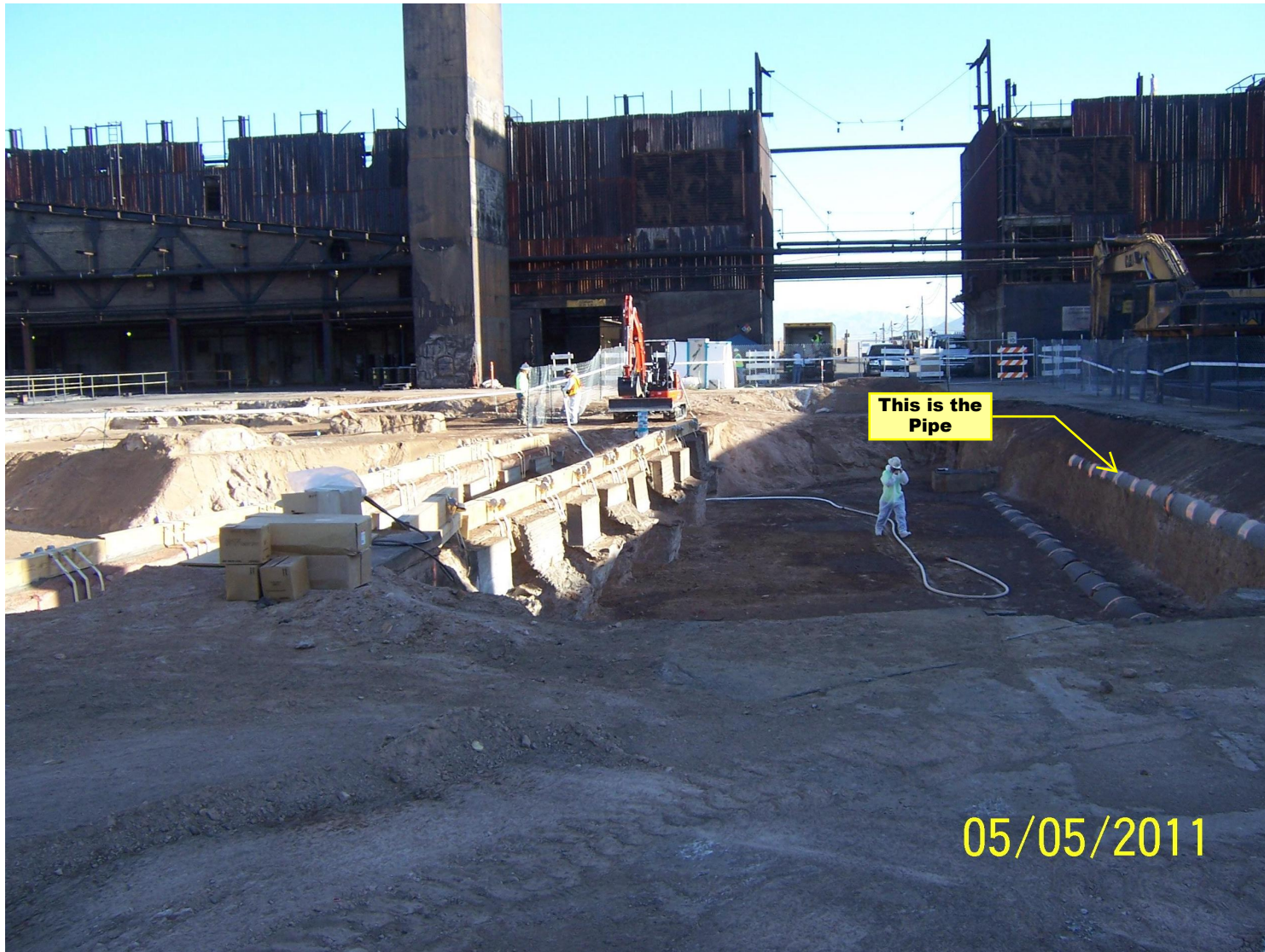
RZ-B-19,20,21 Removal of Pipe Containing Asbestos
