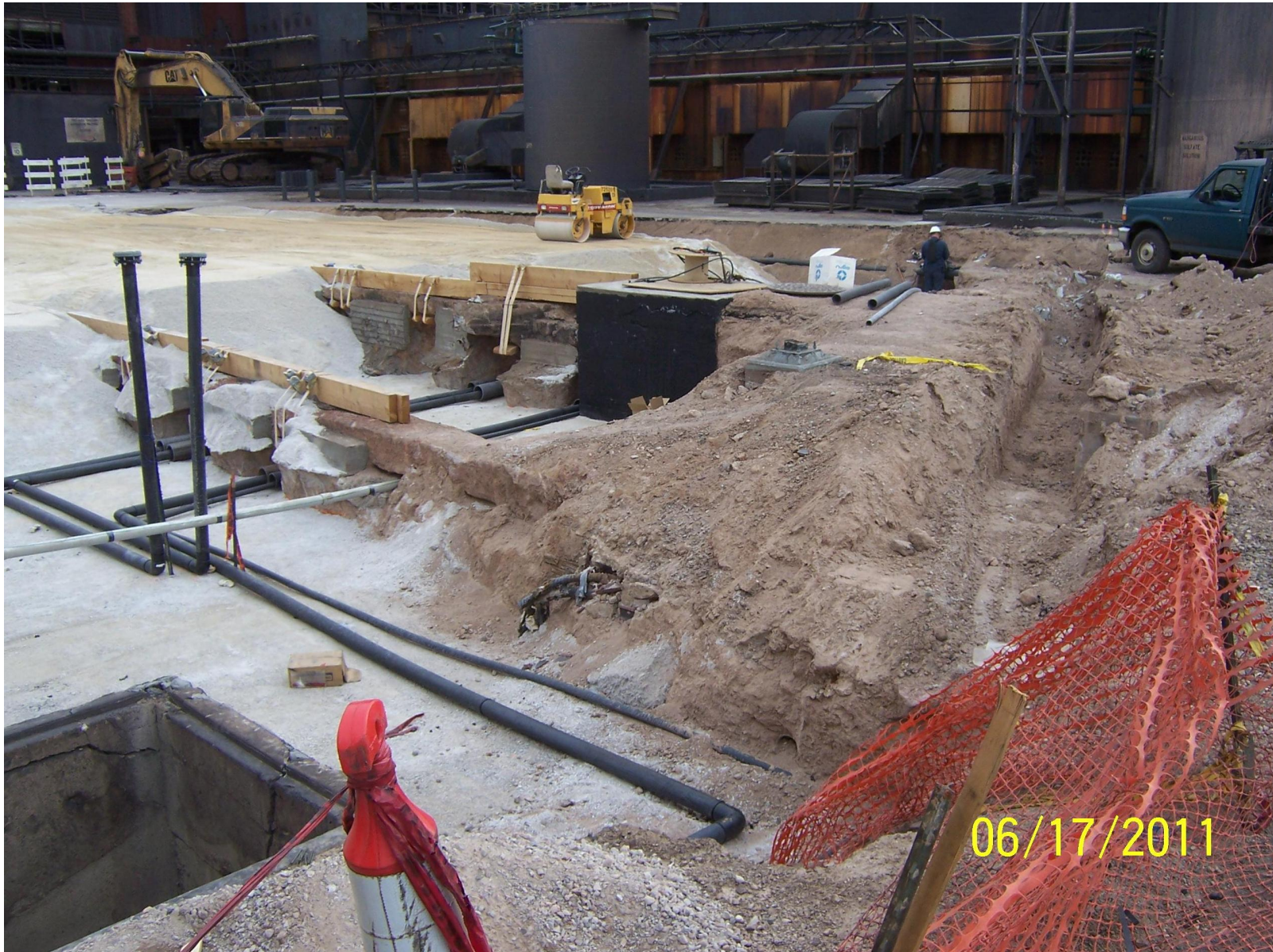
RZ-B-19,20,21 Piping Installed by Tronox for New Addition
