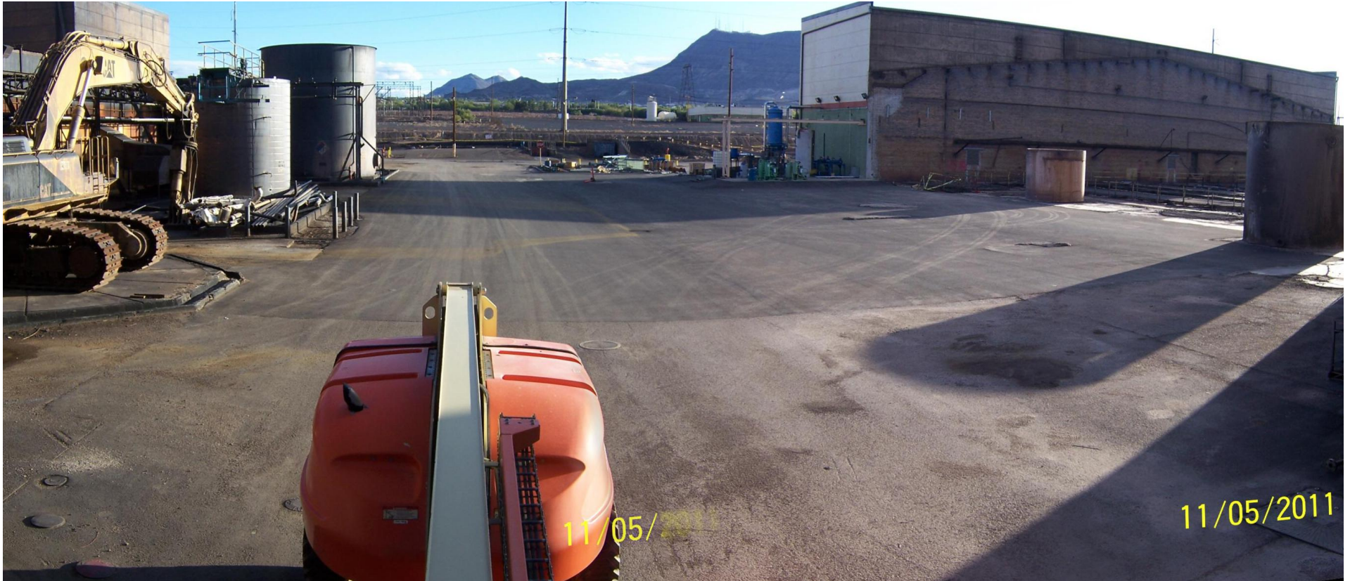
RZ-B-19,20,21 Area Backfilled with Chat and Paved with Asphalt
