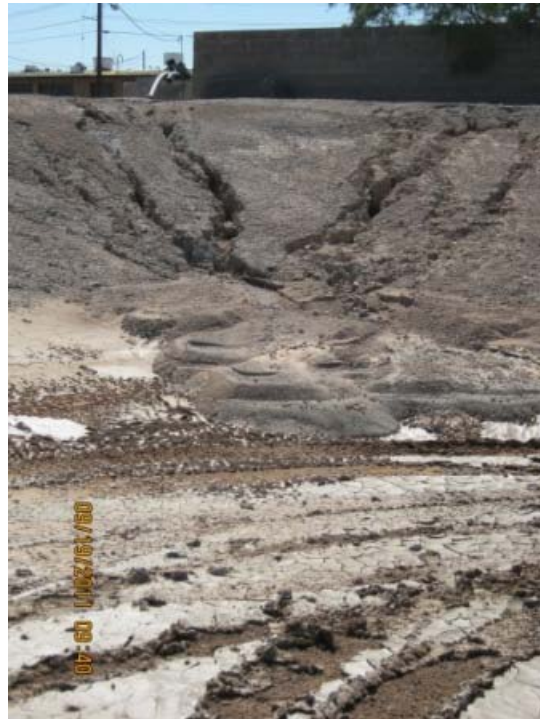
Area 4: RZ-E-4. Will install directional berm(s) to flow into channel at designated location. Slope at inflow will include placement of nonwoven geotextile with 12" of 6" angular stone.
