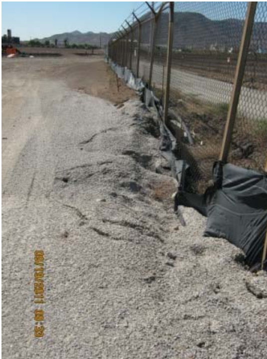
Area 1: West Property Line – Repair. Removal of silt fence once construction is complete allowing flow through culvert as designed, minimizing sheet flow over road and flow around culvert. Area around culvert will be repaired.
