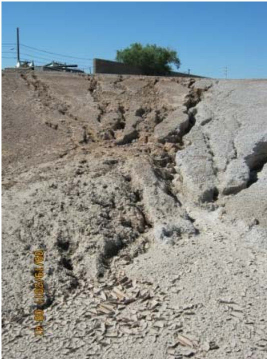
Area 4: RZ-E-4. Will install directional berm(s) to flow into channel at designated location. Slope at inflow will include placement of nonwoven geotextile with 12" of 6" angular stone.
