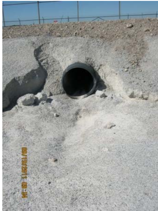
Area 1: West Property Line – Repair. Removal of silt fence once construction is complete allowing flow through culvert as designed, minimizing sheet flow over road and flow around culvert. Area around culvert will be repaired.
