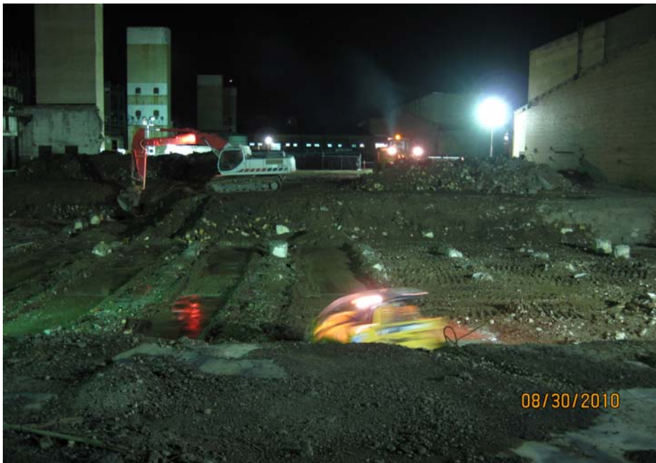
Looking east, Skid Steer working the floor.
