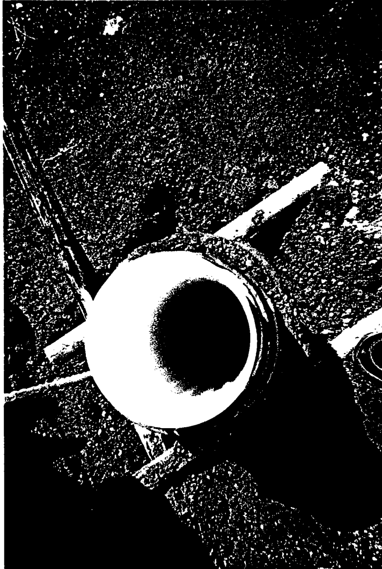
PHOTOGRAPH 9: Close-up inside view of the 20-slot, Bort-Longyear "Circumslot" PVC screen to show the internal ribbing that supports the single piece of PVC extrusion, which permits the continuous-wrap, circumferential slotting. Pittman Lateral, Henderson, Nevada; 9/12/98.
