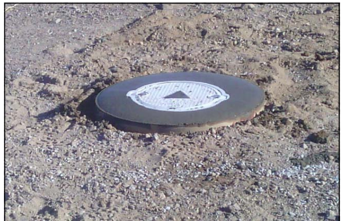
Typical Monitoring Well Surface Completion
