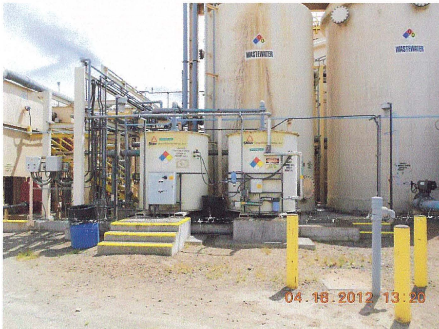
Fig. 7 – GAC Odor Control for Gaseous Emissions
