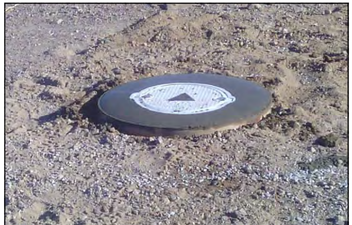
Typical Monitoring Well Surface Completion
