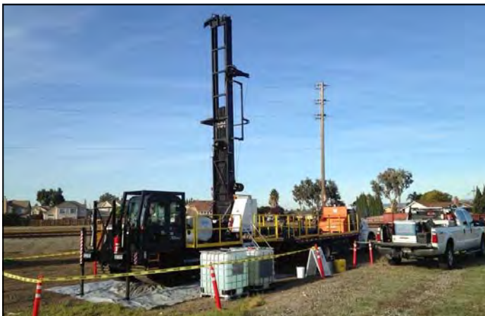
Typical Drill Rig to Be Used
