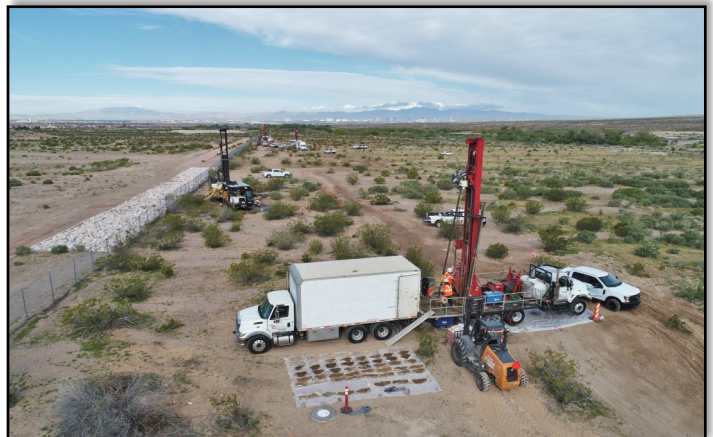
Installation of monitoring wells near the Las Vegas Wash, April 2020
