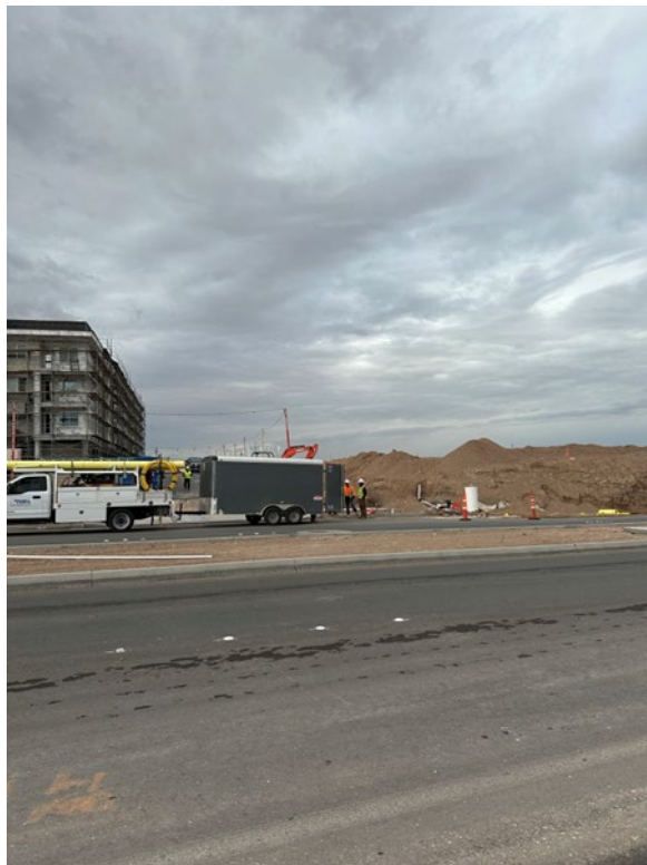
Photo 4b: Apartments being constructed on the former BMI pond areas (June 2022).
