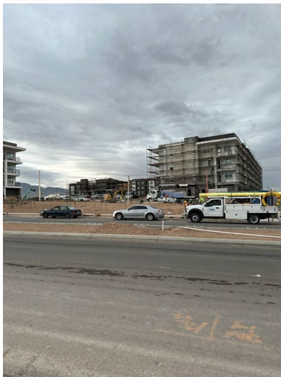
Photo 3b: Apartments being constructed on the former BMI pond areas (June 2022).
