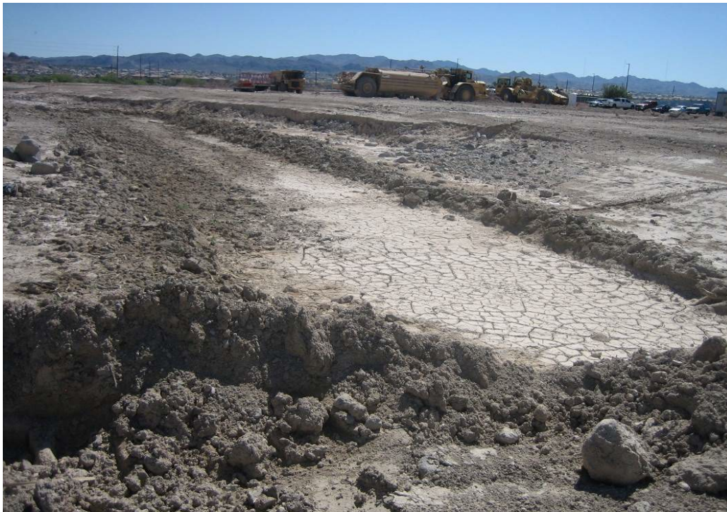
Photo 3a: Excavated areas near former BMI ponds (April 2018).
