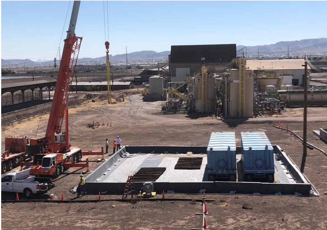
Secondary containment constructed and influent tanks installed.
