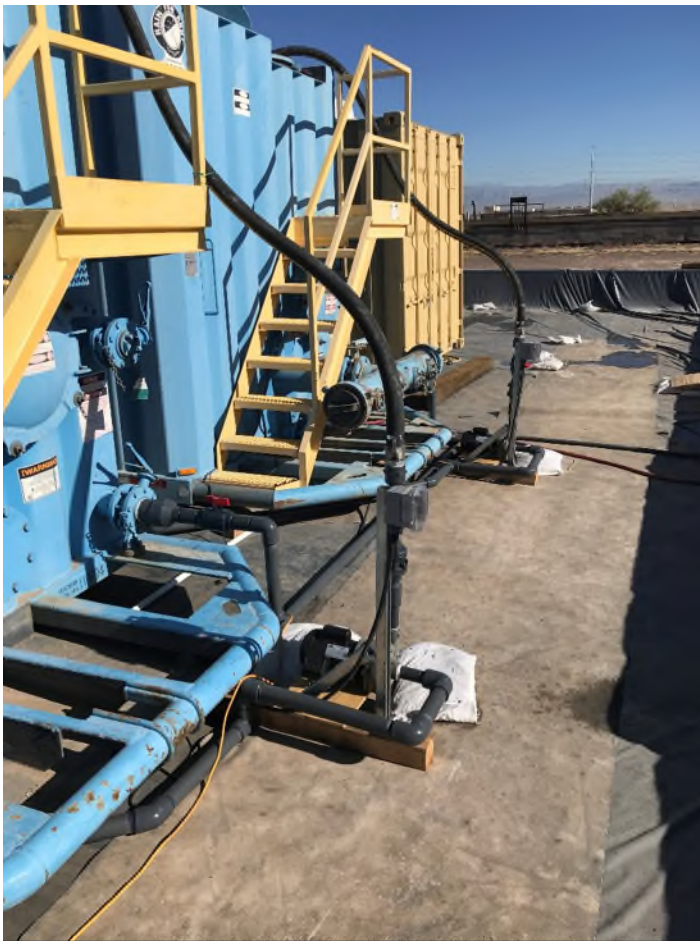
Influent tank recirculation pumps and piping.
