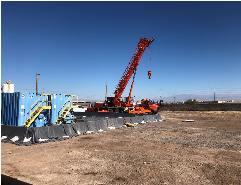
Crane setup to place Pilot Unit containers.
