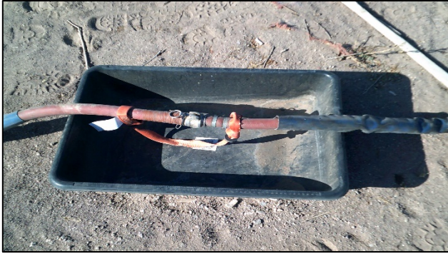
9. Hose connection with nylon whip check and secondary containment.
