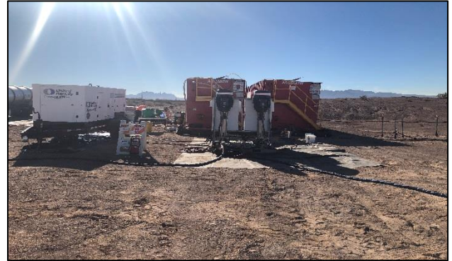
4. Injection pump and containment berm
