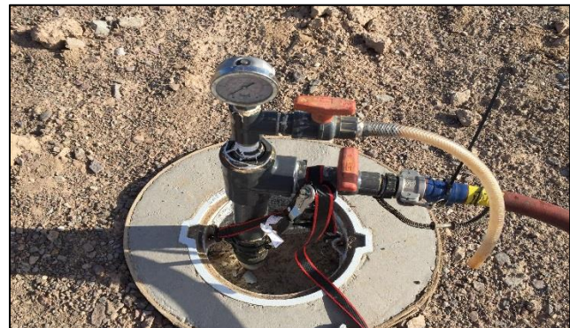
6. Injection well connection
