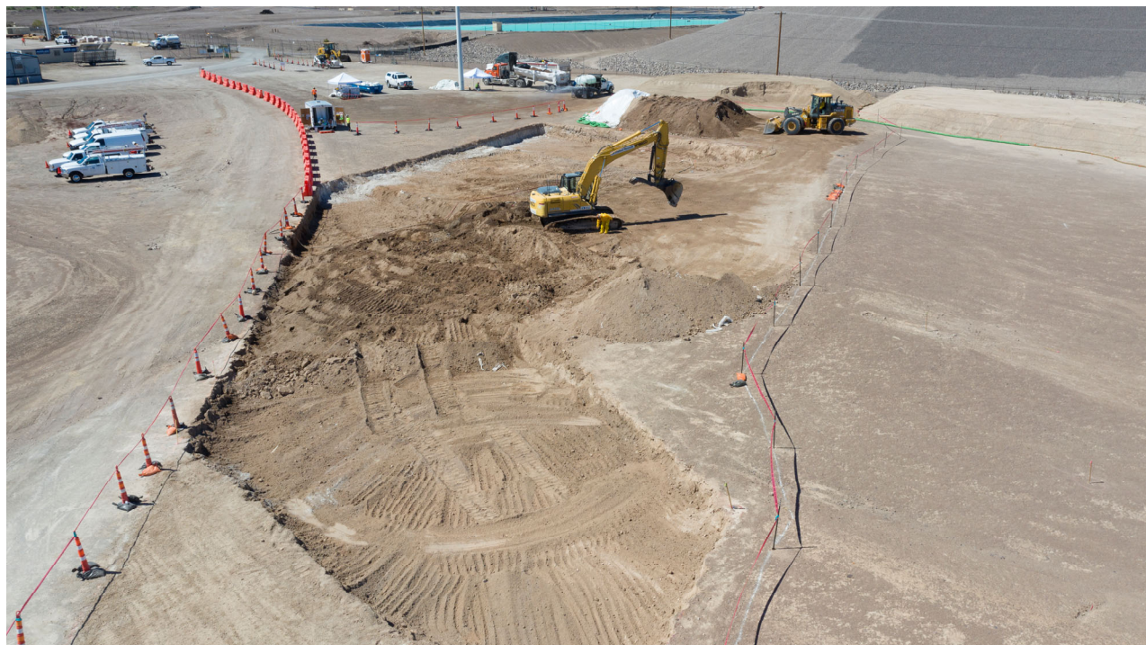
Photo 8: April 18, 2019. Excavation of non-ECA area nearing completion. View to southwest.
