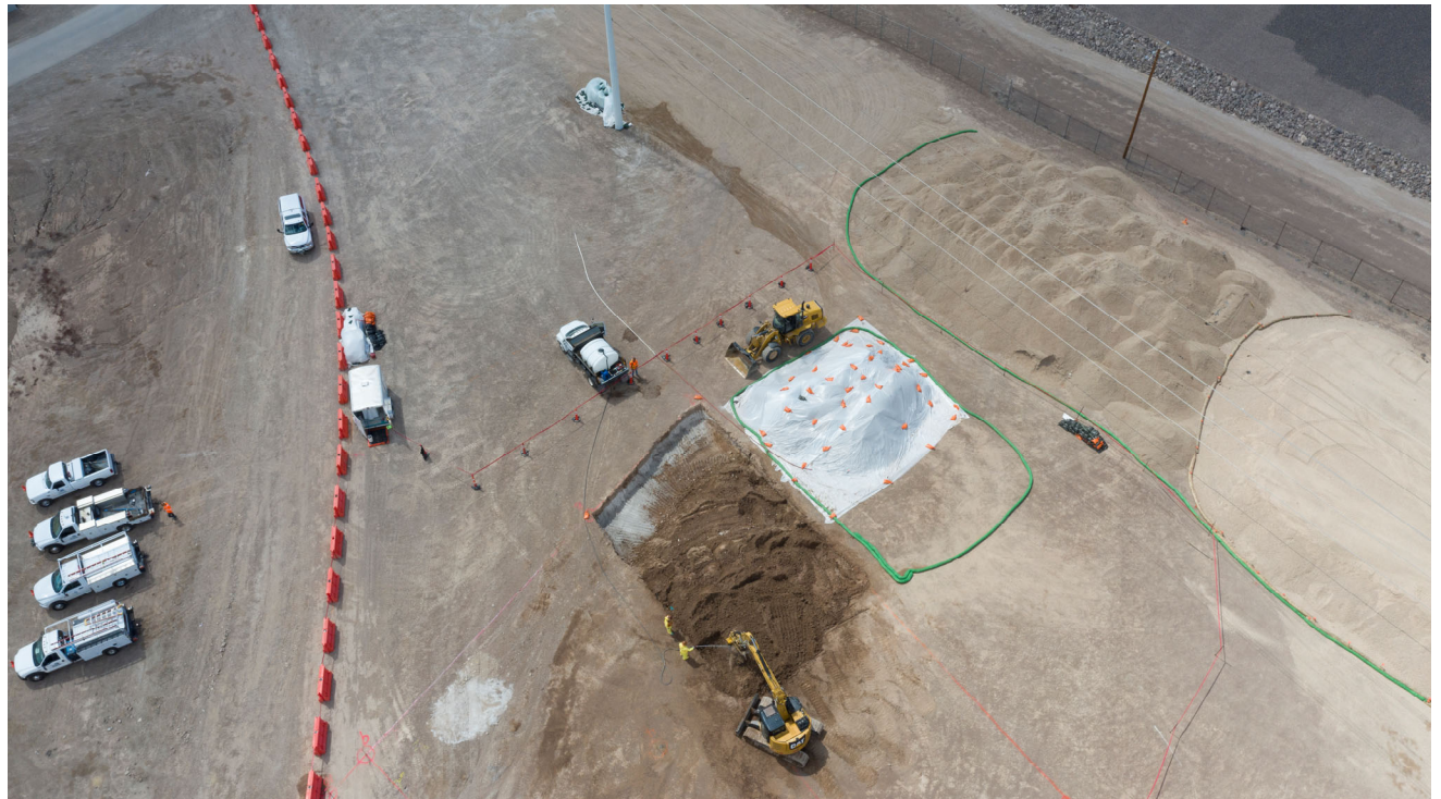
Photo 2: April 2, 2019. Excavation of southwest portion of non-ECA area. View to southwest.
