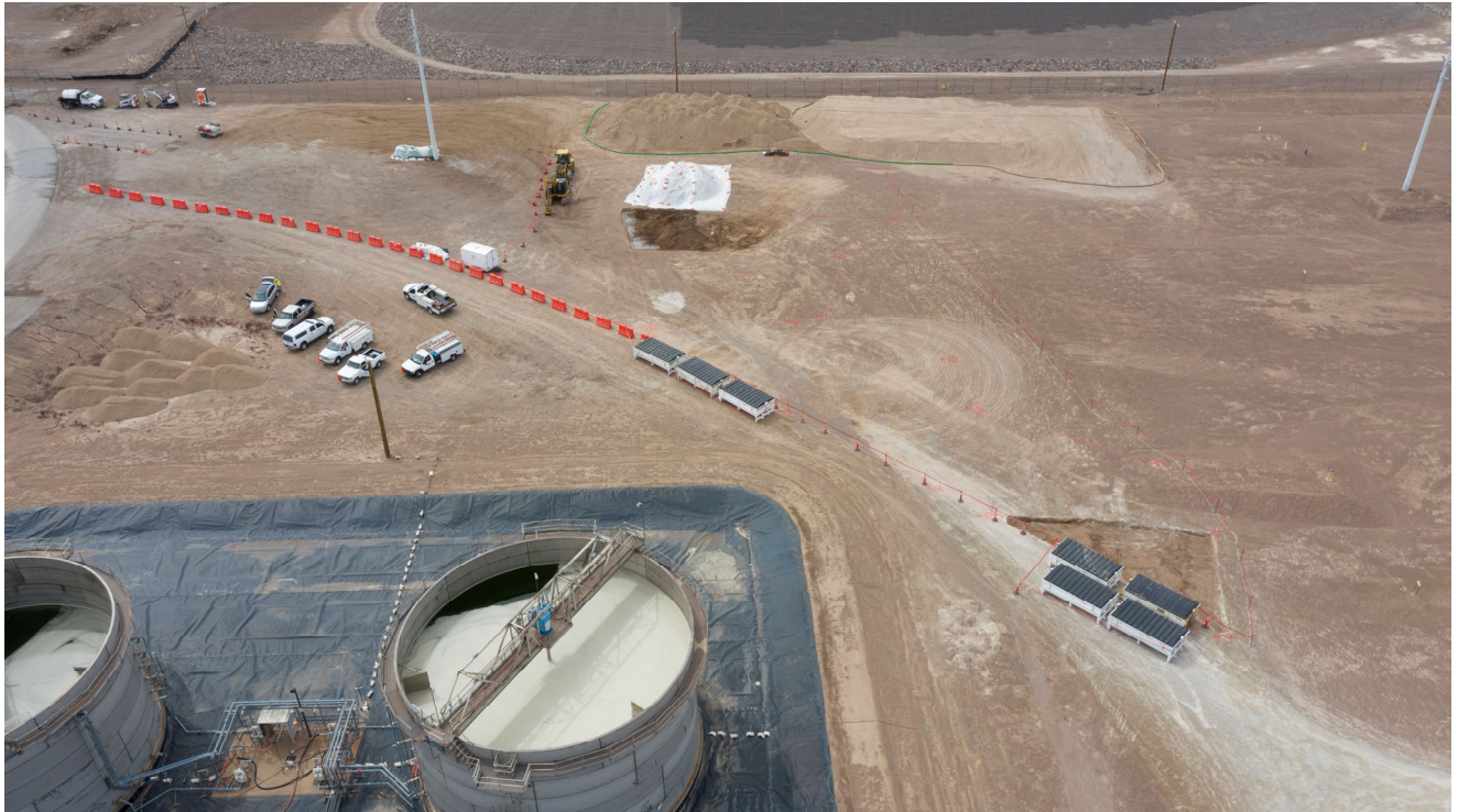
Photo 1: April 1, 2019, first day of excavation activities. Triangular ECA area excavated into bins. Start of excavation of Non-ECA area. Backfill material in background. View to west.
