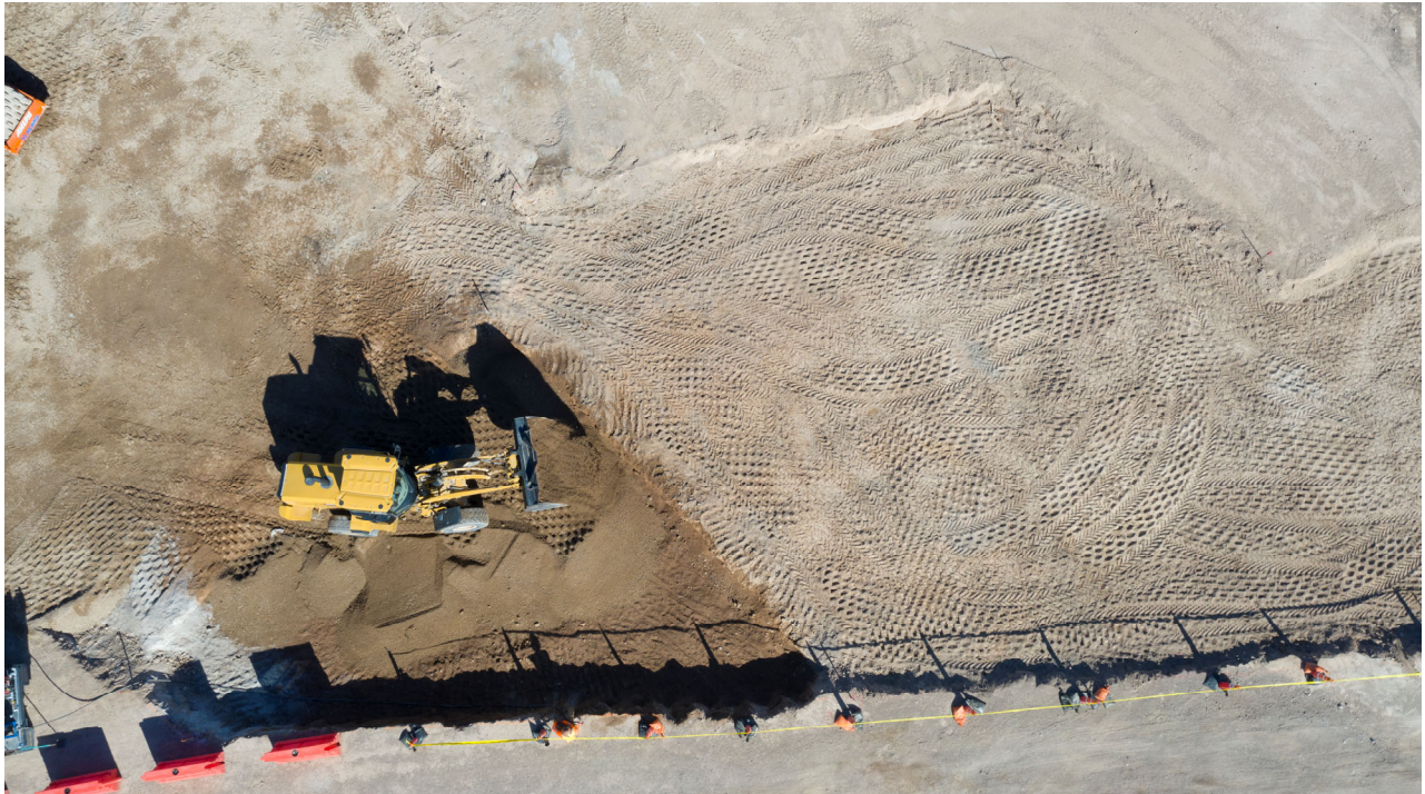
Photo 9: April 20, 2019. Backfilling and compaction of the non-ECA excavation area.
