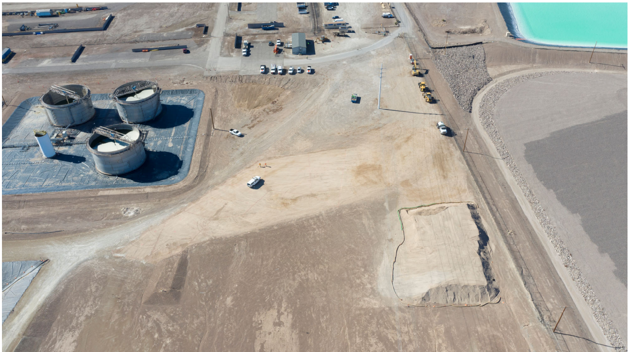
Photo 10: April 24, 2019. Project site at completion of backfilling and restoration. View to south.
