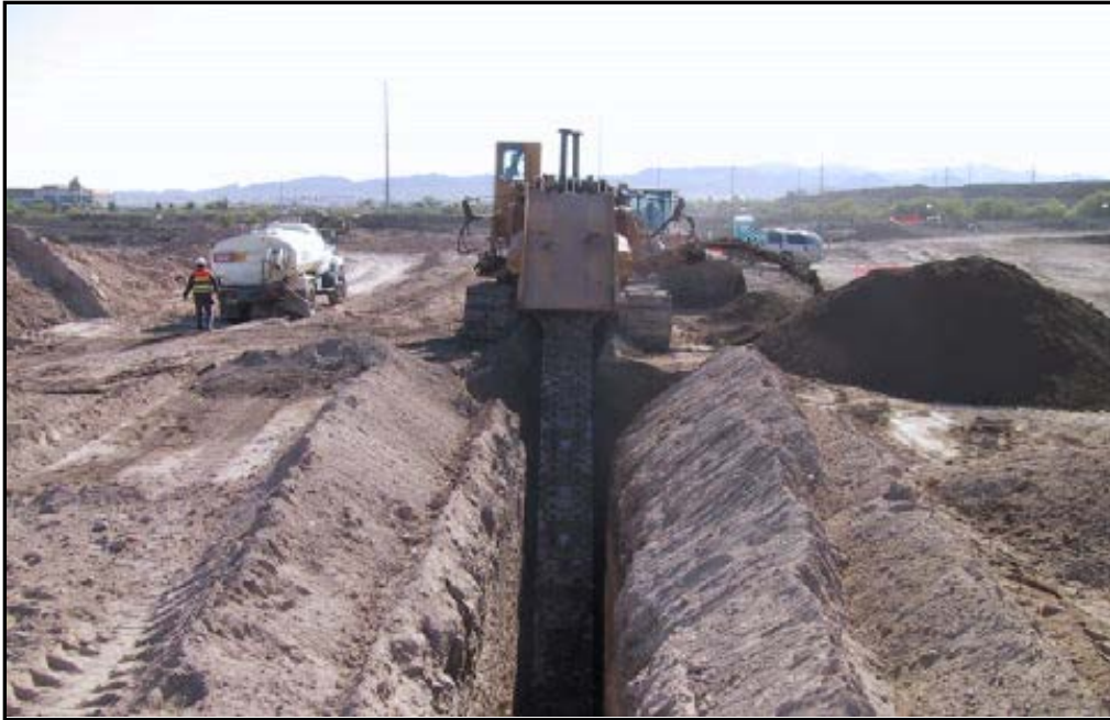
Figure 3 – Subsurface Barrier Wall Construction
