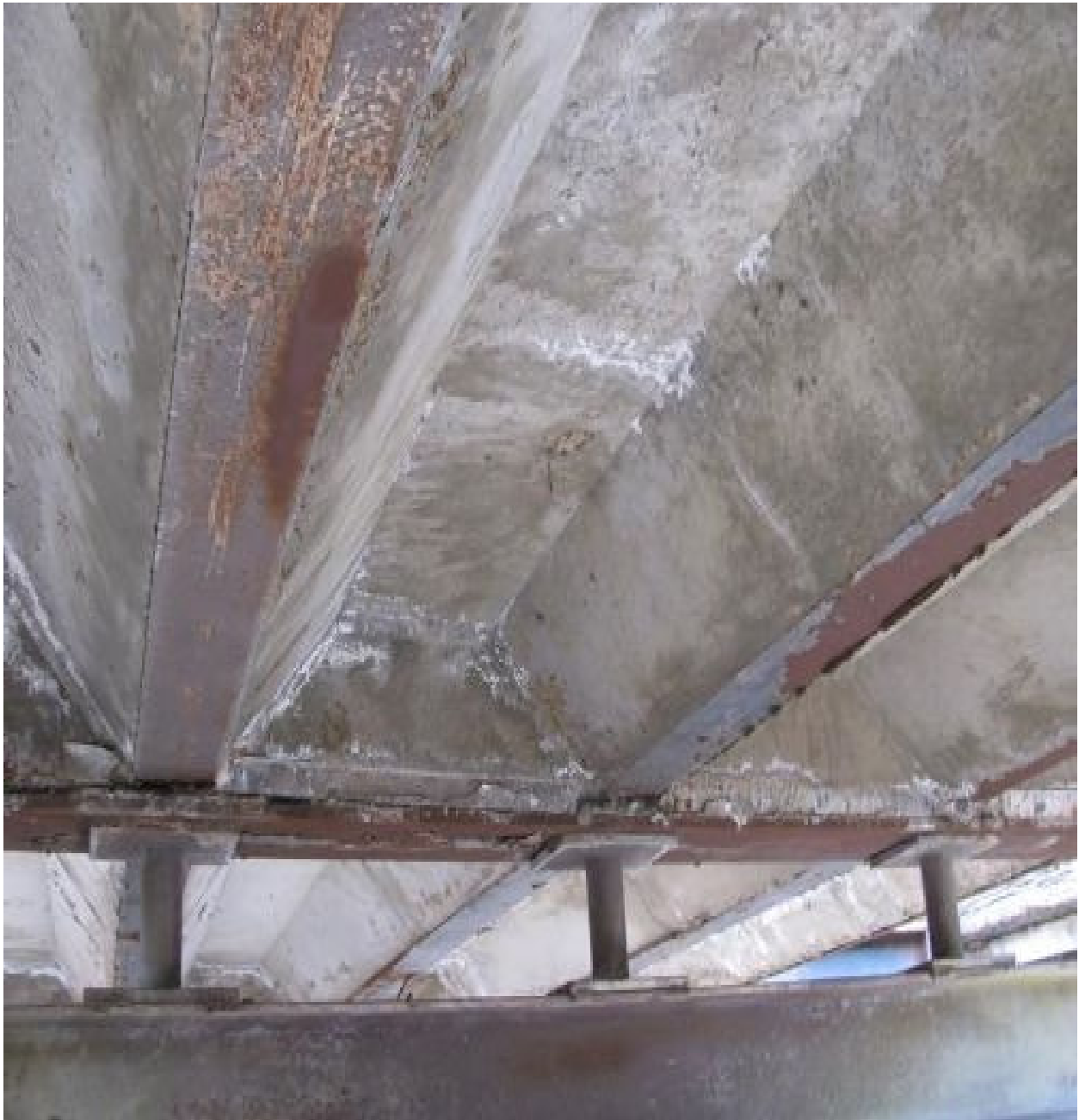
Figure 23: Typical cell floor concrete encasement
