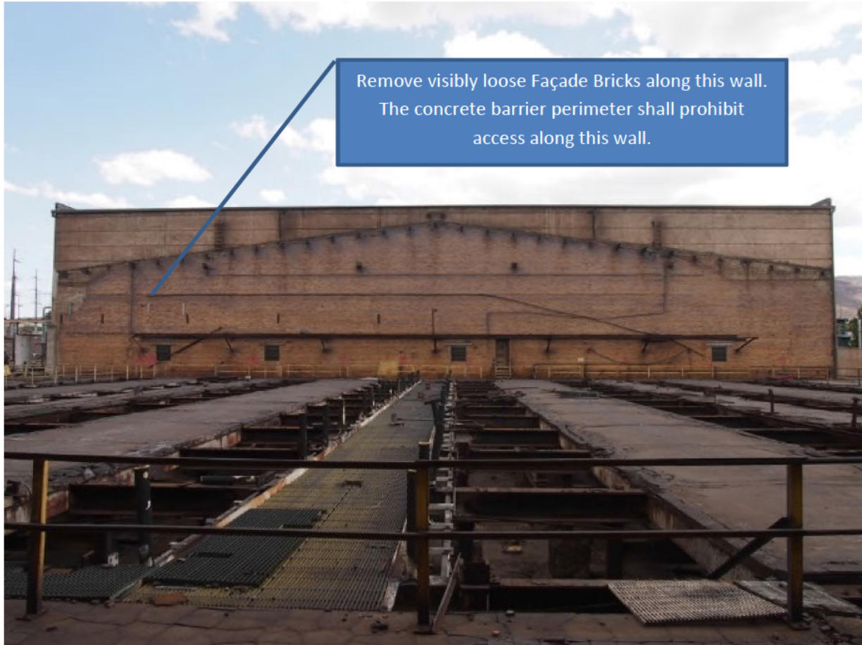
Figure 1: North Wall of Substation Building
