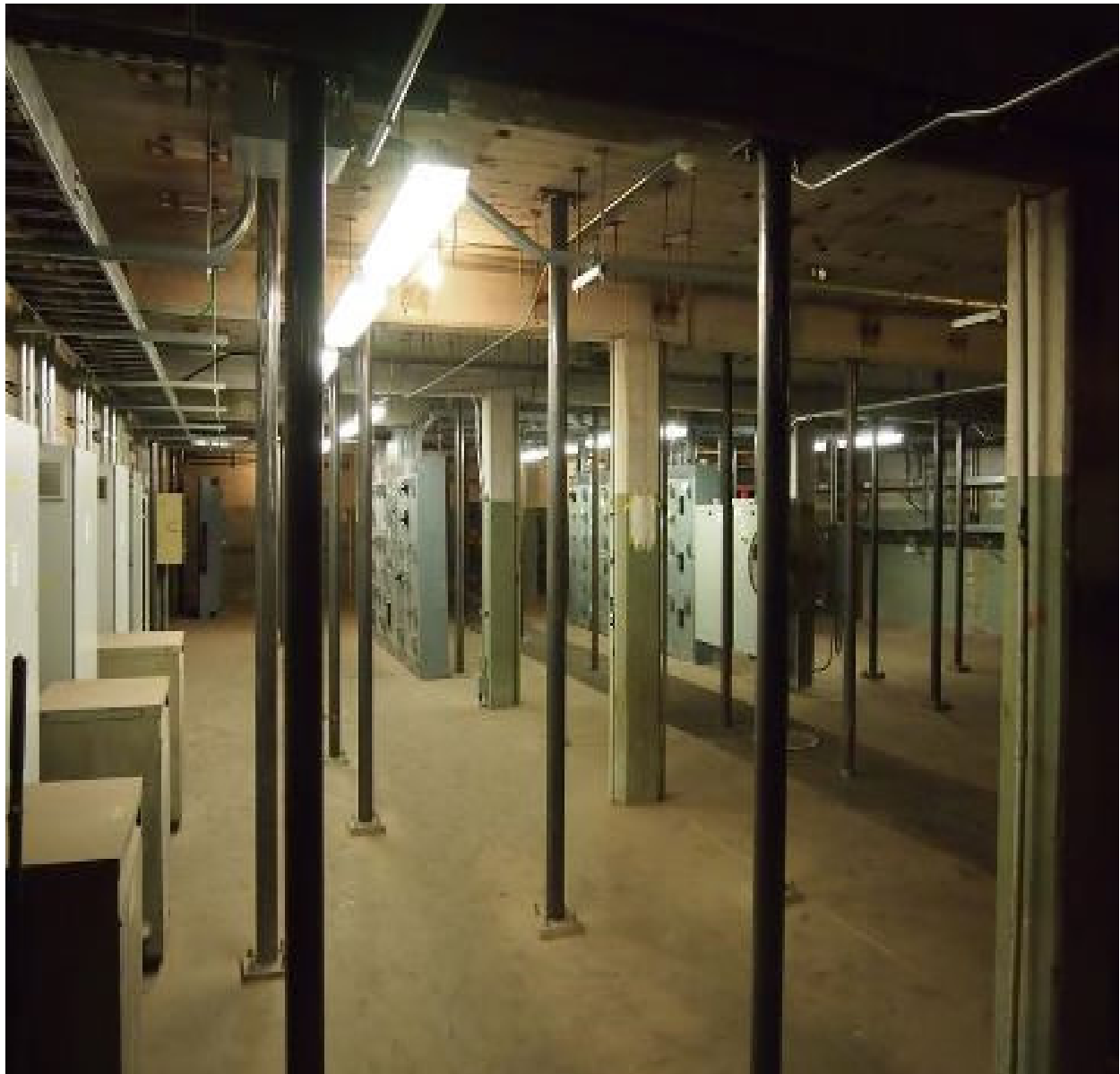
Figure 11: Floor reinforcing columns, Unit 4 Substation Building
