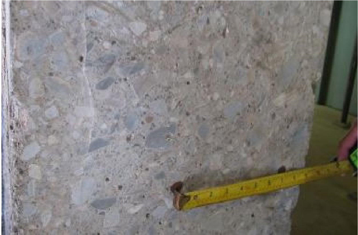
Figure 14: Basement wall section at doorway to Cell Floor
