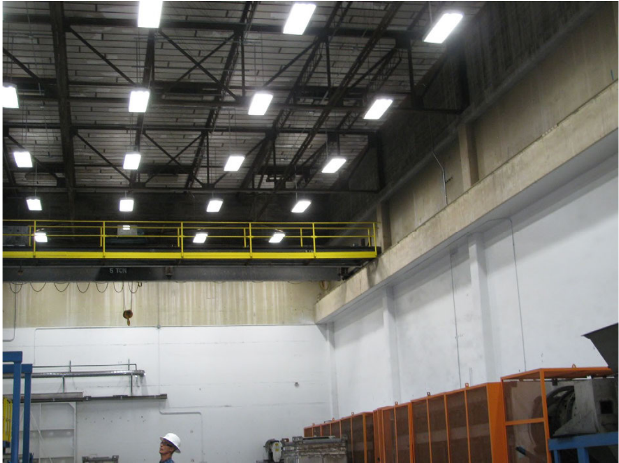
Figure 6: Main Floor of Substation Building
