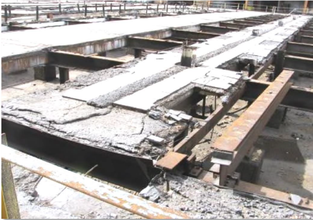
Figure 3. Unit 4 Cell Island Slab and separation
