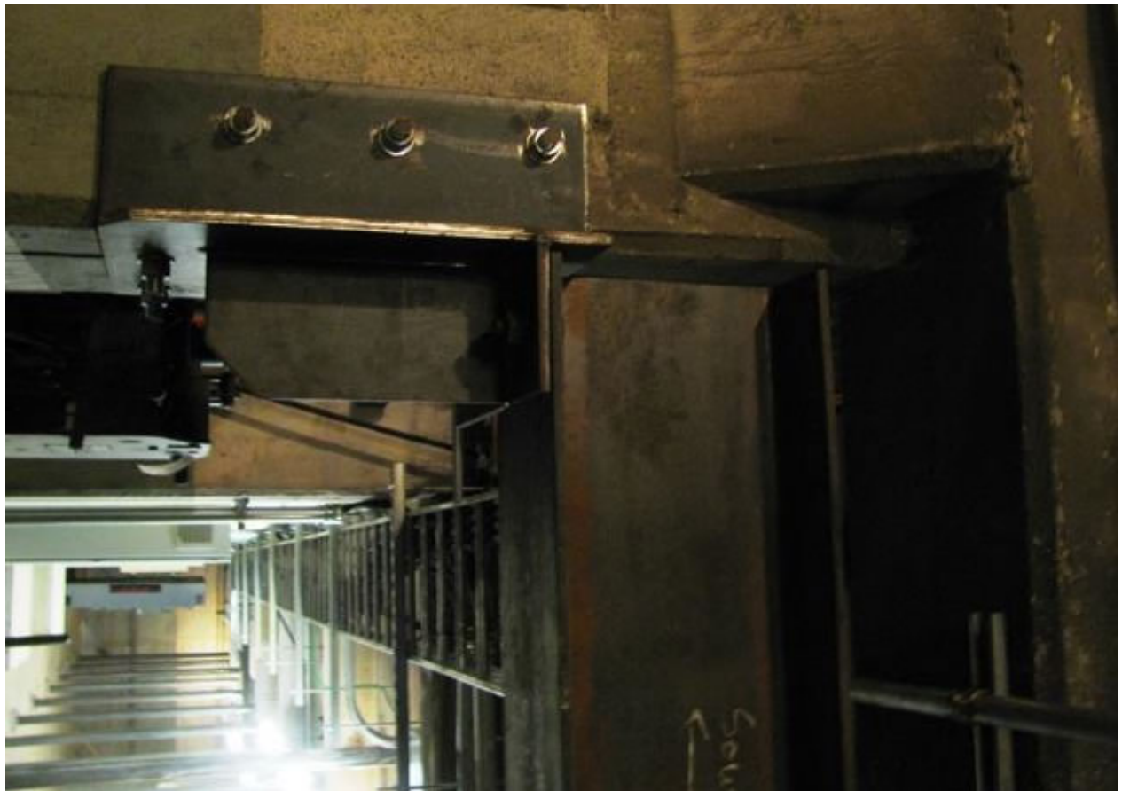
Figure 8: Floor reinforcing bracket, Unit 4 Substation Building
