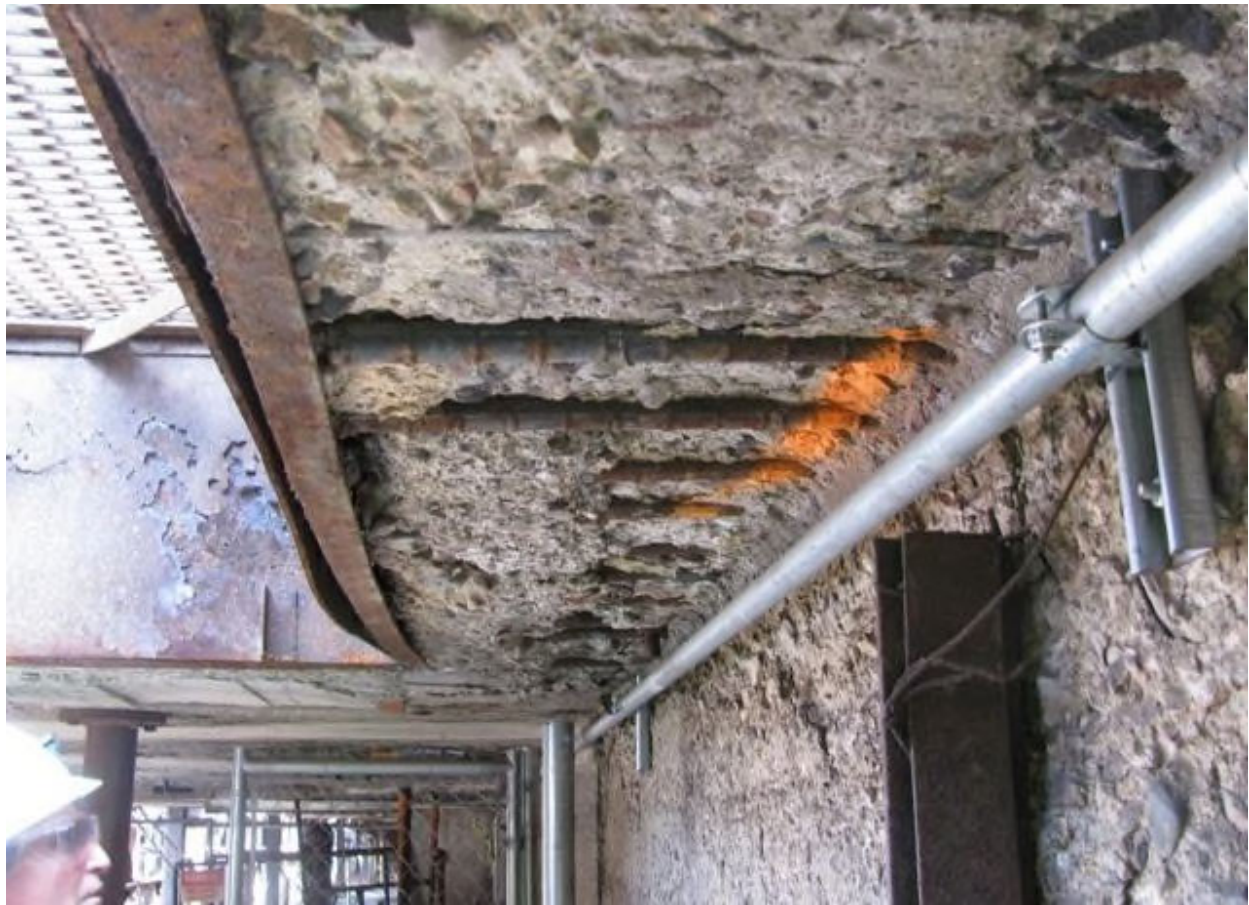
Figure 15: Curtain slab of Unit 4 Cell Floor near Substation Building foundation wall
