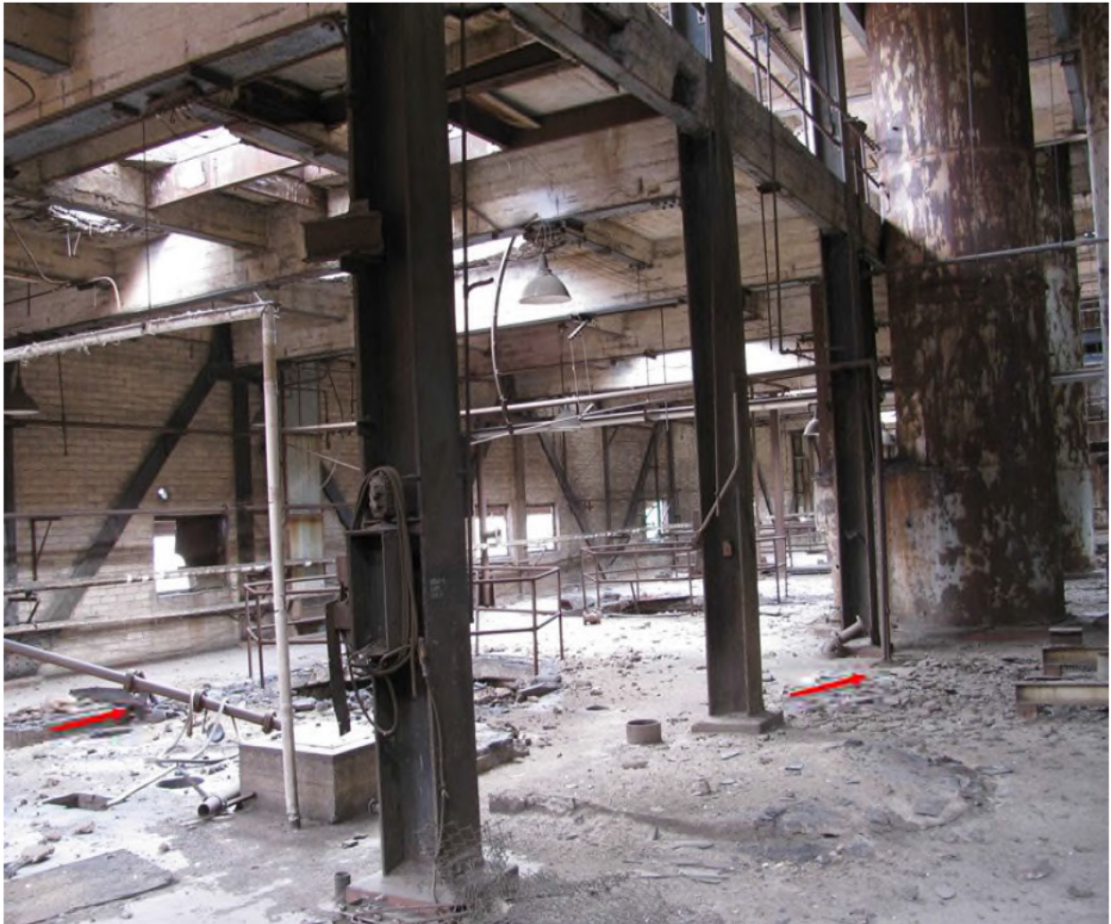
Figure 33: Unit 4 Chlorinator Building – second level
