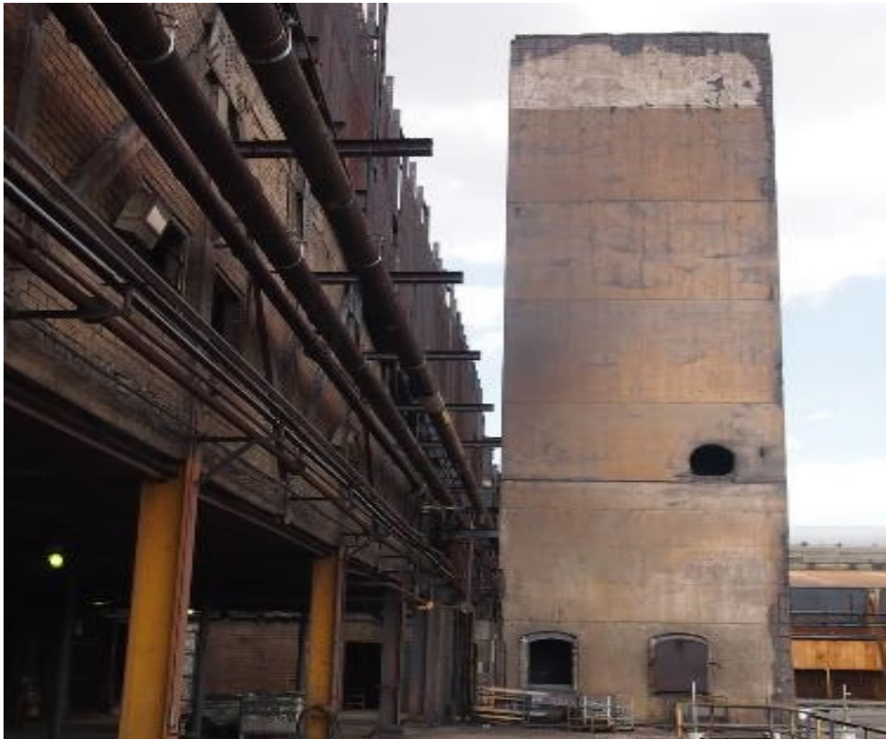
Figure 5: Unit 4 Wash Down Tower, looking east
