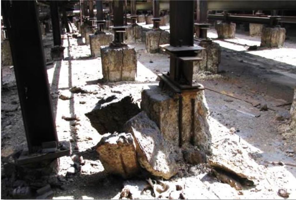
Figure 5. Steel Column Concrete Pedestal on the Unit 4 Cell Building basement floor
