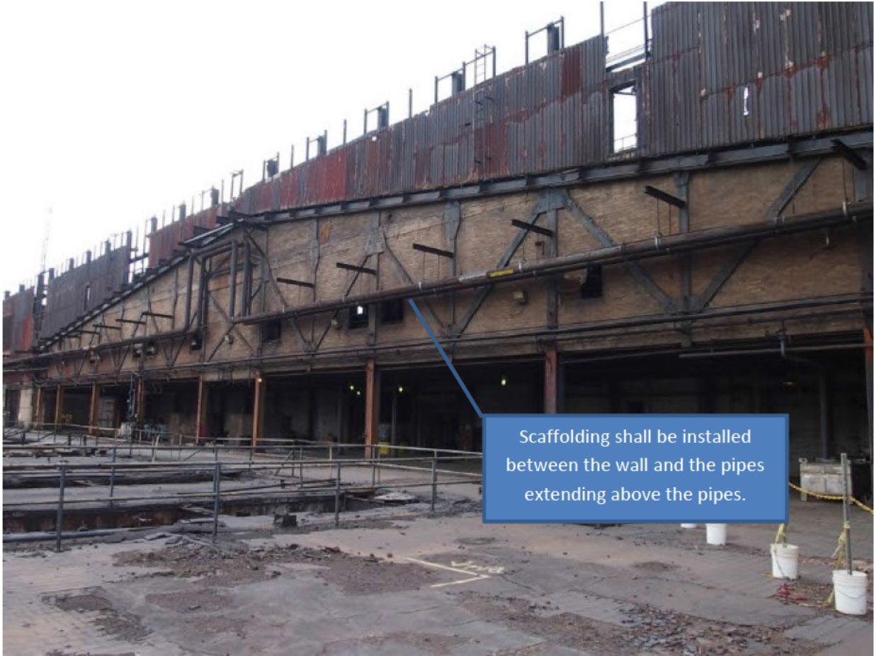
Figure 2: South Wall of Chlorinator Building
