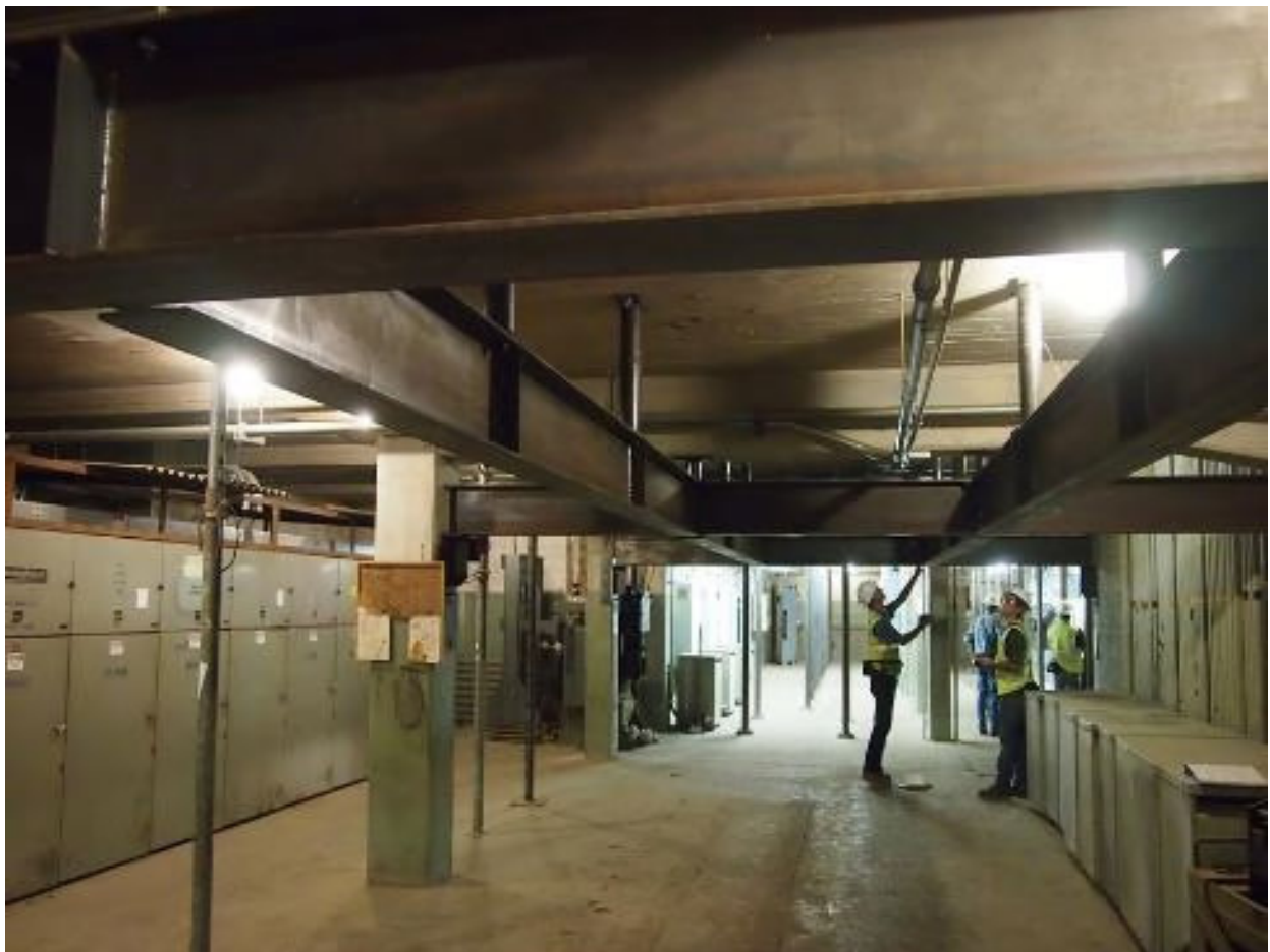
Figure 10: Floor reinforcing beams, Unit 4 Substation Building
