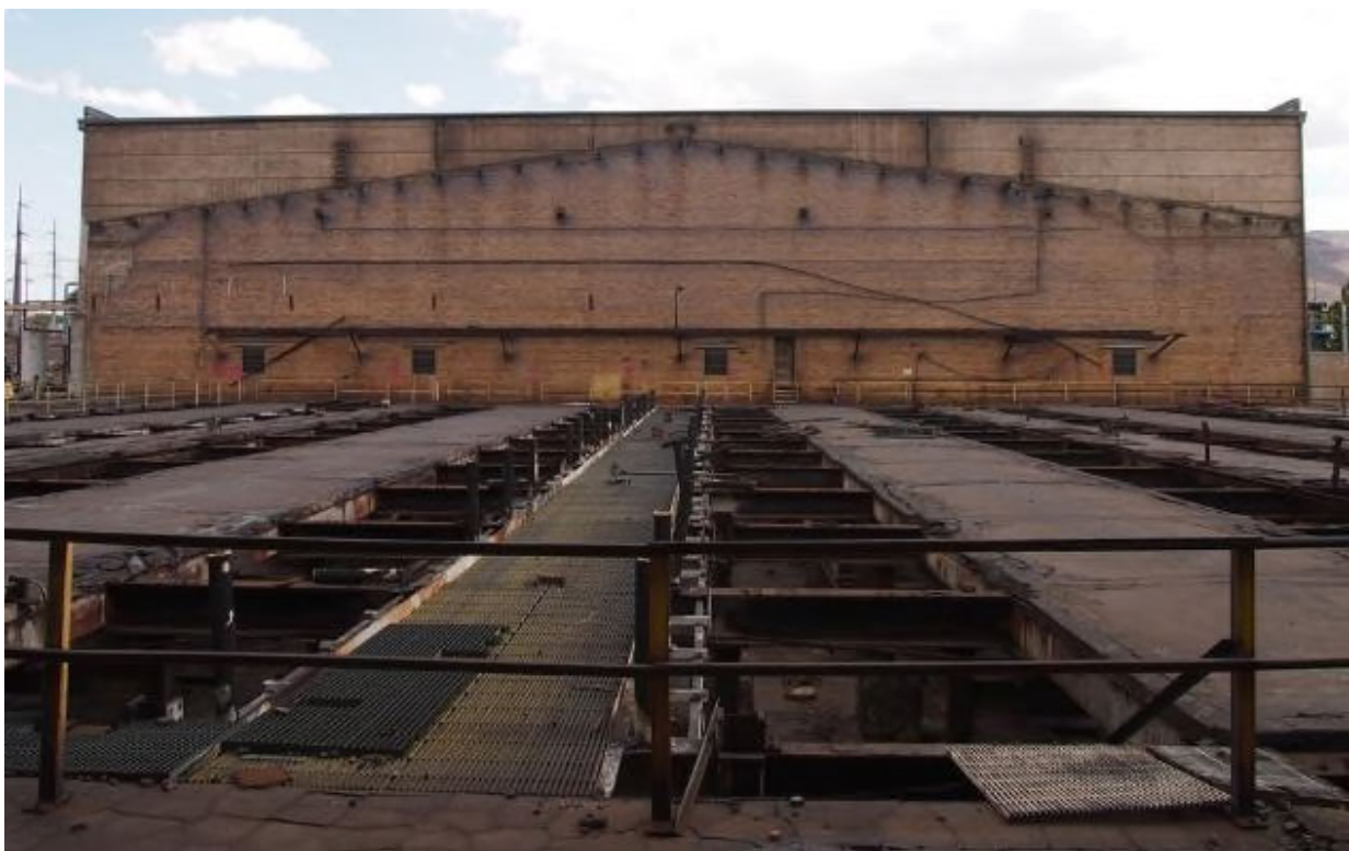
Figure 3: Unit 4 Substation Building brick wall, looking south
