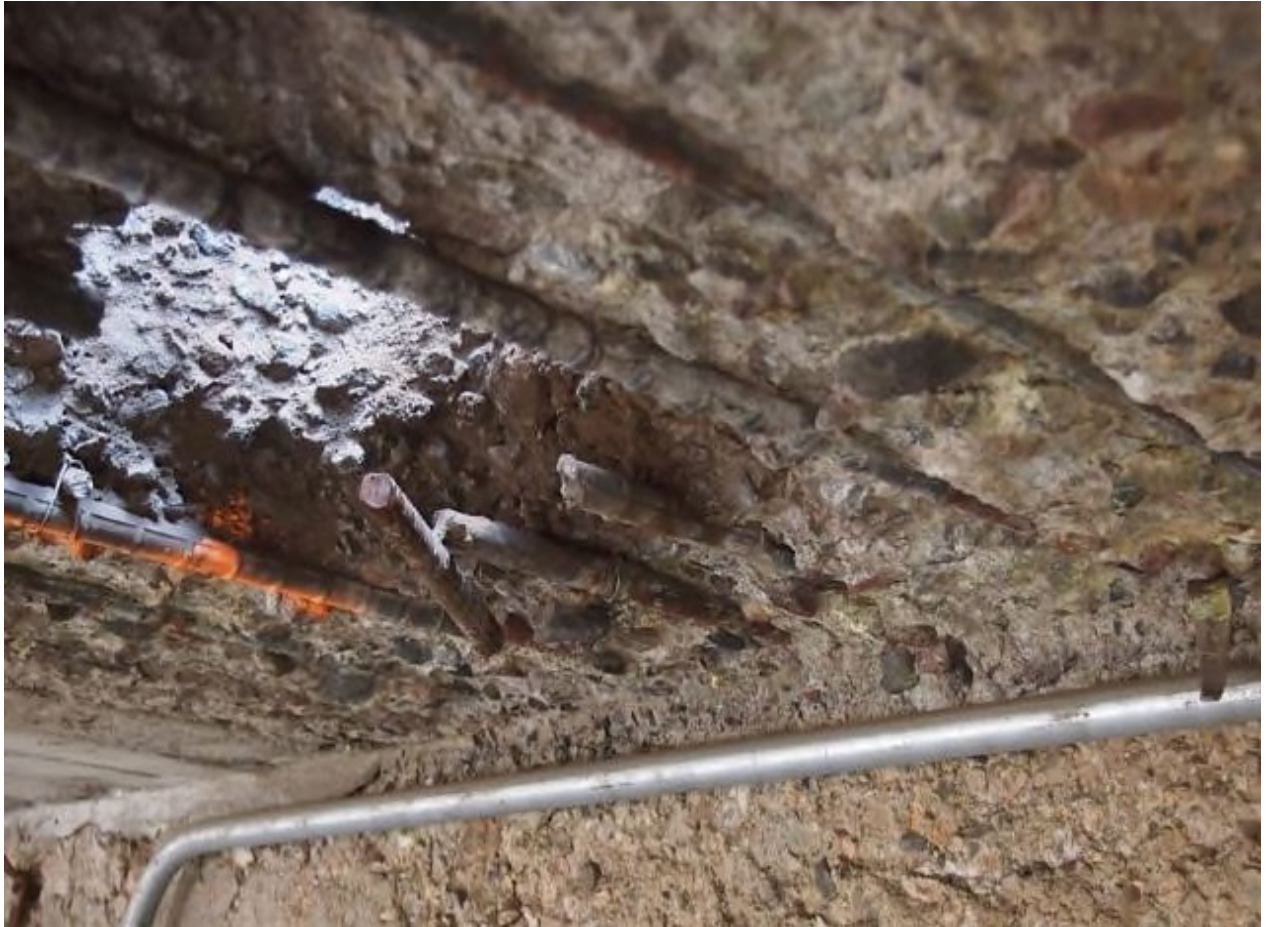
Figure 16: Curtain slab of Cell Floor near Unit 4 Substation Building foundation wall
