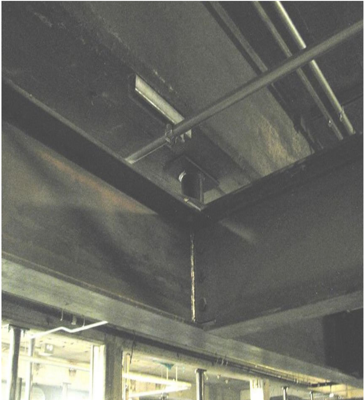
Figure 9: Floor reinforcing beams, Unit 4 Substation Building
