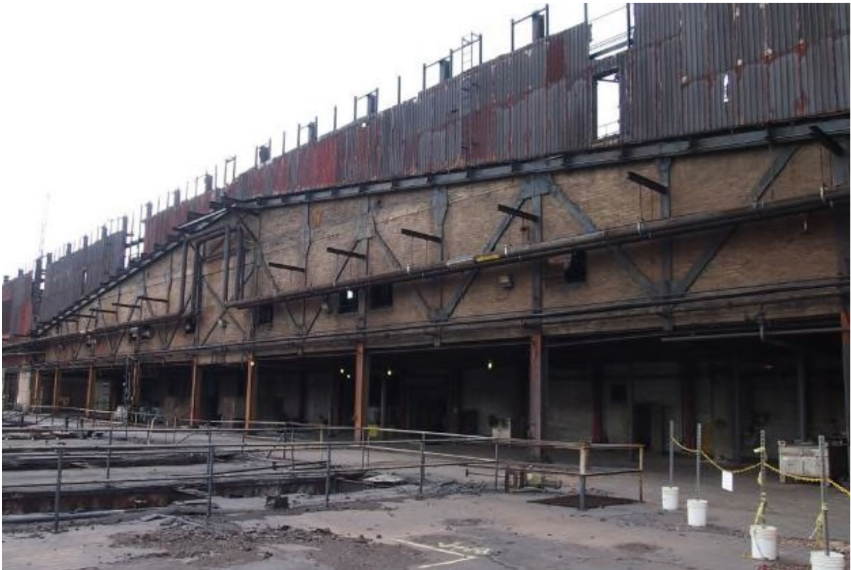
Figure 37: Unit 4 Chlorinator Building - integrated roof truss along south side
