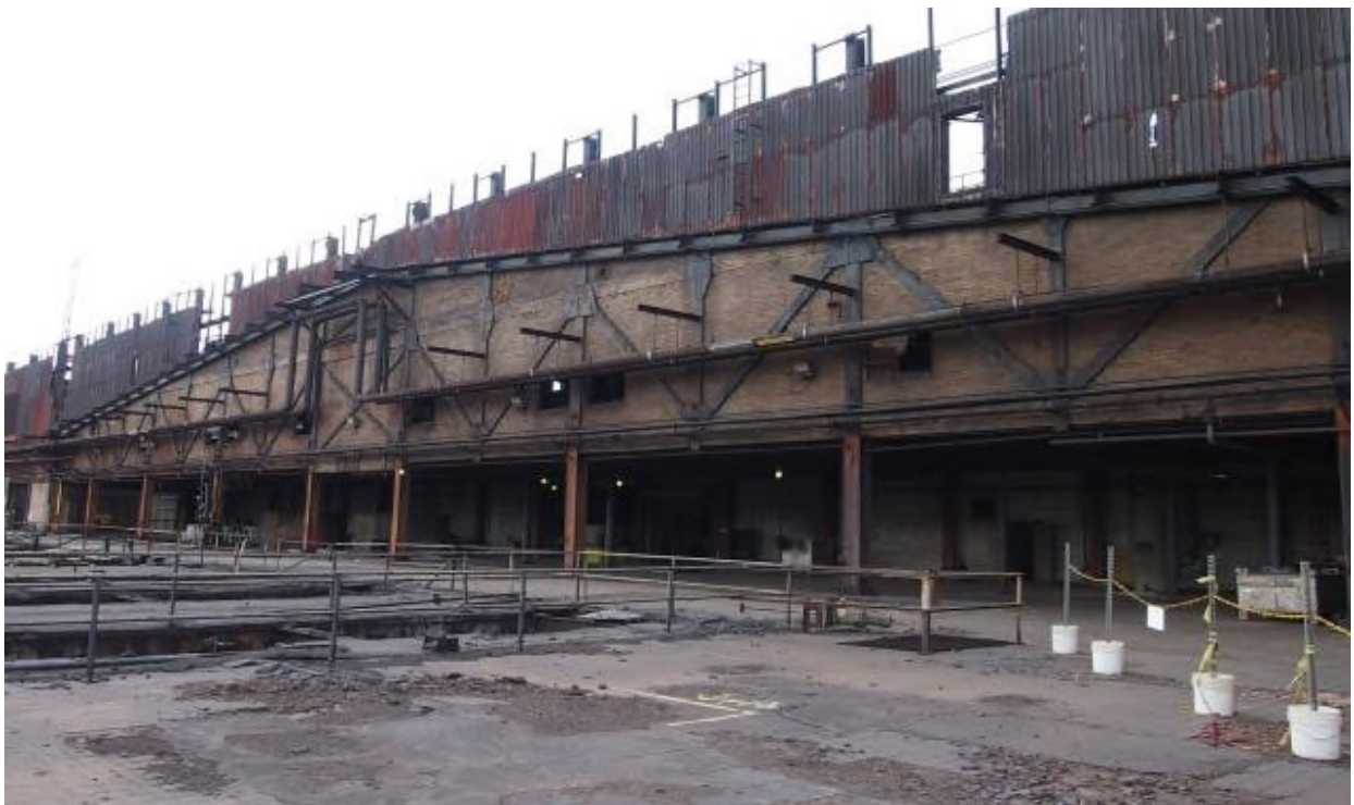
Figure 4: Unit 4 Chlorinator Building wall, looking northwest
