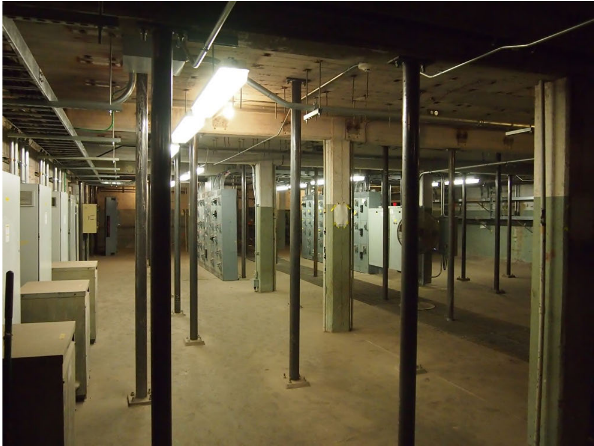
Figure 4: Structure in Basement of Substation Building
