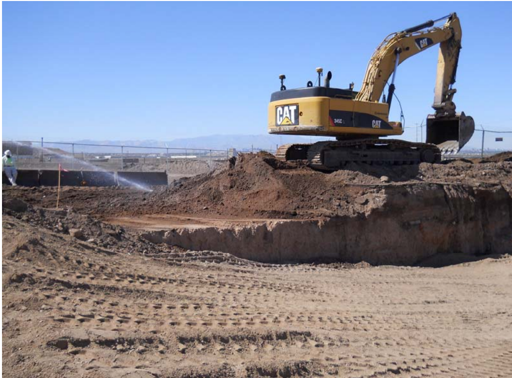
Photo 3: Facing northwest. Excavation progress near end of second day. October 2, 2013.
