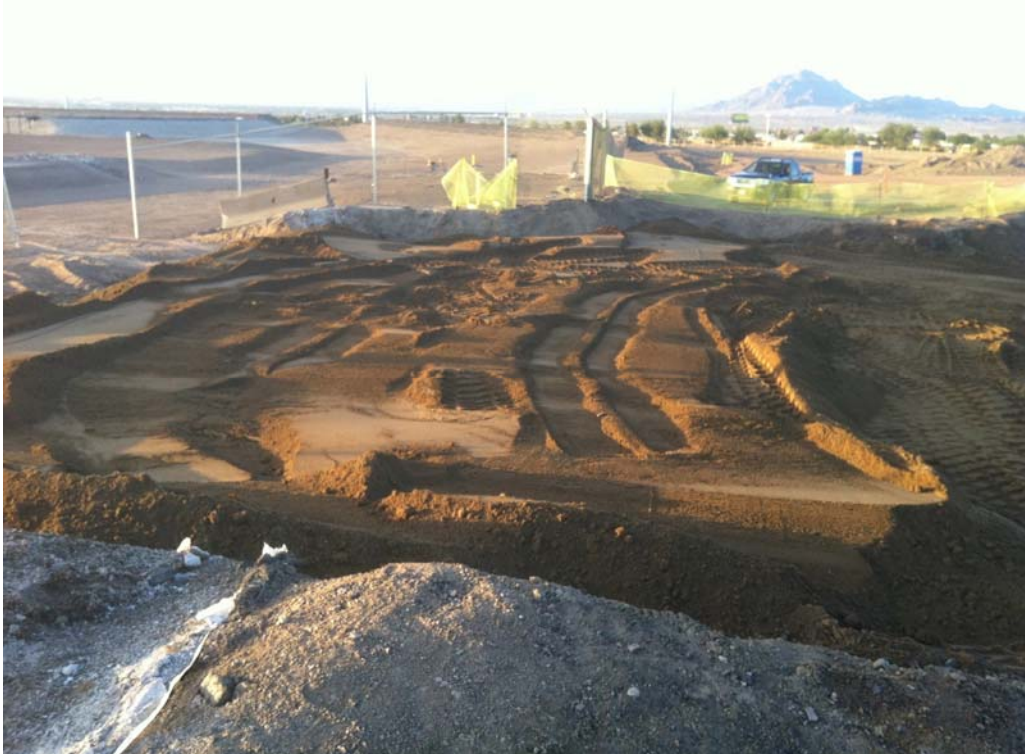
Photo 11: Facing north. Excavation during backfilling and compaction. October 11, 2013.
