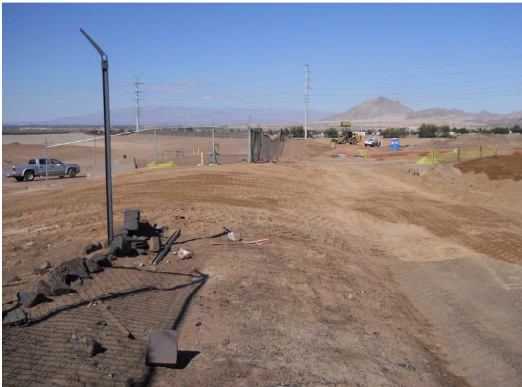
Photo 14: Facing north. Restoration of perimeter roadway after completion of backfilling and compaction. October 14, 2013.
