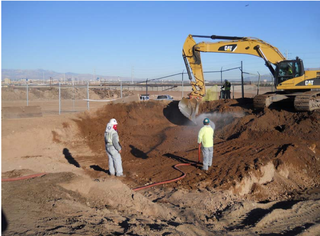
Photo 7: Facing northwest. Excavation nearing completion on fourth day. October 4, 2013.
