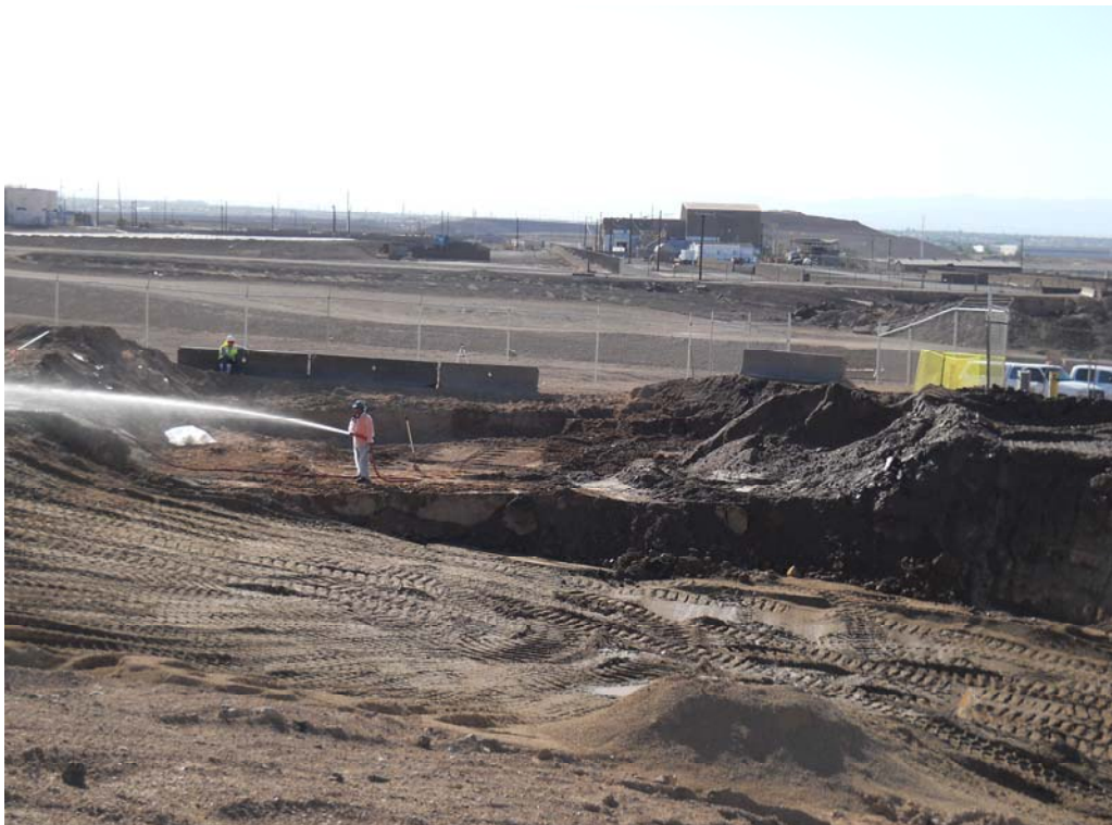
Photo 6: Facing west. Excavation progress toward end of third day. October 3, 2013.
