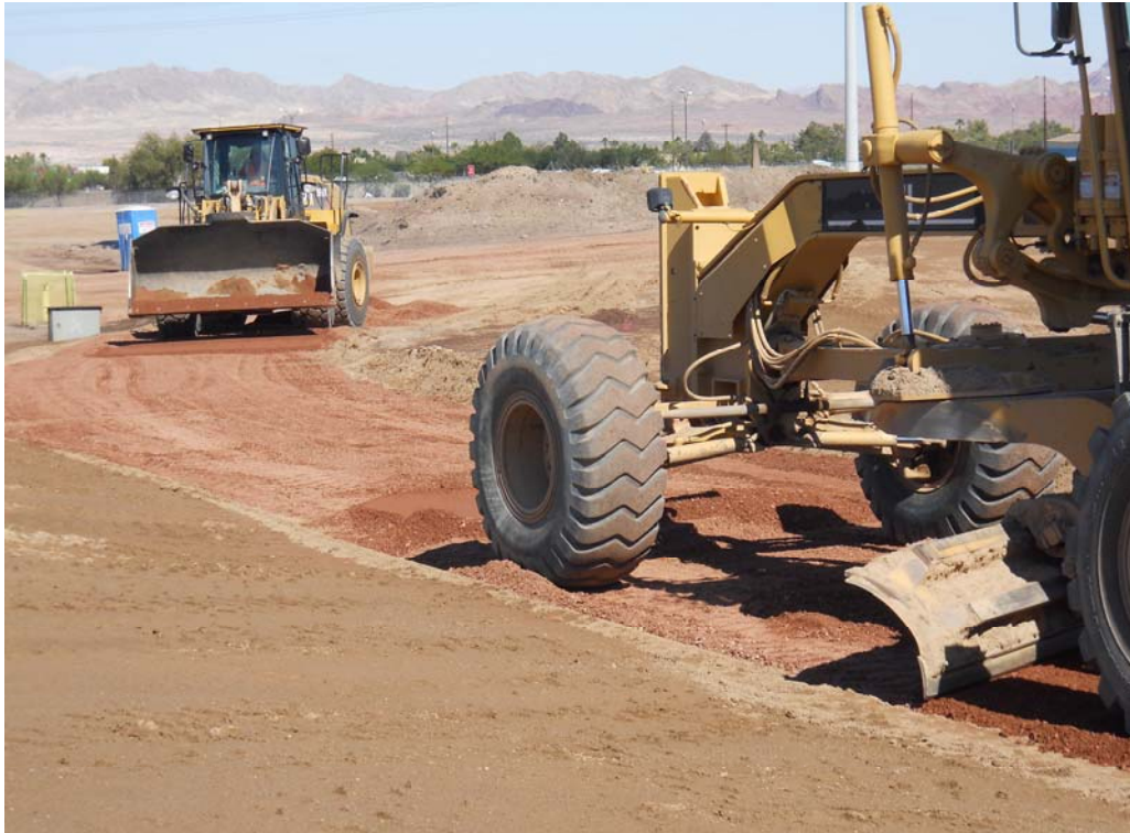
Photo 15: Facing northeast. Resurfacing of perimeter roadway with gravel road base. October 15, 2013.
