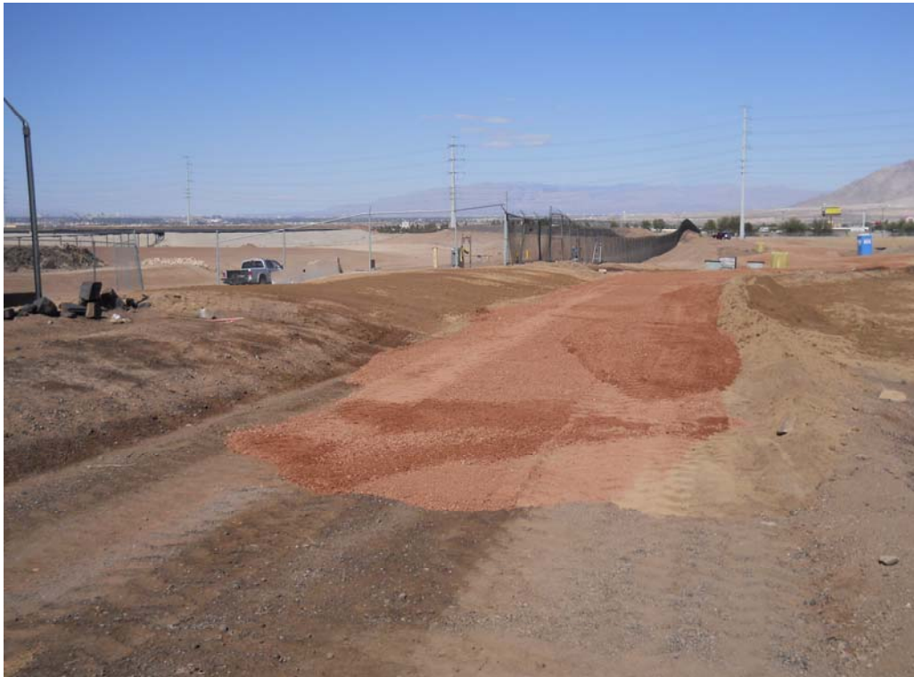
Photo 16: Facing north. Perimeter roadway after resurfacing. October 15, 2013.
