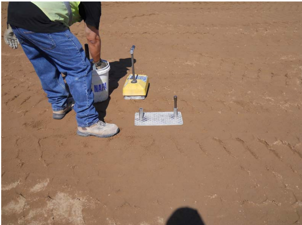
Photo 12: Facing east. Compaction testing of backfill materials. October 11, 2013.
