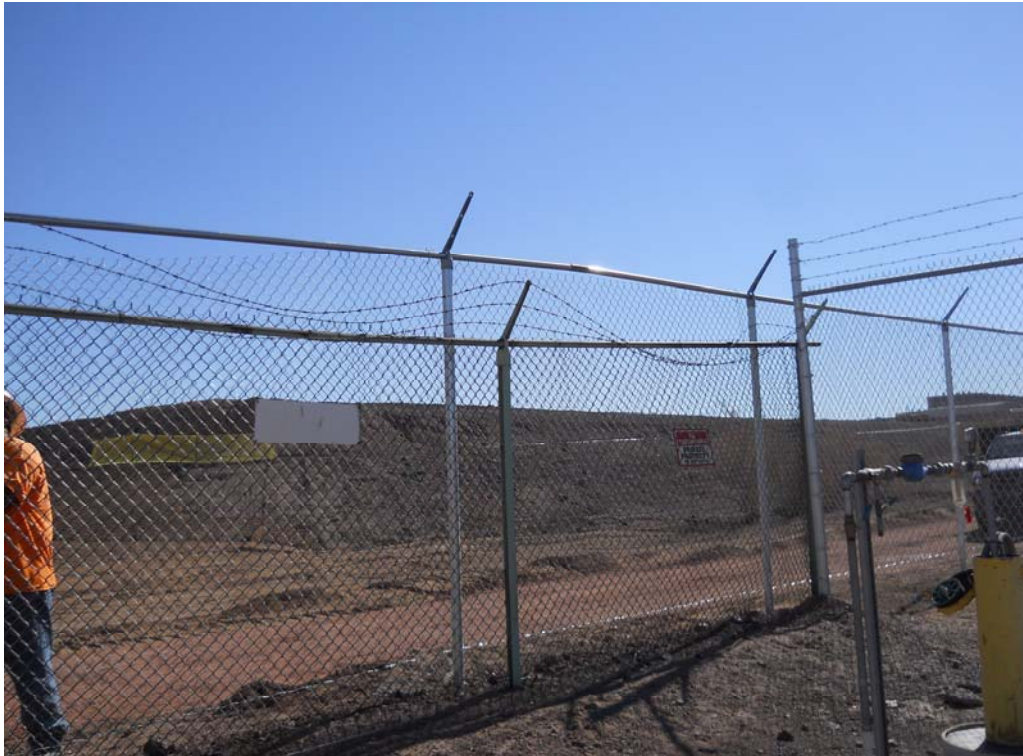
Photo 17: Facing southeast. Installation of new perimeter security fence. October 18, 2013.
