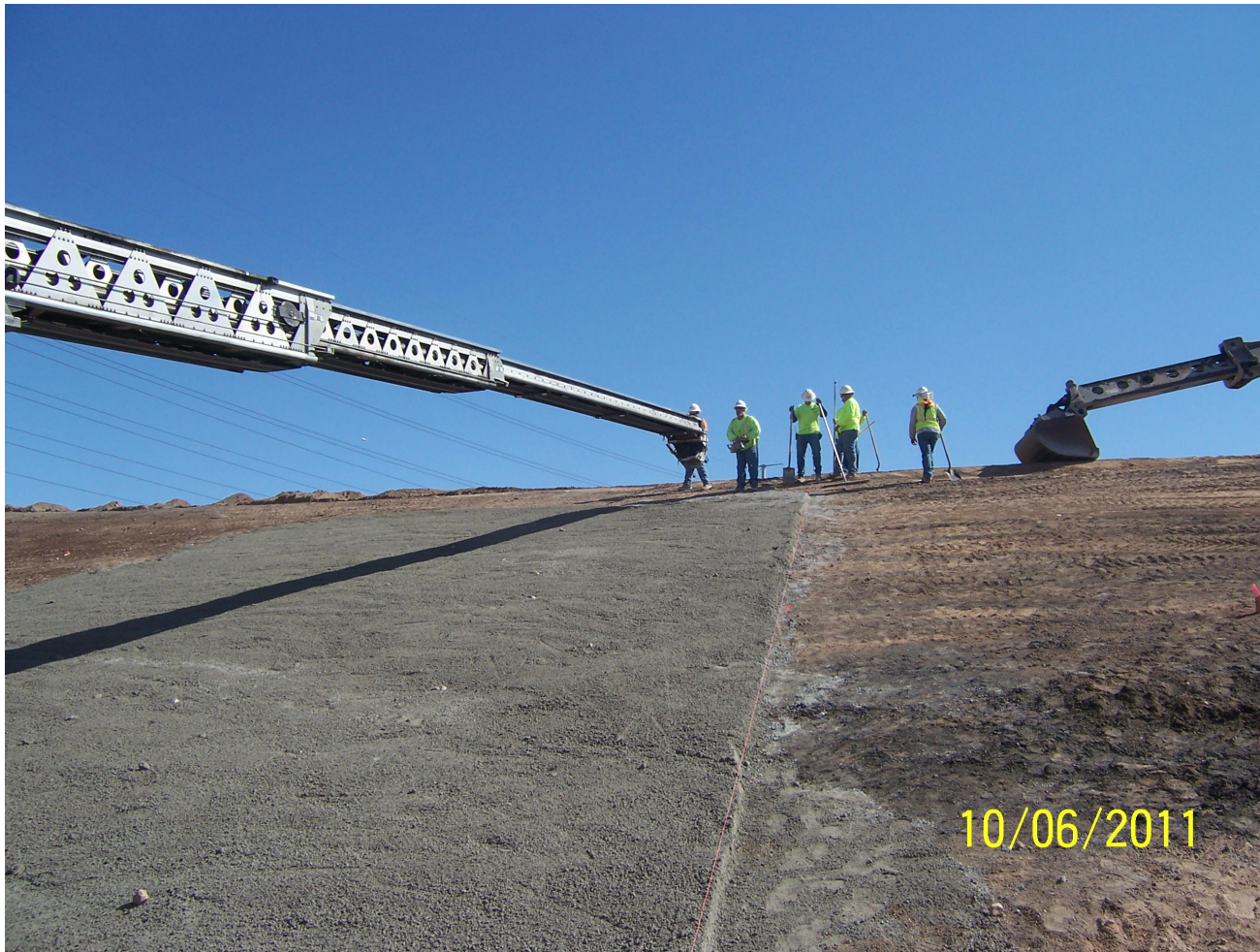
West RZ-D-1 to 7 Placement of Slope Treatment
