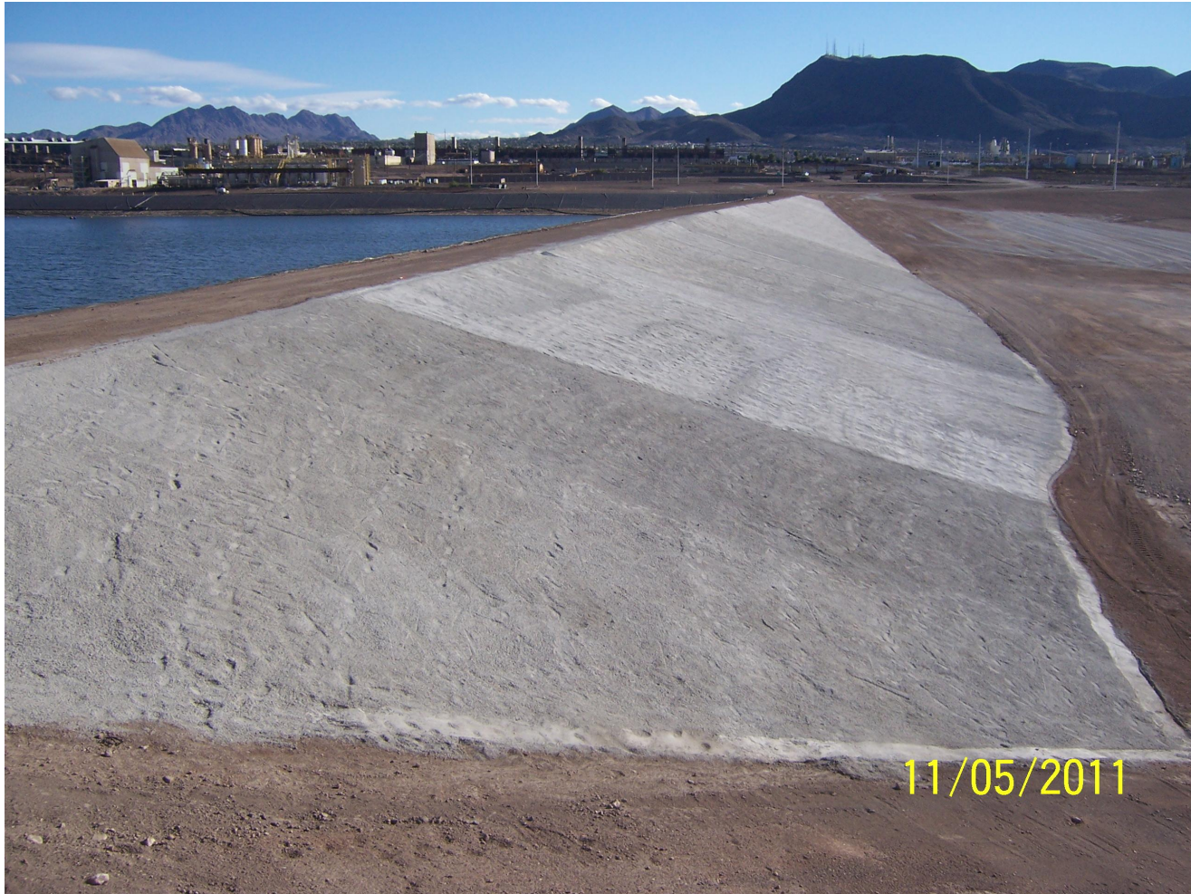
West RZ-D-1 to 7 Slope Treatment Placed
