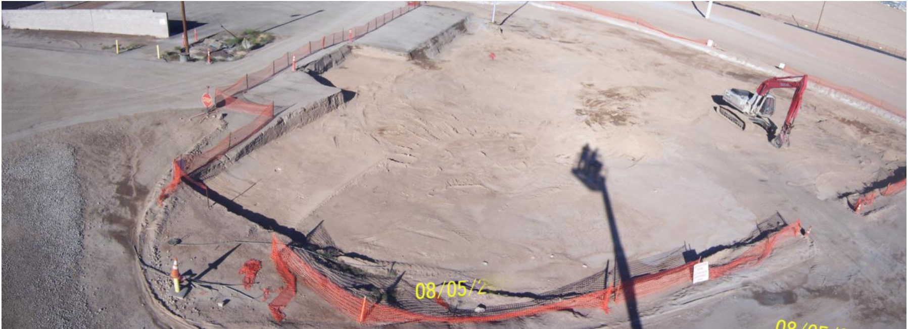
West RZ-D-8 to 14 Visually Impacted Soil Excavation
