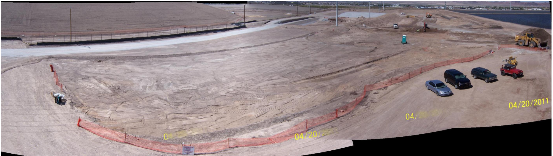
West RZ-D Outside of Polygons Visually Impacted Soil Excavation
