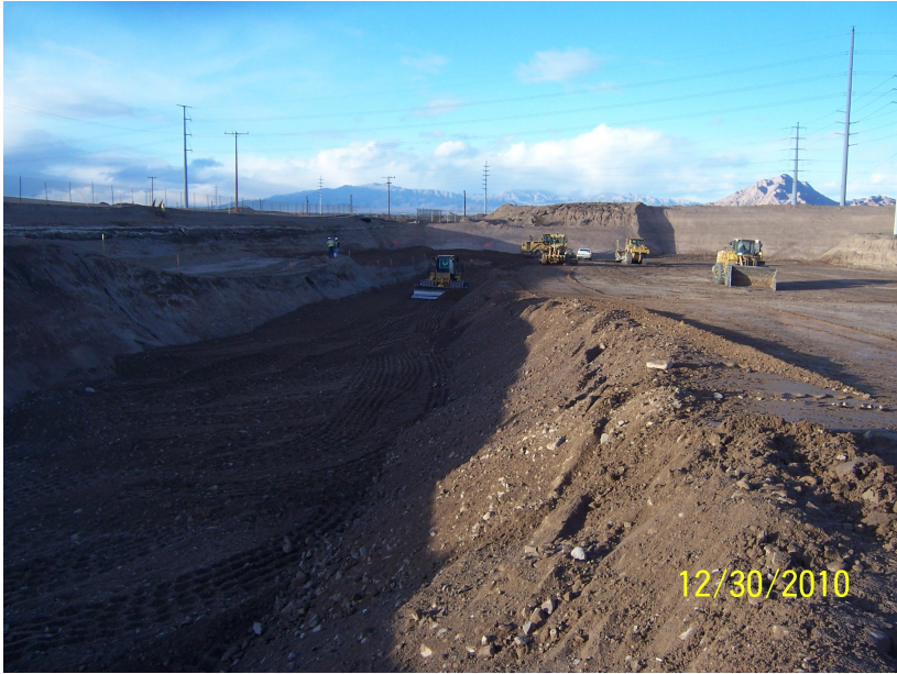
West RZ-D-01A1 Polygon Backfill
