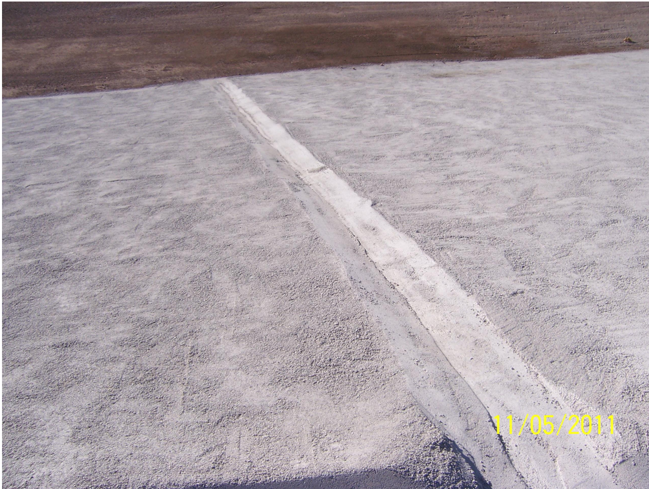
West RZ-D-1 to 7 Typical Down Drain Compacted into Slope Treatment
