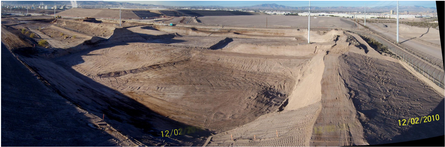
West RZ-D-1 to 7 Polygon Excavation
