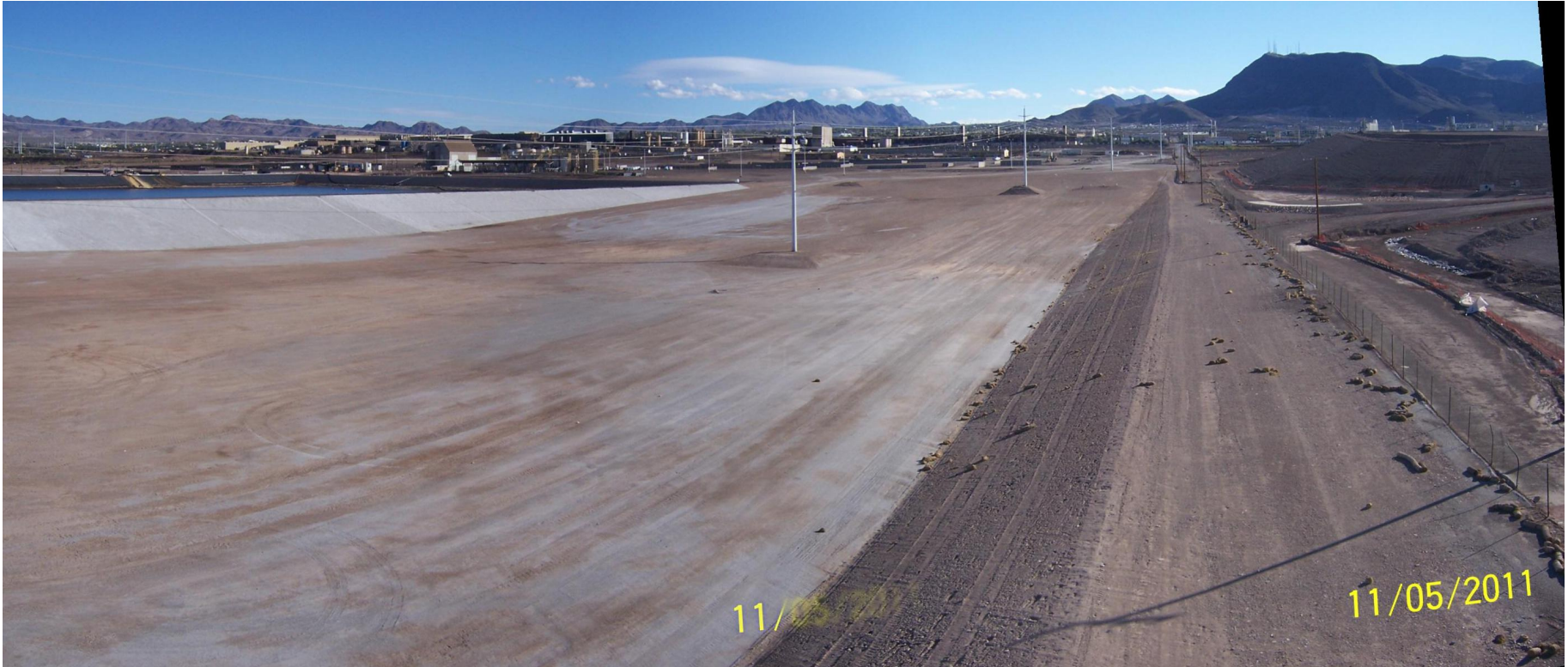
West RZ-D-1 to 7 Finished Grading and Slope Treatment
