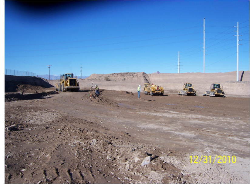
West RZ-D-01A1 Polygon Backfill
