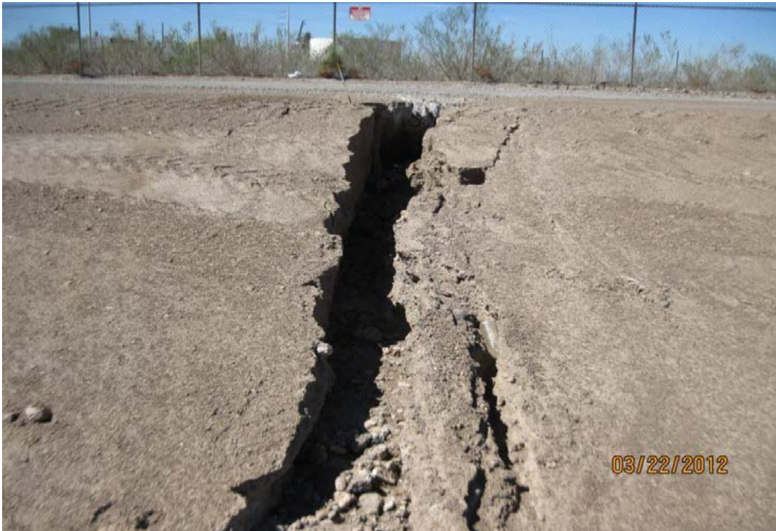
Photo 5: Looking west at a wash out off of 5th Street.
