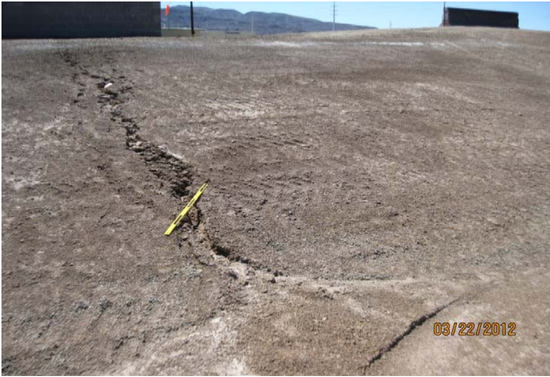
Photo 1: Looking south-southwest rill in southern slope of Beta Ditch just east of 5th Street.
