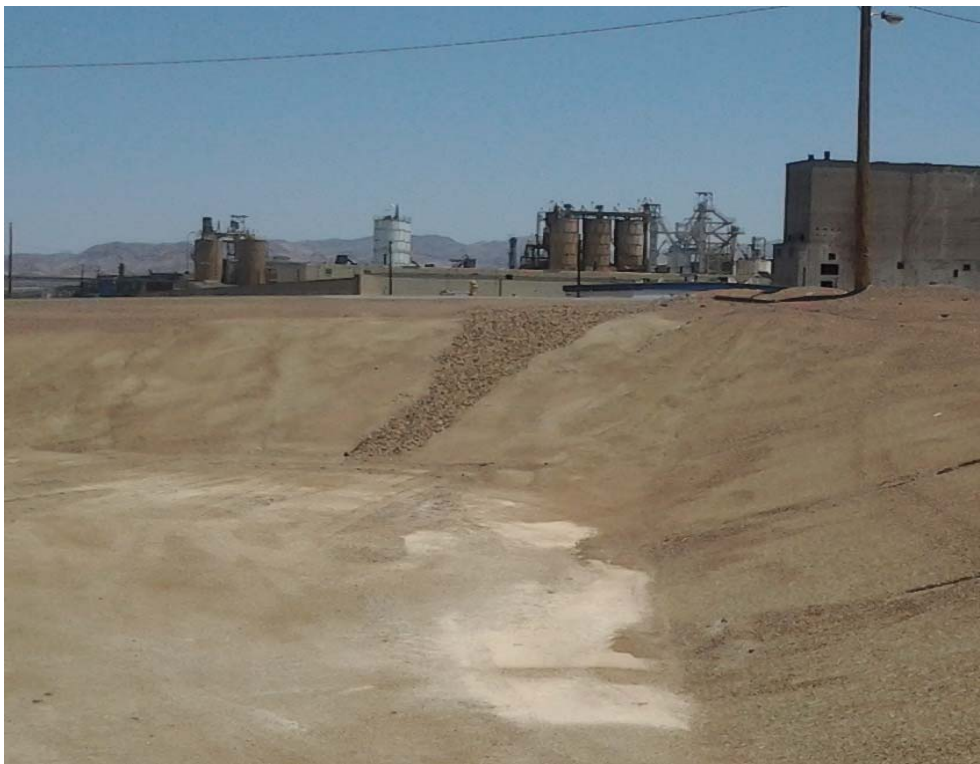
Photo 2: Typical Energy Dissipating Channel
