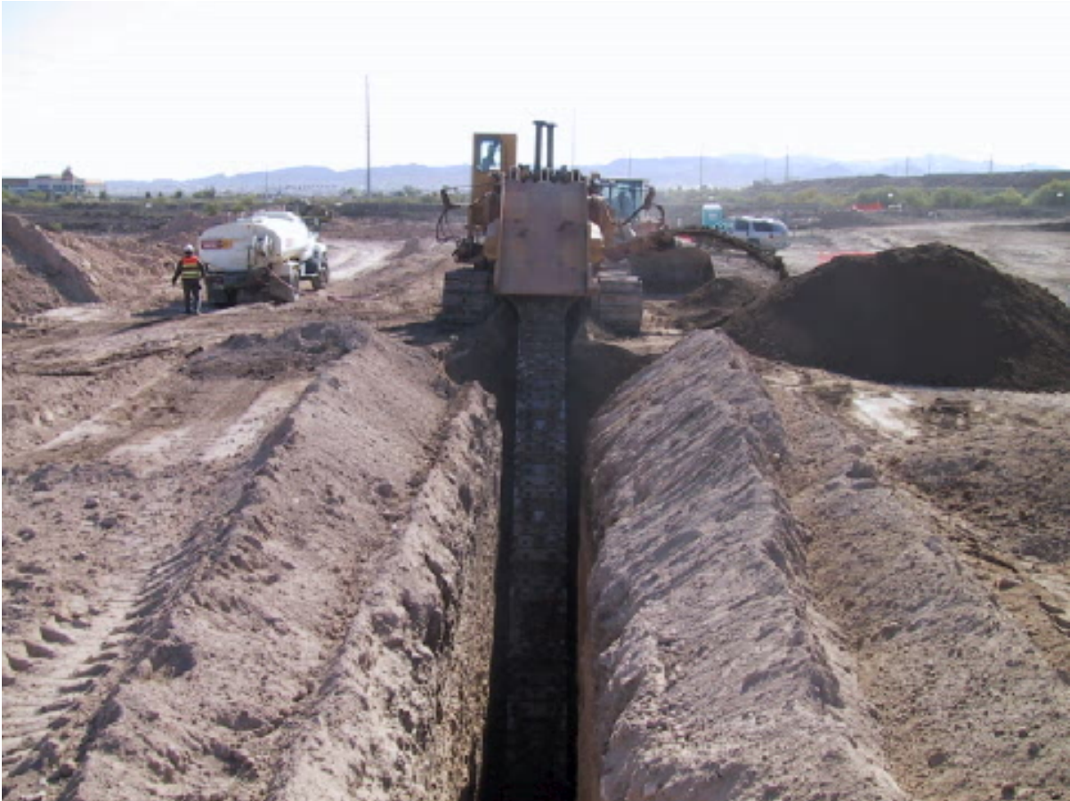
Figure 7-2: Typical Trench Excavation
