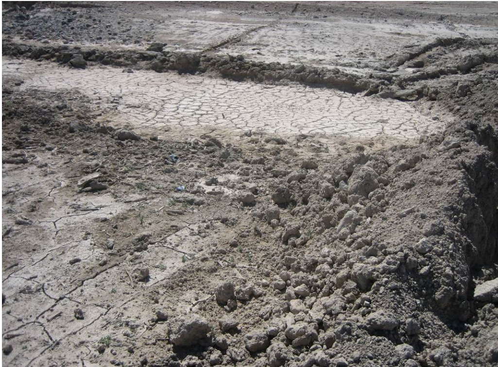
Photo 5: Excavated areas near former BMI ponds.
