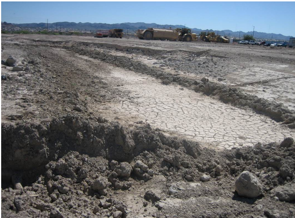
Photo 4: Excavated areas near former BMI ponds.
