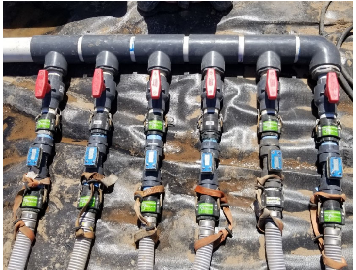
Right: Four bag filters are used to filter sediment from the extracted groundwater prior to the groundwater being pumped to the frac tanks/injection system in the laydown area. Left: Extraction manifold with flow meter for each extraction well.
