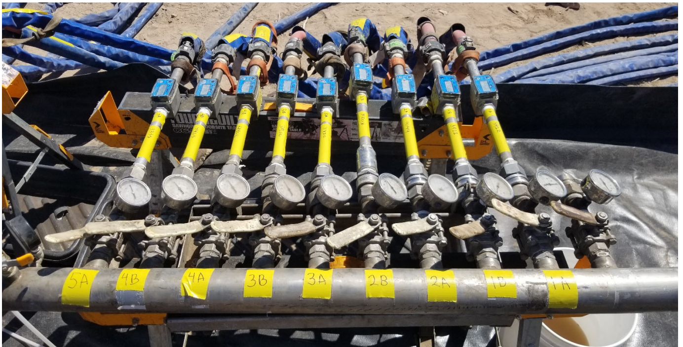
Injection manifold with flow meters and pressure gauges for each injection well.
