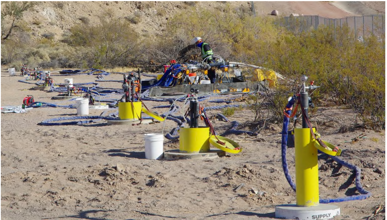
Fully connected Injection well transect line within Zone 3 – UMCf-cg.
