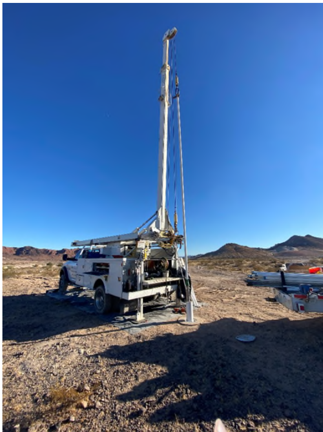
During mobilization activities, high-capacity pumps were installed in six extraction wells (left). Extraction wellhead with sampling port, electrical box, pressure gauge, and 3/4-inch PVC pipe for depth to water monitoring (right).
