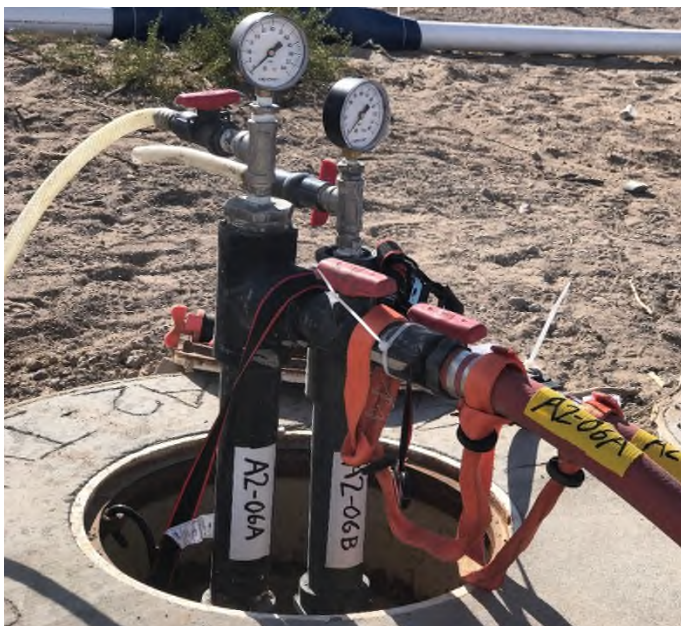
Injection Wellheads
