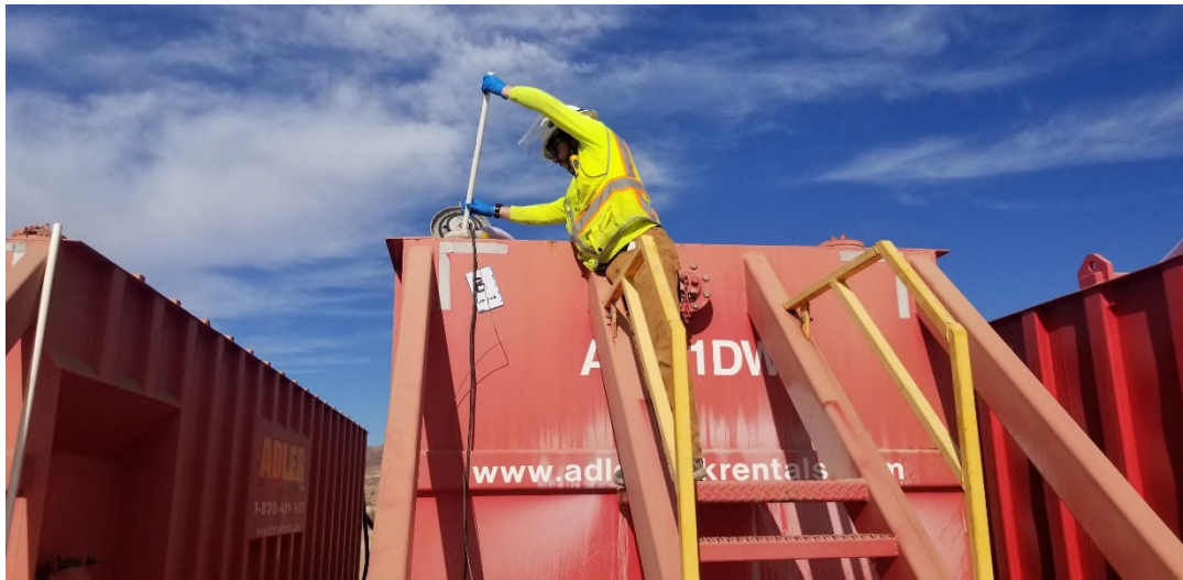
Collecting a sample of carbon substrate solution to prior to injection.
