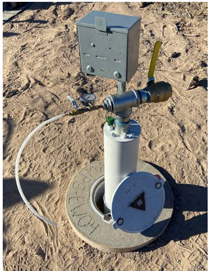
During mobilization activities, high-capacity pumps were installed in six extraction wells (left). Extraction wellhead with sampling port, electrical box, pressure gauge, and 3/4-inch PVC pipe for depth to water monitoring (right).
