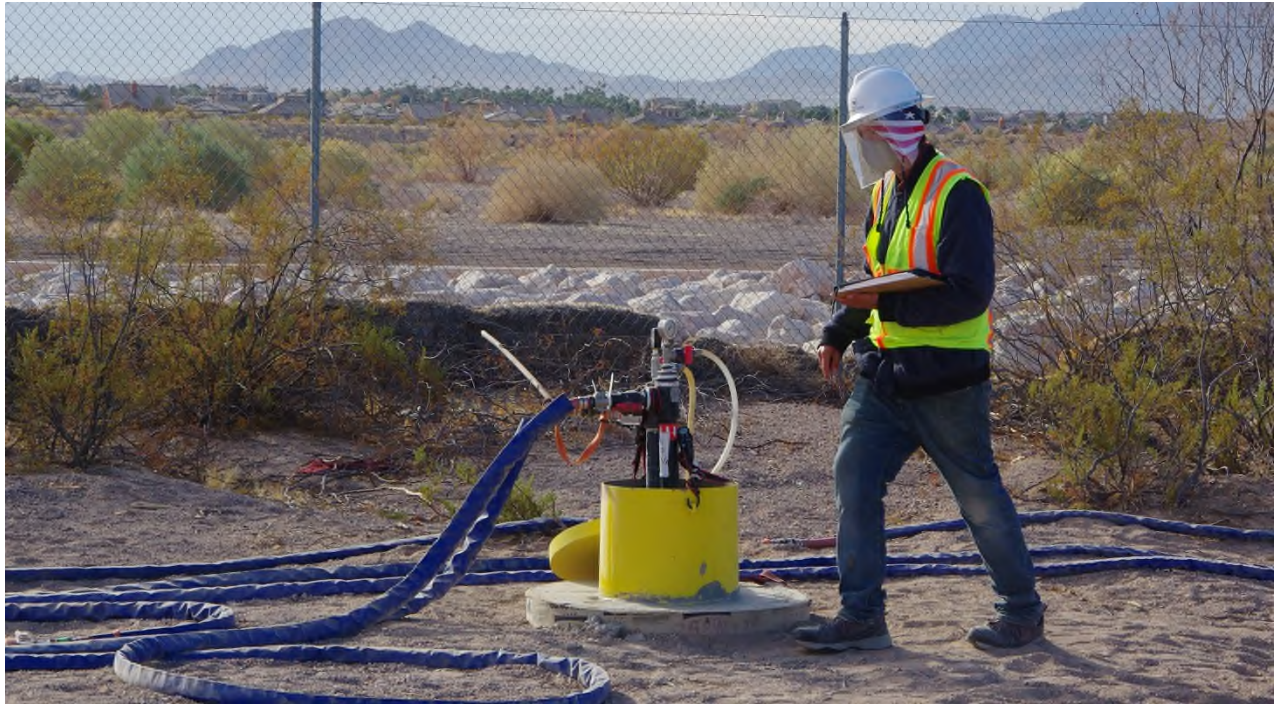
Walking the injection line within Zone 3 to record pressure readings at individual injection wellheads.
