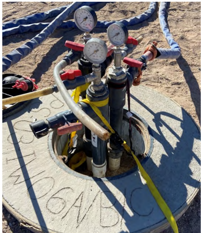
Walking the injection line within Zone 3 to record pressure readings at individual injection wellheads.
