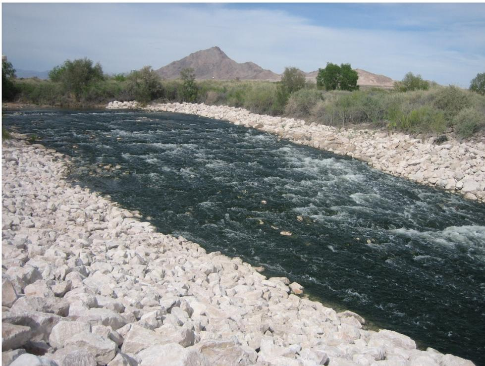
Photo 19: Illustration of bank stabilization at the temporary diversion channels used during weir condition.
