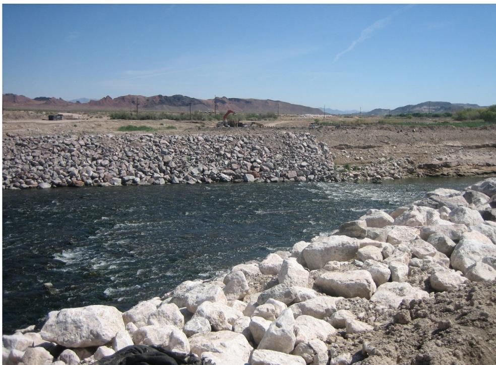
Photo 20: Illustration of bank stabilization at the temporary diversion channels used during weir condition.
