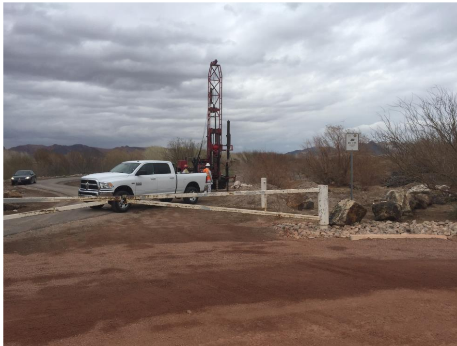
Photo 2. Borehole B-5, View looking east along water conveyance pipeline alignment.
