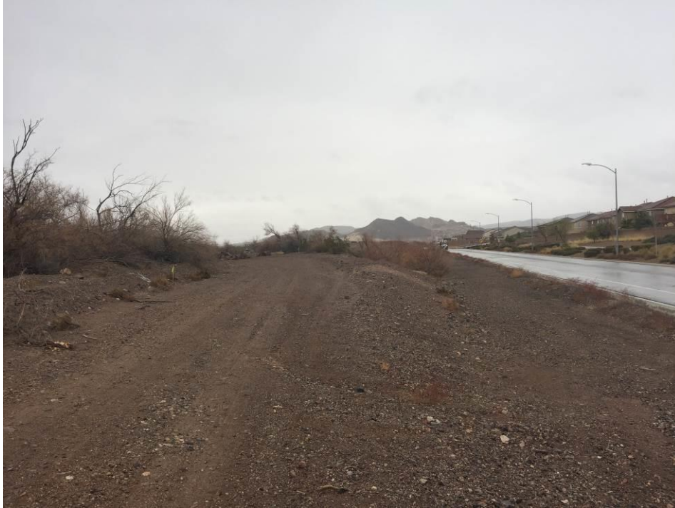
Photo 5, View looking east along water conveyance pipeline alignment north of Russell Road.
