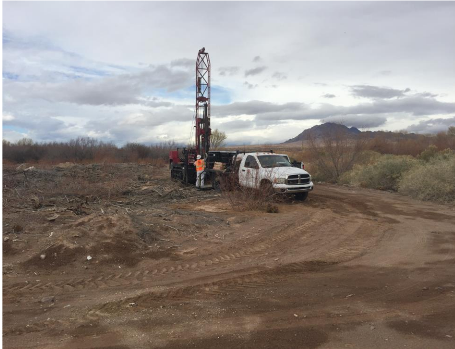
Photo 3. Borehole B-3, View looking north along pipeline alignment.
