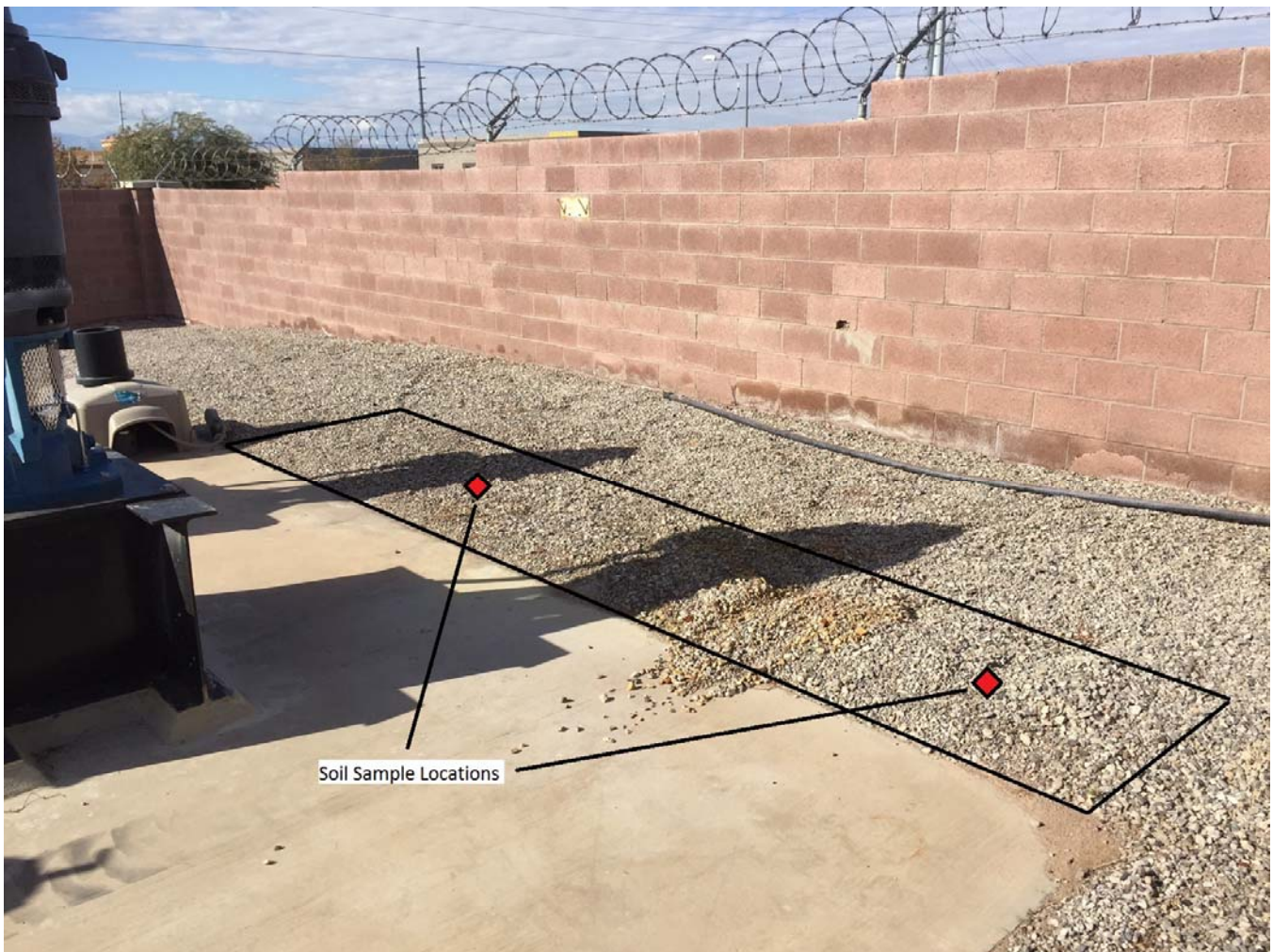
Photograph 1 Extent of Excavation with Lift Station 2
