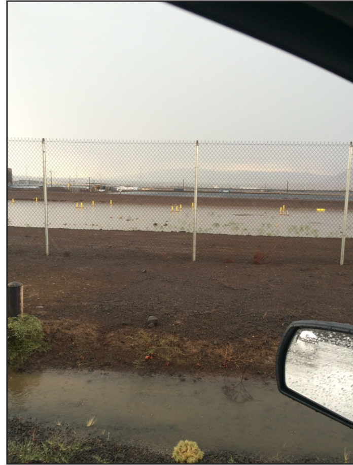
Central Retention Basin, view facing north. Photo taken at 4:31 PM, August 13, 2015.
