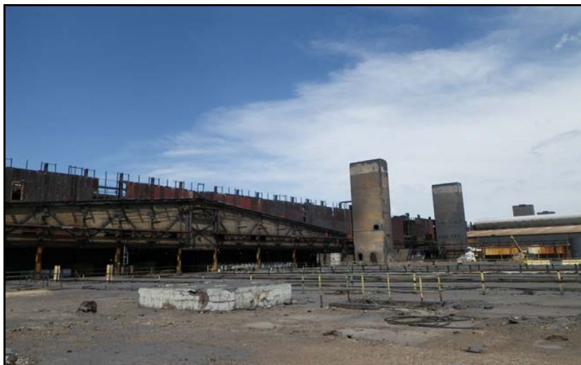
Unit 4 cell building floor, Unit 4 chlorinator building in background (View looking northeast)
