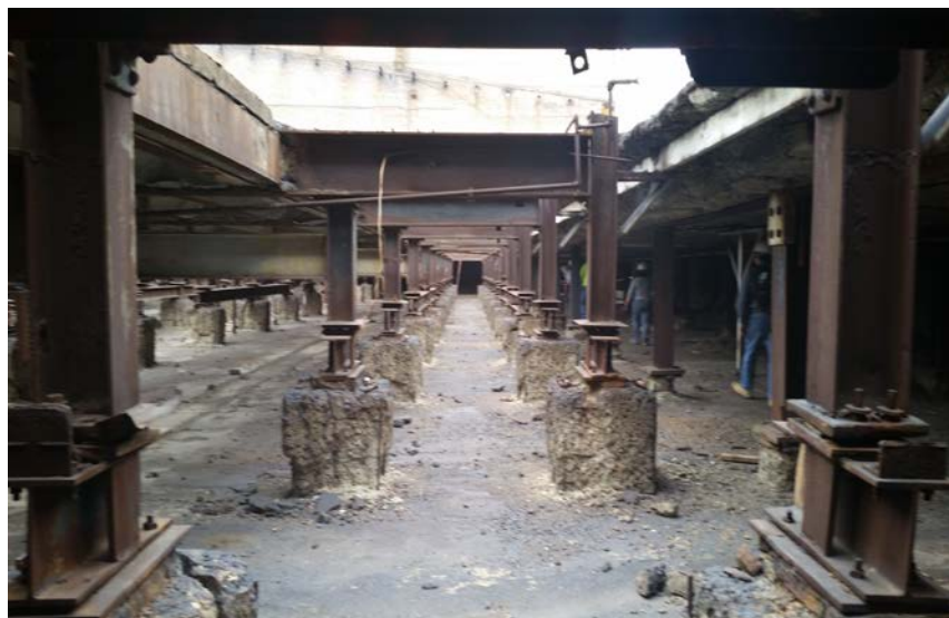
Unit 4 cell building basement floor
