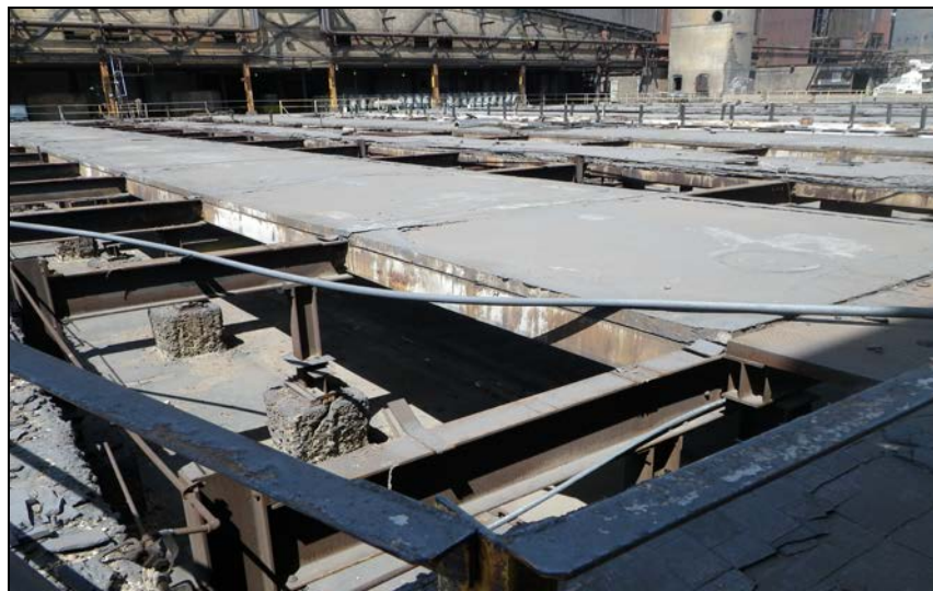
Unit 4 cell building floor (View looking north)
