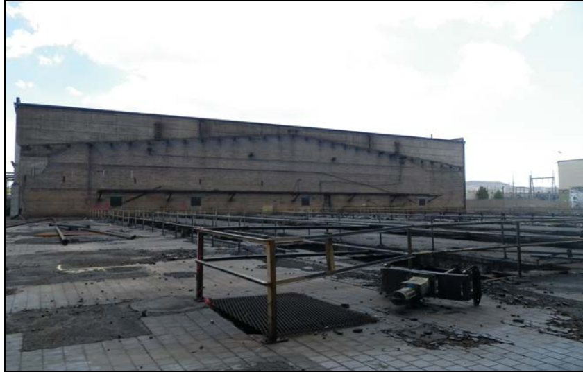
Unit 4 cell building floor with Unit 4 substation building in background (View looking southwest)
