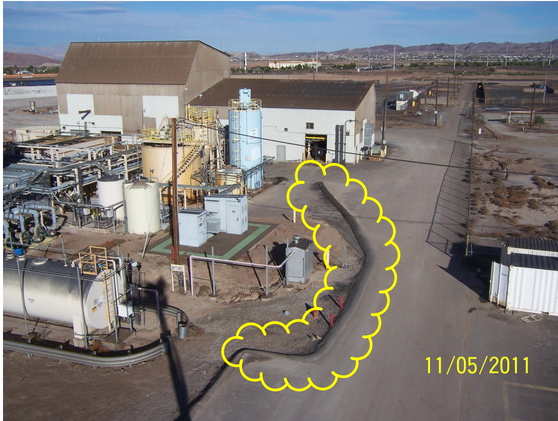
East RZ-D-Veolia Water Storm Water Diversion Berm
