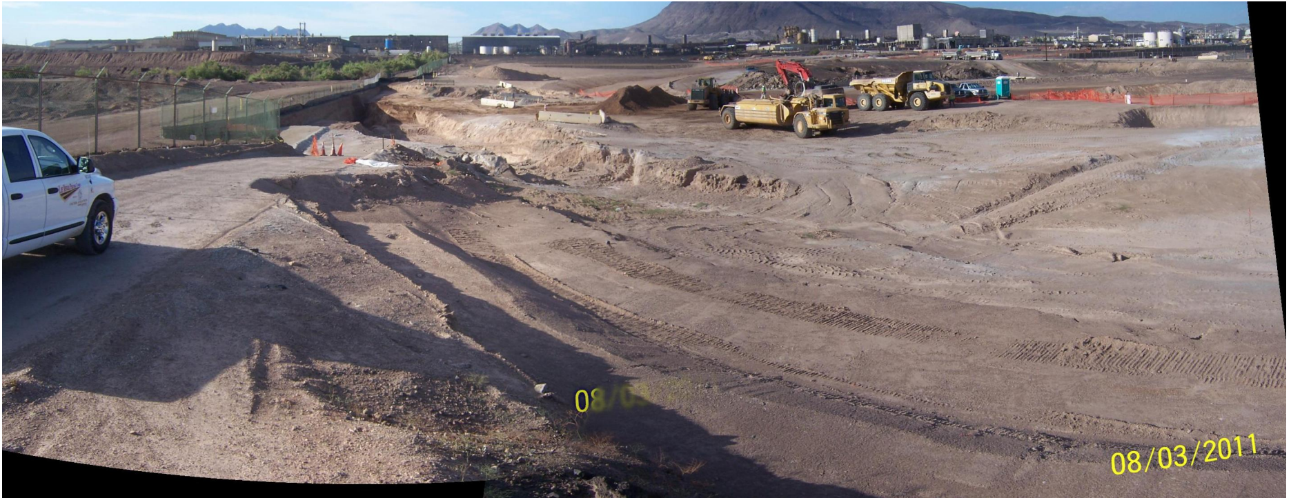
East RZ-D-24 to 25A Visually Impacted Soil Excavation
