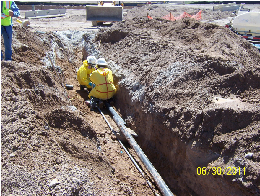
East RZ-D-24 to 25A Lowering of the Extraction Well Line to allow for the New Channel to Travers the Area
