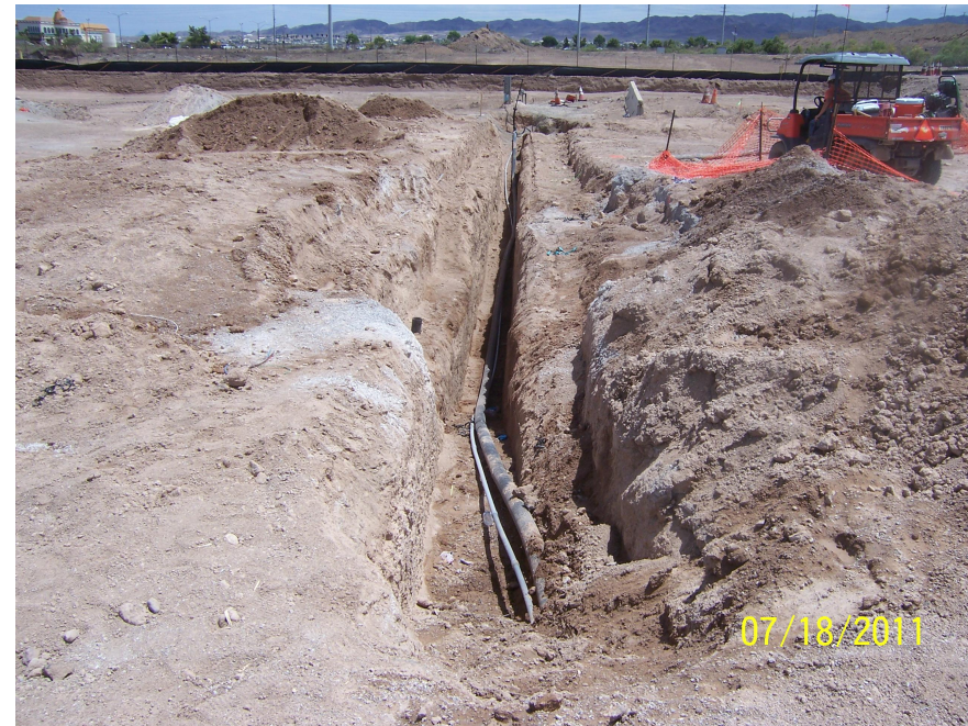
East RZ-D-24 to 25A Lowering of the Extraction Well Line to allow for the New Channel to Travers the Area
