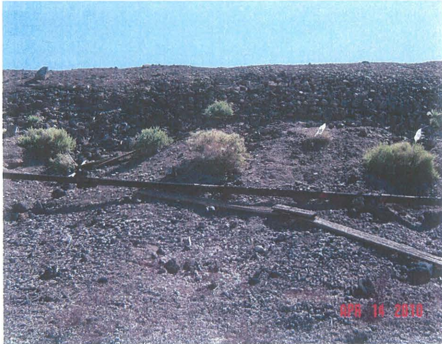
Photo 11 – West debris pile with pipe on side of hill. Pipe contains asbestos pipe wrap.
