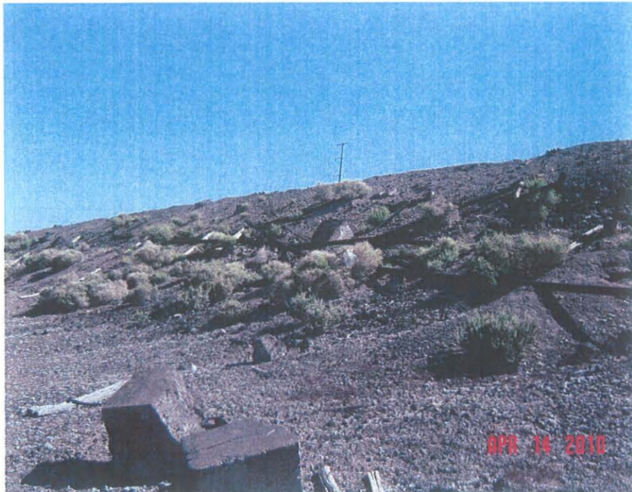
Photo 13 – West debris pile with pipe on side of hill. Pipe contains asbestos pipe wrap.
