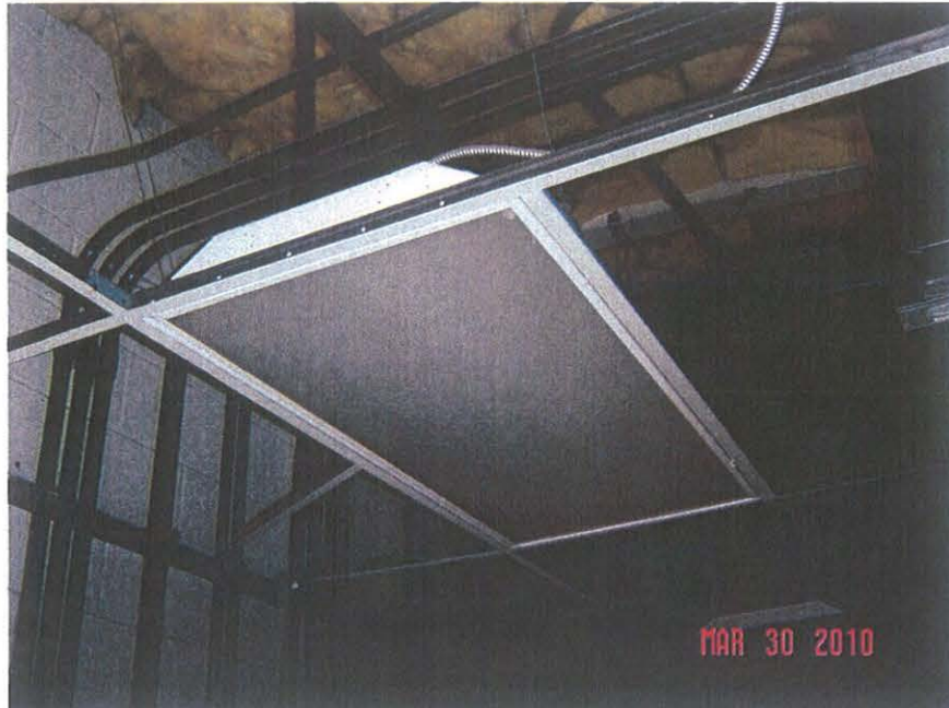
Photo 1 – Light fixtures with fluorescent lights.
