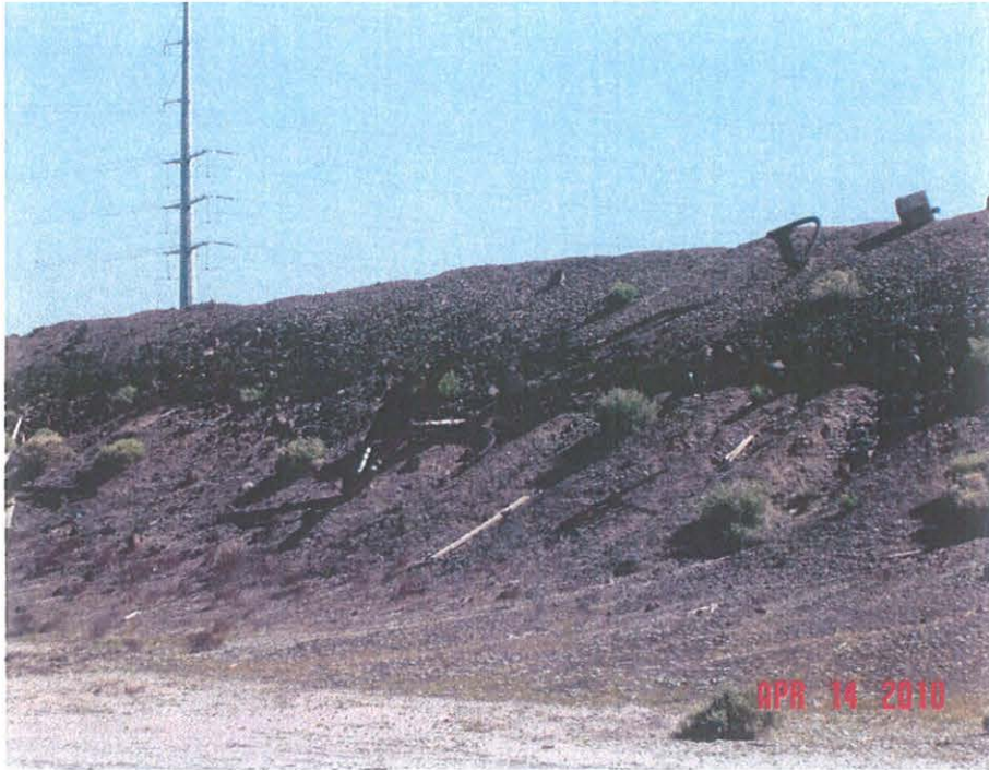
Photo 7 – West debris pile with pipe on side of hill. Pipe contains asbestos pipe wrap.
