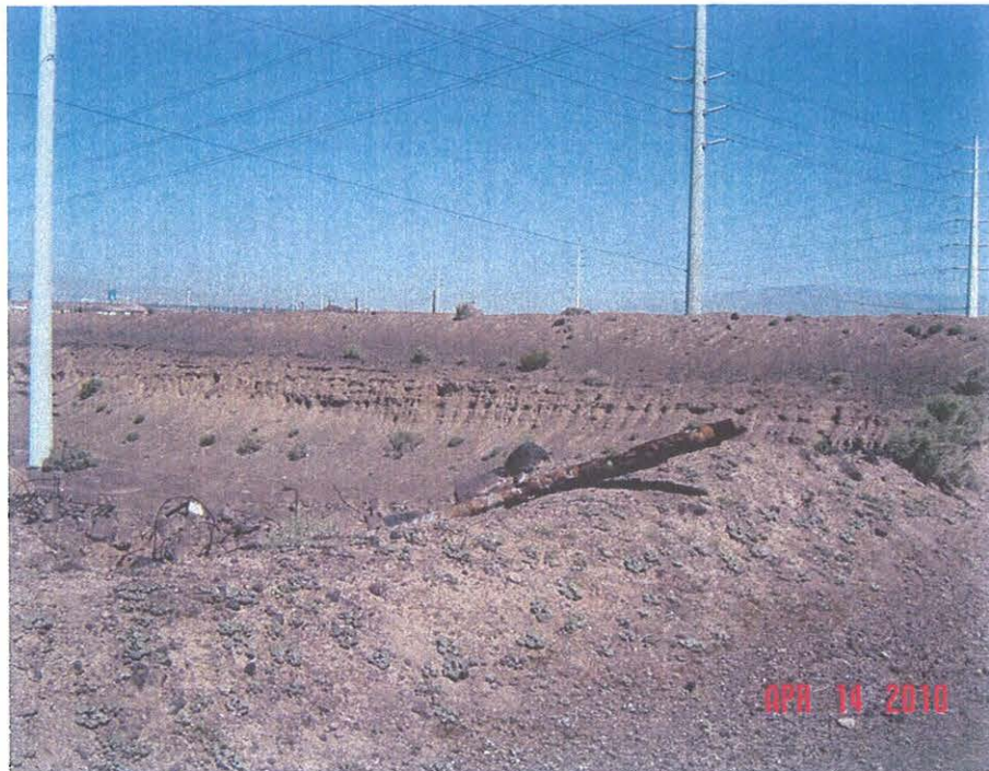
Photo 15 – West debris pile with pipe on side of hill protruding over hill. Pipe contains asbestos pipe wrap.
