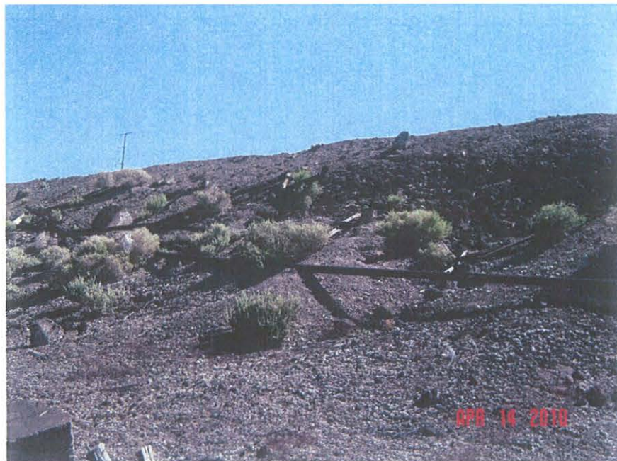
Photo 12 – West debris pile with pipe on side of hill. Pipe contains asbestos pipe wrap.
