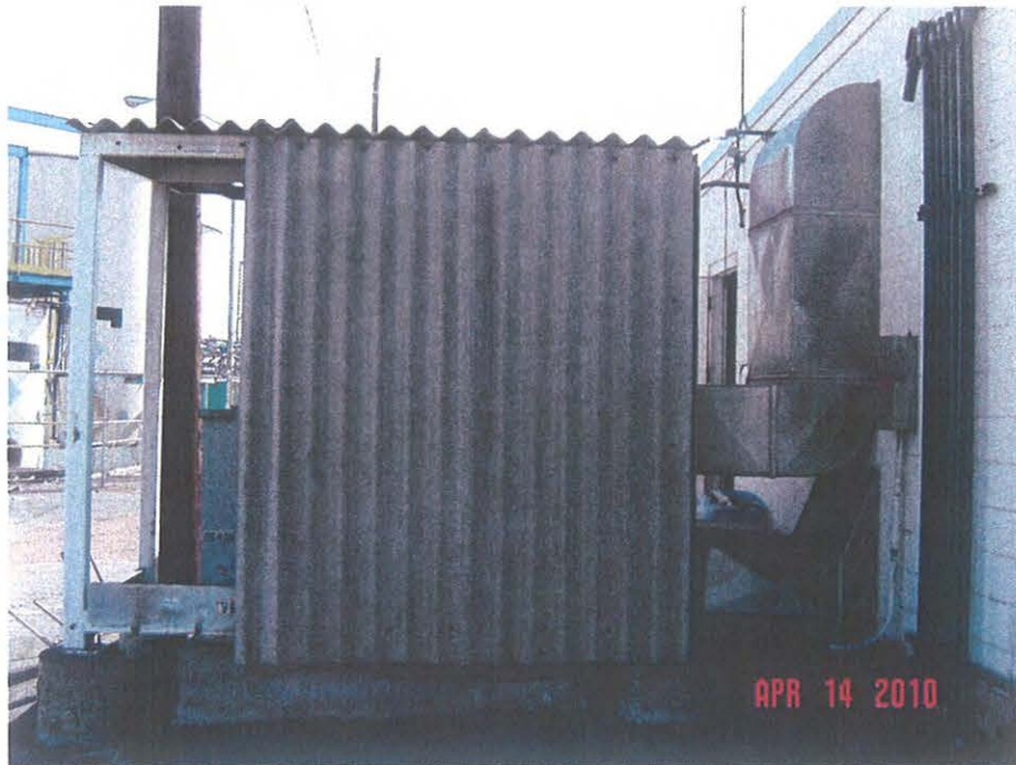
Photo 5 – These panels are non-Asbestos.
