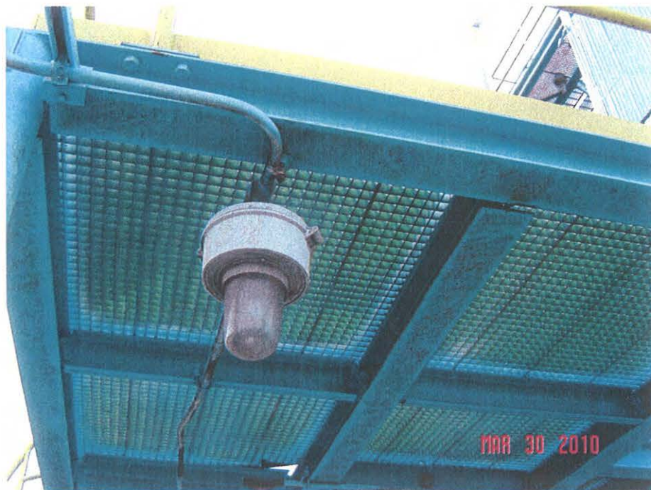
Photo 5 – Mercury containing light, these lights can be found throughout the AP area.
