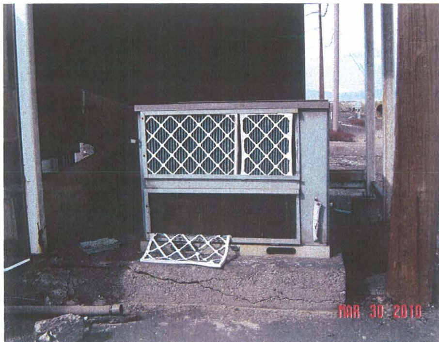
Photo 2 – AC unit in back of block building near west pipe bridge.
