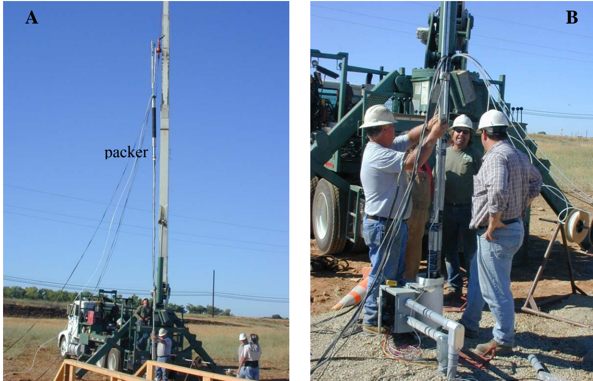
Figure 2.2. Photograph of Equipment Installation into the Downflow HFTW at Aerojet. The packer is visible in panel A and the wiring, tubing, and equipment present in the HFTW is seen in Panel B.
