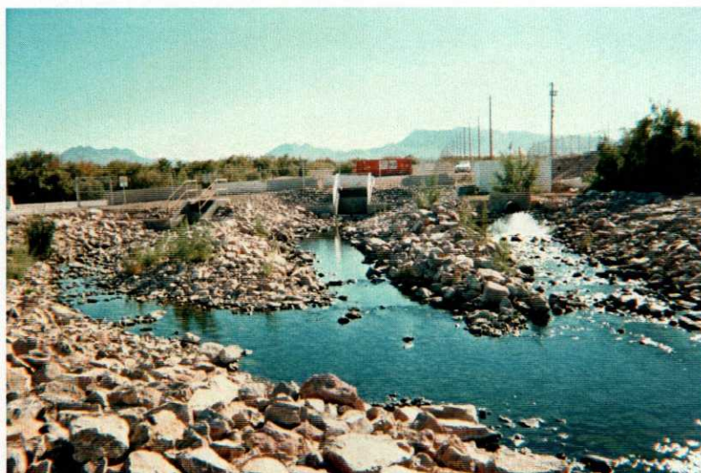
Figure 5: Henderson discharge channel showing the three main discharge streams upstream of the Kerr-McGee discharge water inflow point; the primary and secondary Henderson wastewater discharges (left and middle) and the BMI discharge (right).
