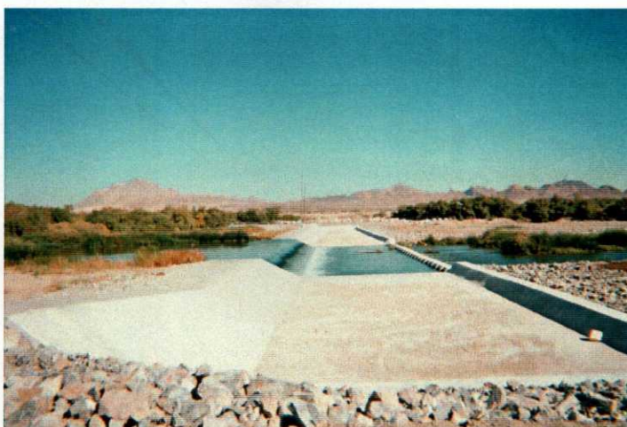
Figure 3: Las Vegas Wash at the Pabco Road erosion control structure.
