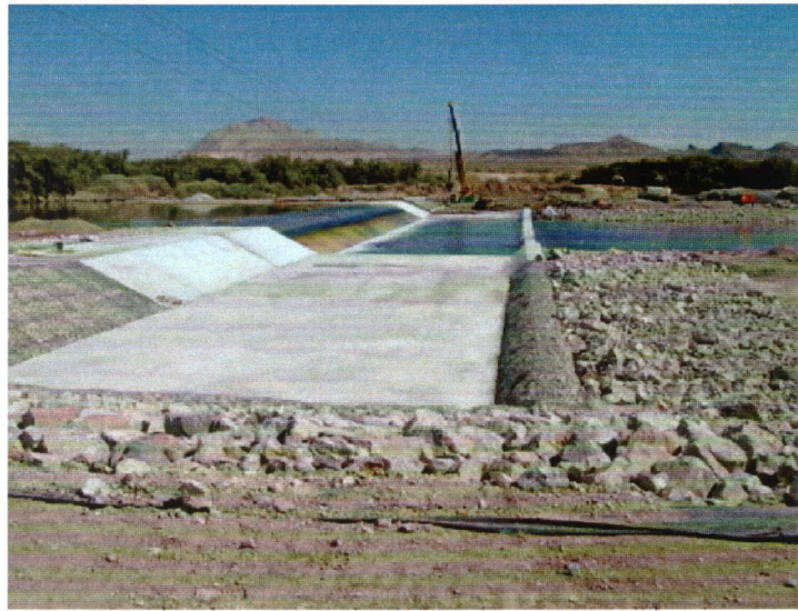
Figure 5 – Photograph of Pabco Road erosion control structure downstream of Kerr-McGee discharge.
