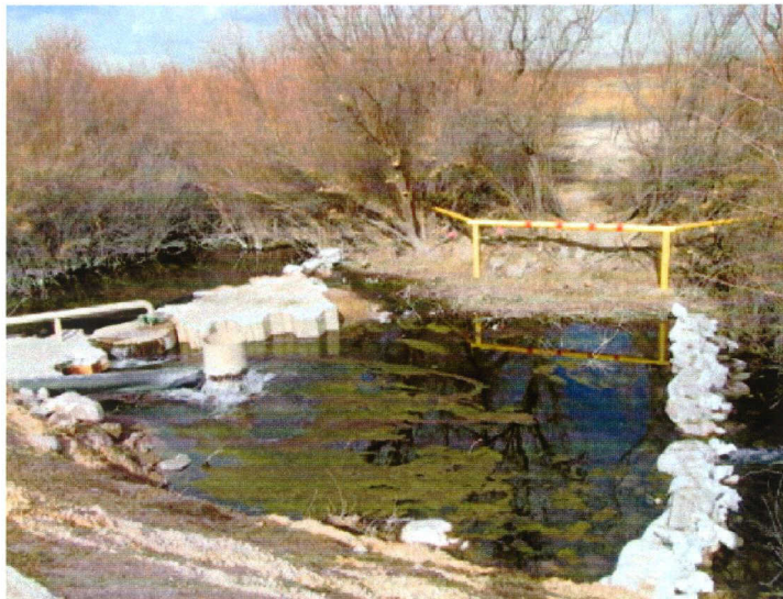
Figure 6 – Photograph showing Kerr-McGee discharge into a pool and discharge from that pool through a low point in a dam.
