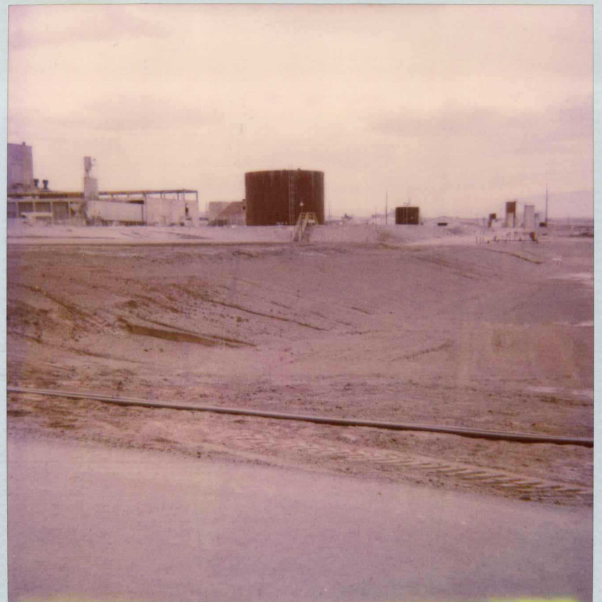
KERR MCGEE 9/89 CLOSED SURFACE IMPOUNDMENTS looking west
