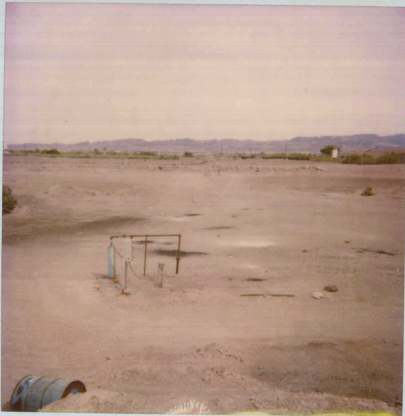
KERR MCGEE 9/89 GW INTERCEPT SYSTEM looking east
