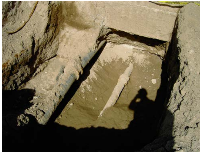
Fig. 1 – Supply Pipeline Excavation and Repair
