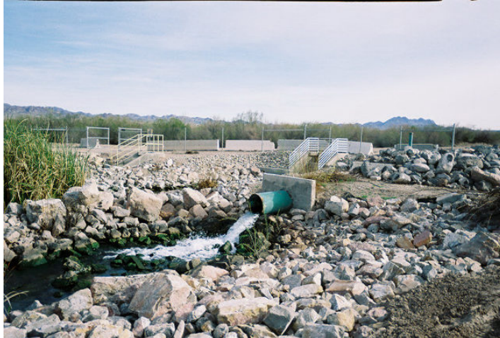
Fig. 7 – Pittman Bypass Pipeline (Las Vegas Wash)
