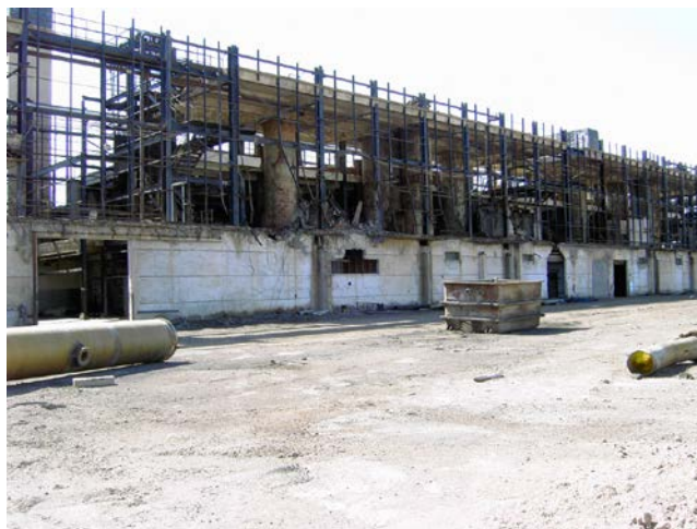
Fig. 2 – Decommissioned Process Unit
