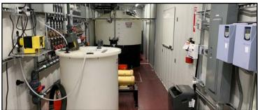
Injection and Extraction System Equipment for a NERT Treatability Study
