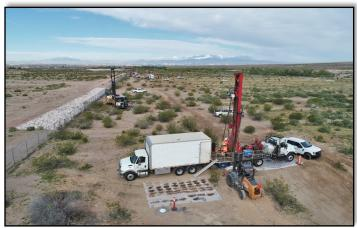
Installation of monitoring wells near the Las Vegas Wash, April 2020
