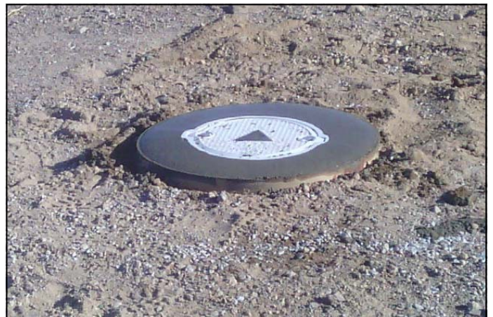
Typical Monitoring Well Surface Completion
