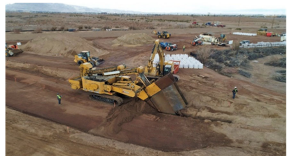
Zero Valent Iron Installation for a NERT Treatability Study
